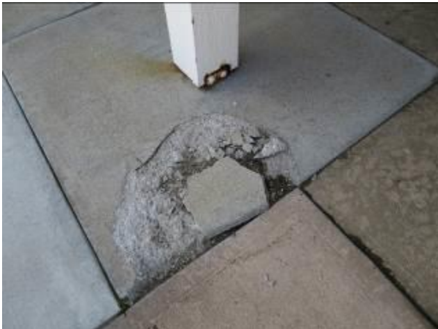
Deteriorated Sidewalk Retail Strip Building (S)
