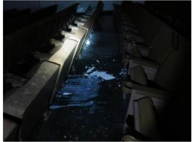
Ceiling Damage In Former Theater
