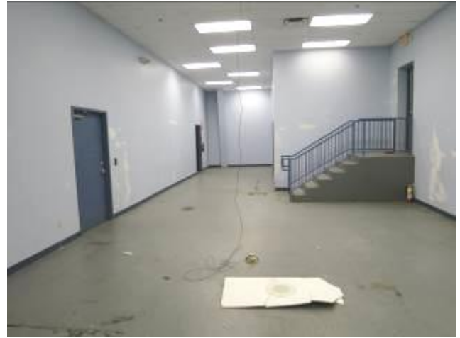
Varied Floor Levels In Vacant Building
