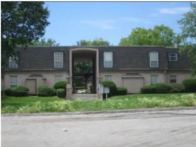
Close (Unshielded) Proximity Of Adjoining Apartment Units To The Unsightly Rear Of Grocer
