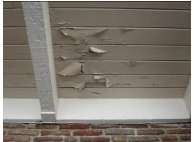
Deteriorating Canopy
