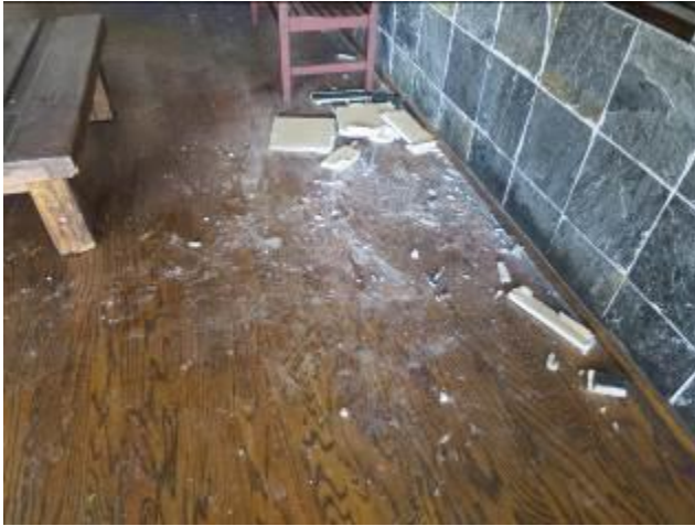
Ceiling Damage In Small Shops
