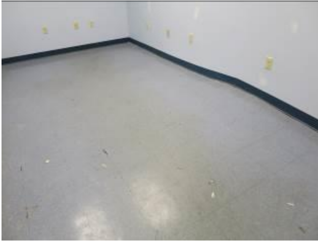
Curving Floor In Office In Vacant Building
