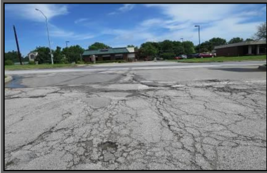
PHOTOGRAPH NO. 10: THE NW ENTRANCE FROM RED BRIDGE ROAD
