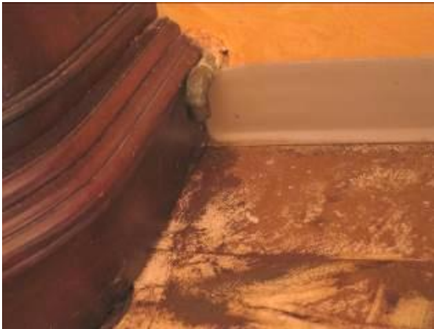
Open Pipe Draining Into Small Shop Space
