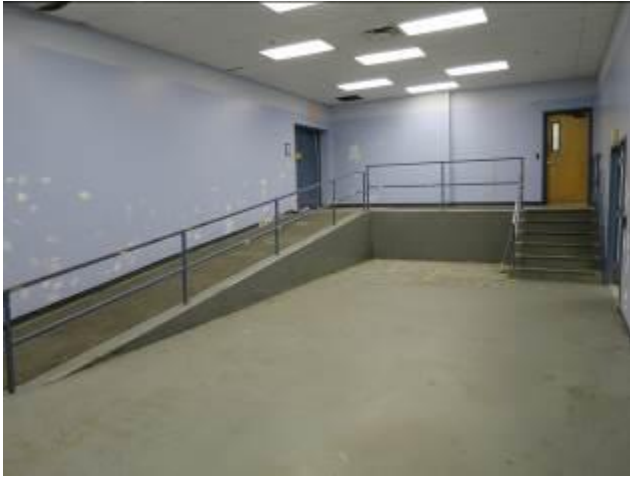
Varied Floor Levels In Vacant Building
