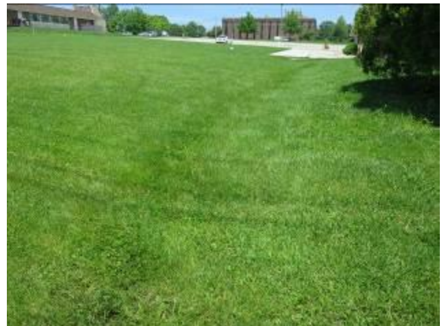
Swale (No Drainage) In SWC Of Vacant Building
