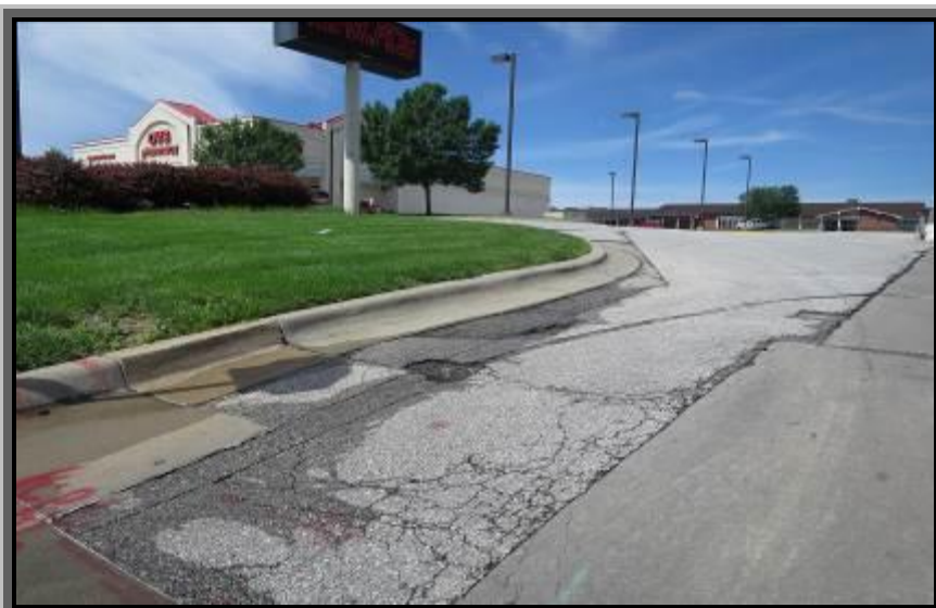
PHOTOGRAPH NO. 12: THE NE ENTRANCE FROM HOLMES ROAD
