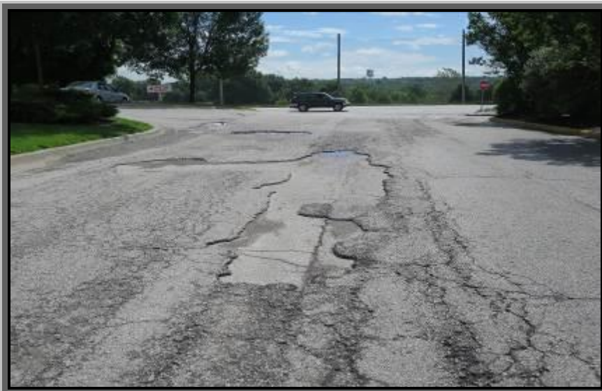
PHOTOGRAPH NO. 11: THE SE ENTRANCE FROM HOLMES ROAD
