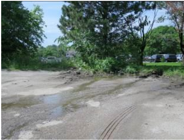
Trash & Standing Water & Mud
