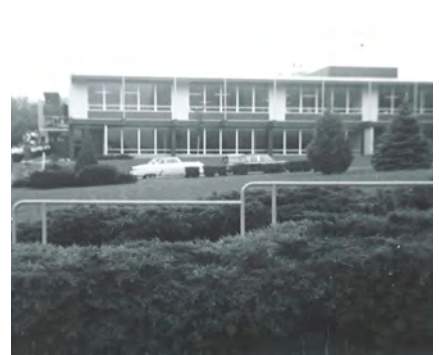
Photos of St. Francis Xavier School, under construction and in use during its early years.
