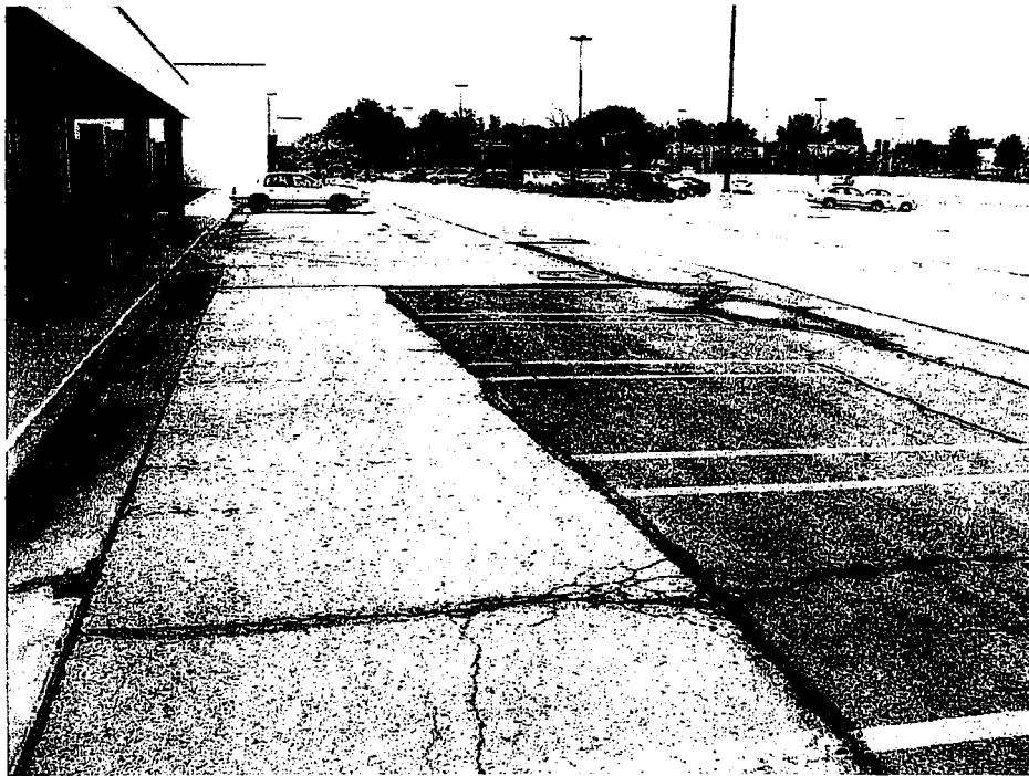
700 NE Barry Road – Deterioration of parking surface
