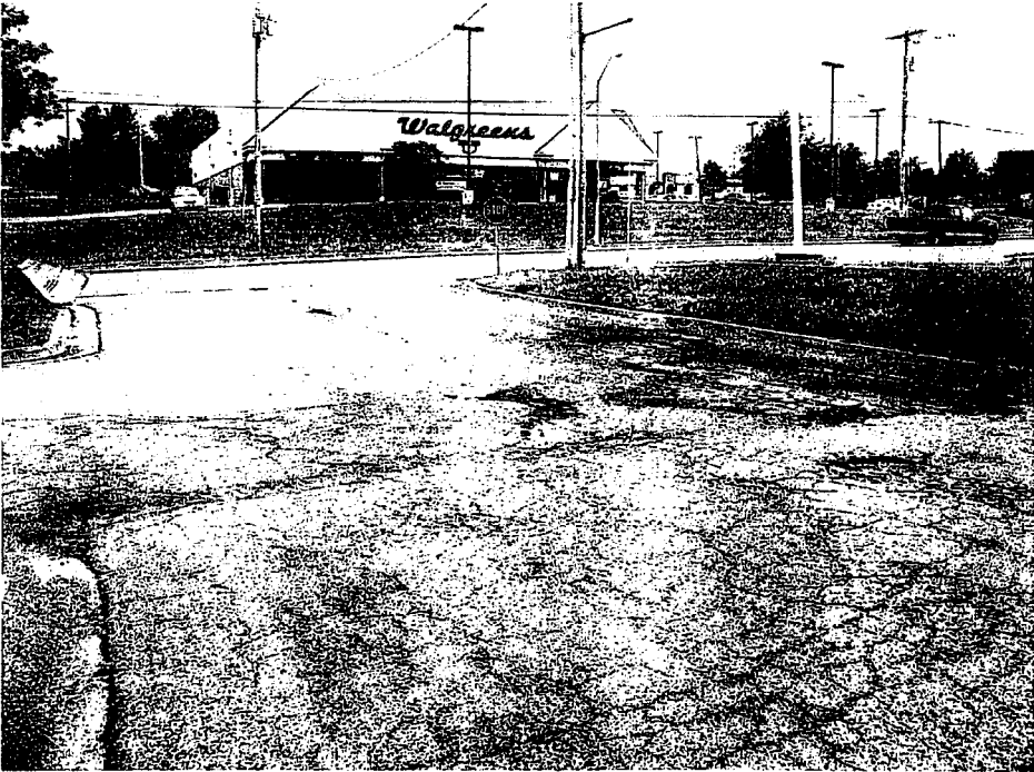
8405 N. Oak Trafficway – Deterioration of driveway; trash
