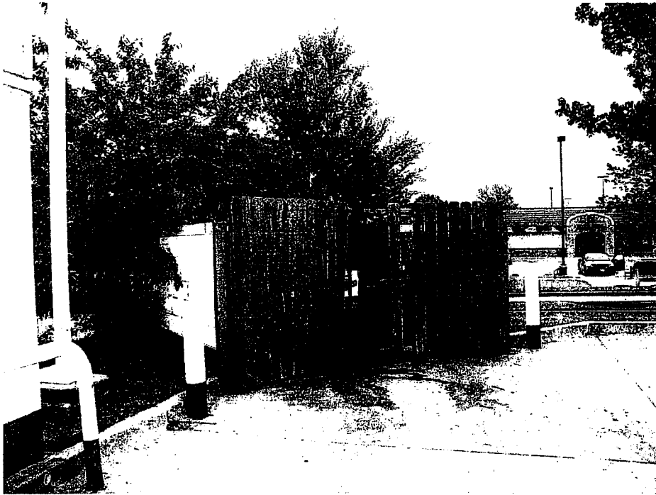
8401 N. Oak Trafficway – Deterioration of gates, walls; failure of finishes
