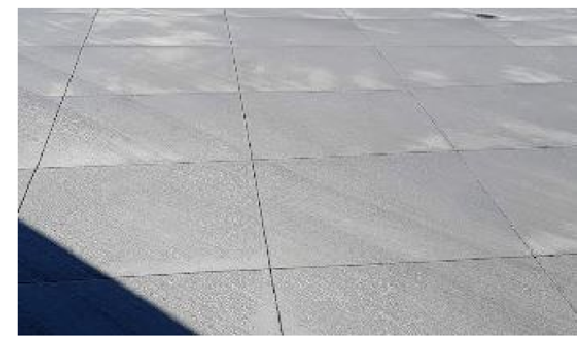
3 CROSSWALK PAVING DECORATIVE, DIAGONAL, SAWCUT PATTERN CONCRETE
