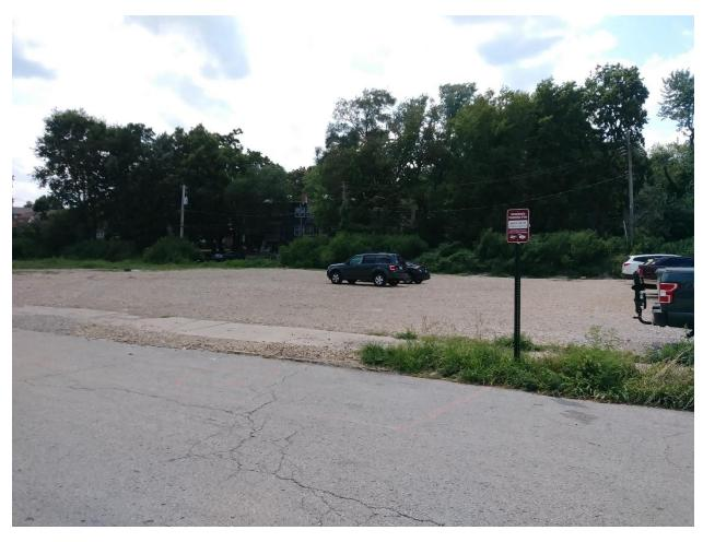
Gravel parking surface is not in conformance with City off-street parking standards; lock of driveway apron, weeds.
