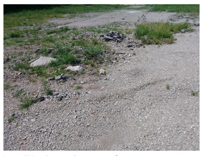
Pavement debris, weeds, uneven settling, note stormwater flow pattern
