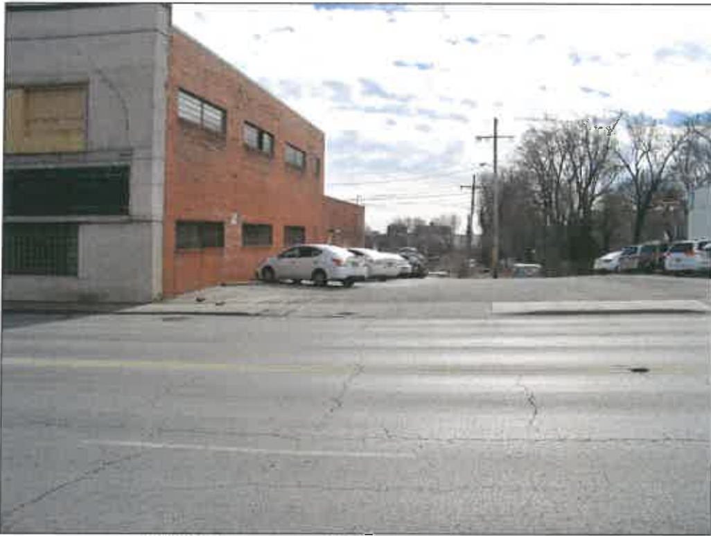
319 E. 31 st Street – looking south – lack of directional signage, pavement markings
