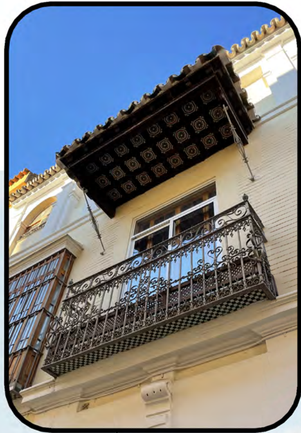
RESIDENTIAL BALCONY PRECEDENT: SEVILLE, SPAIN The alley-facing elevation features a wide variety of balcony types with ornamental metal railings and tiled soffits.
