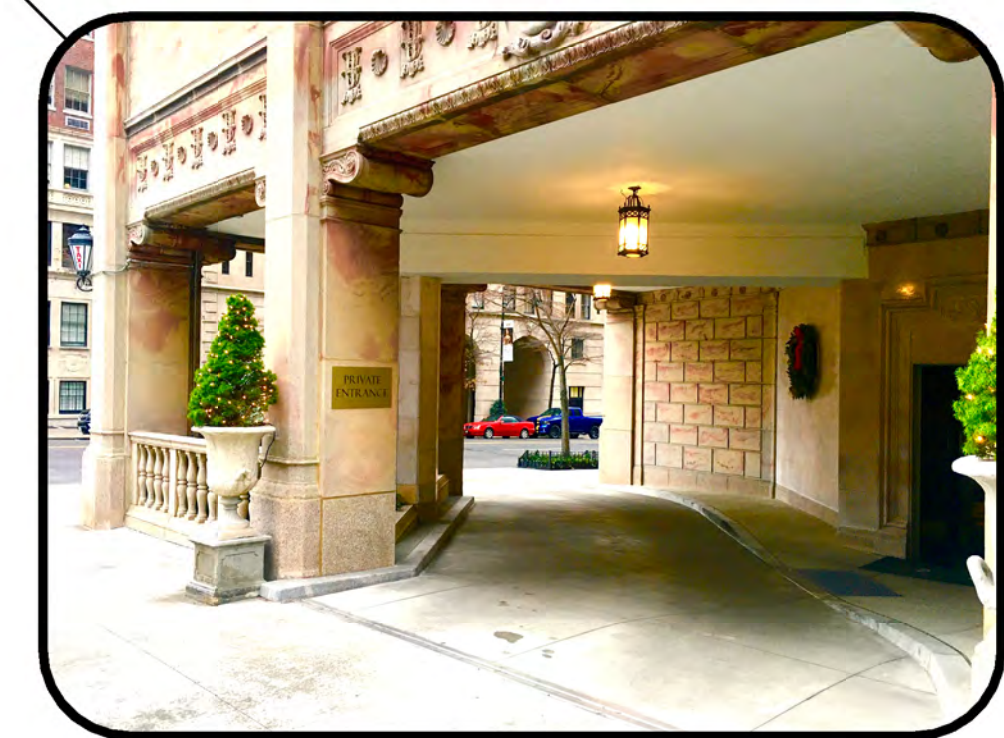
ENTRANCE ONLY DRIVEWAY, URBAN PORTE COCHERE: SUTTON PLACE, NEW YORK The upper level parking entrance is partially tucked under the building for convenient access to the lobby and amenity deck.
