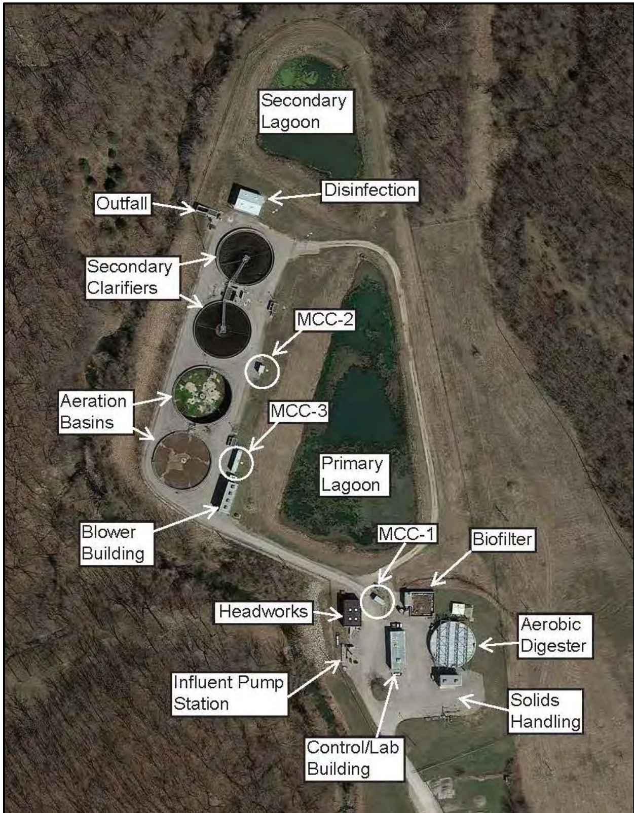
Figure 7-10: Rocky Branch WWTP Aerial Photograph
