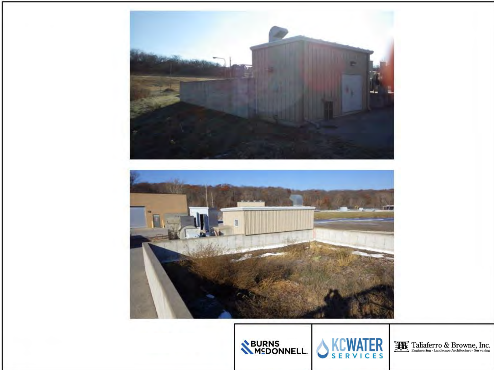
Figure 7-33: Biofilter Building Structural -
