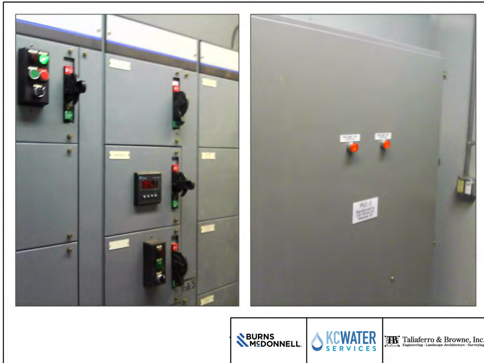
Figure 7-23: MCC-2 Building Electrical - MCC-2, PLC-2 - MCC-2
