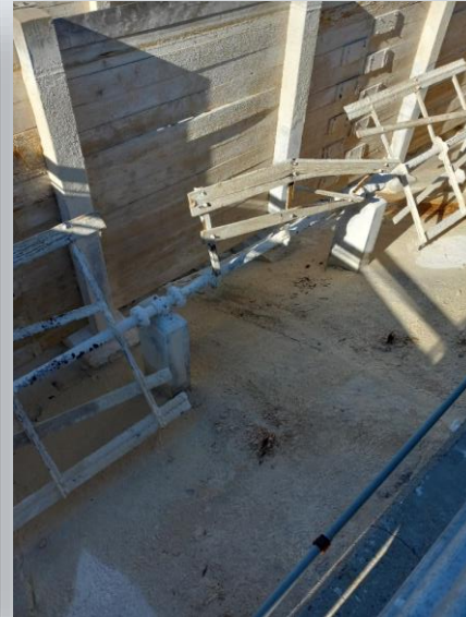
Secondary Improvements Project and Damaged Paddle on Air Wheel
