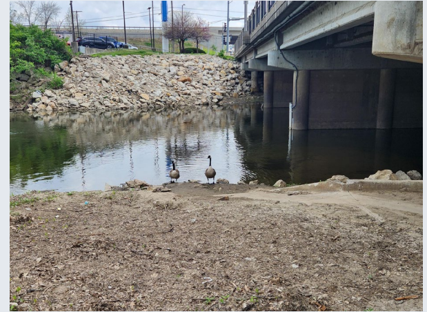
East side of Wornall Road Bridge
