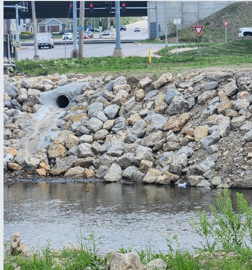
West side of Wornall Road Bridge at 103 rd Street
