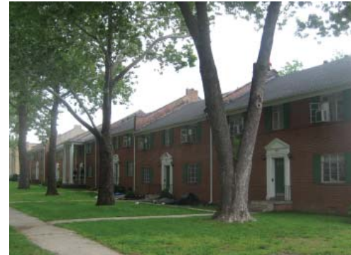
Art Gallery Apartments on the east side of Campbell
