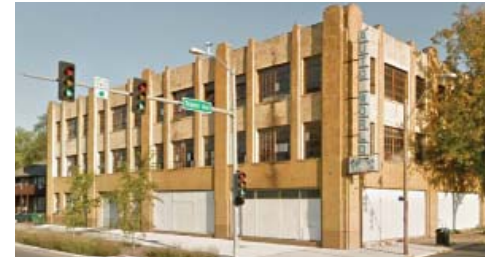
Former Auto World building
