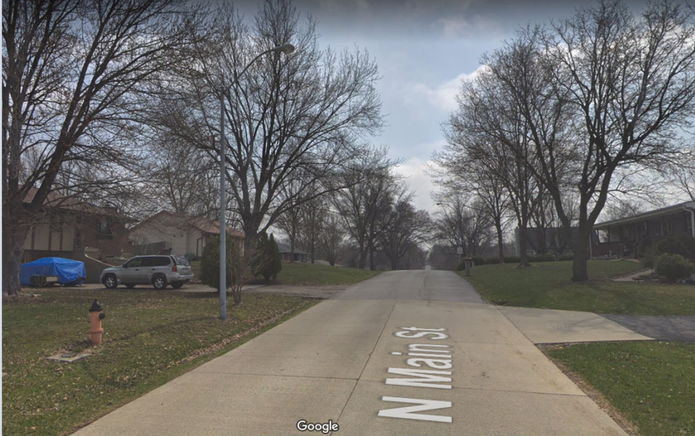
Looking south on N. Main Street
