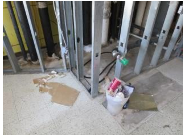
Water Damage – Scarritt Building
