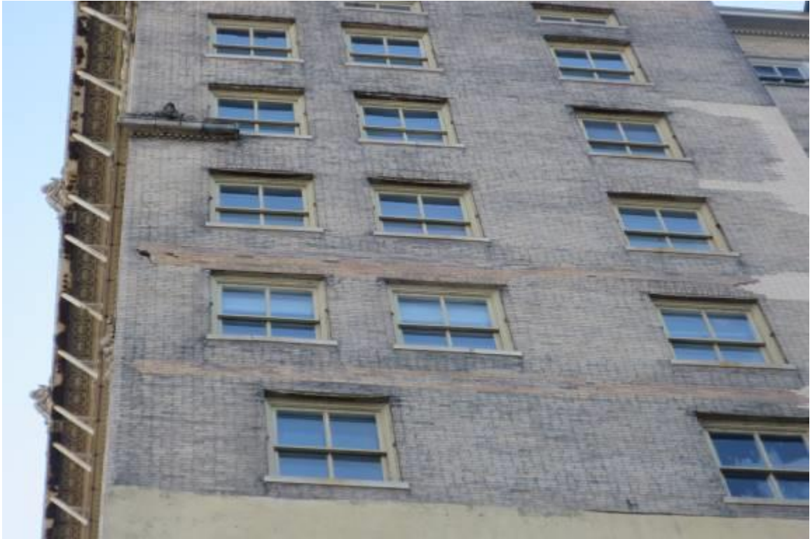
Deteriorating North & East Walls Of Arcade Lacking Window Space
