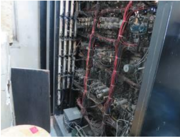
Obsolete Elevator Switchgear – Scarritt
