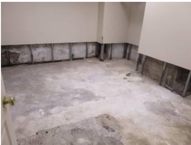
Water Damage – Scarritt Building
