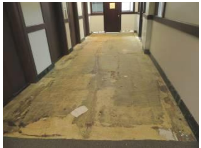
Water Damage – Scarritt Building
