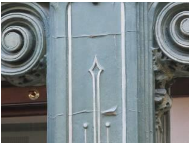
Water Damage From Skylight Leak – Arcade
