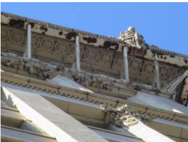
Deteriorating Cornice Work – 11 th Floor Of Scarritt
