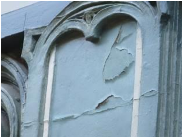
Lightwell Damage – Arcade
