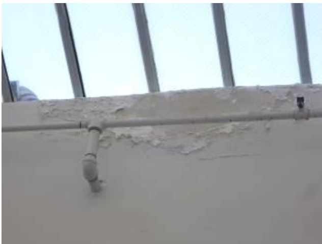
Water Damage From Skylight Leak – Arcade
