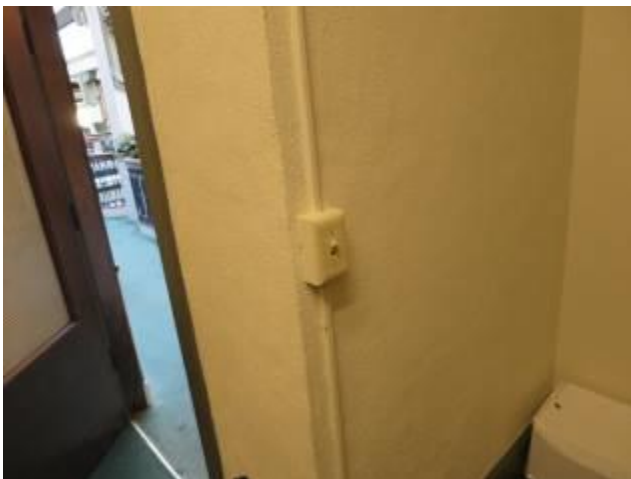
Electrical Wall Strips – Arcade
