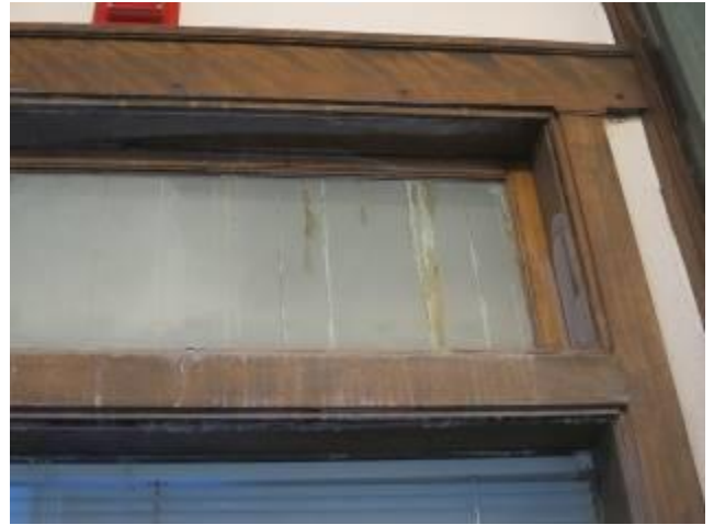
Water Damage From Ceiling Leak – Arcade
