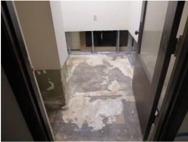
Water Damage – Scarritt Building
