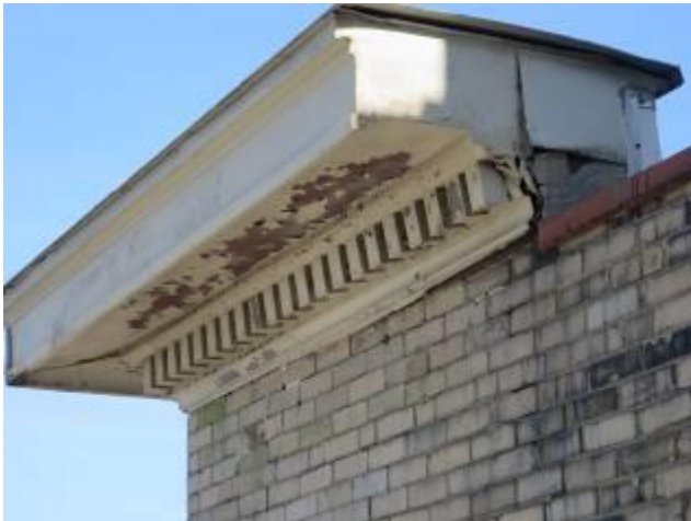
Deteriorating Cornice – West Elevation Scarritt
