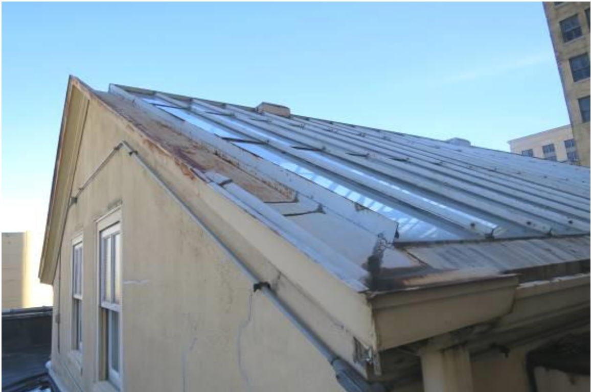
Deteriorating & Rusting Skylight Supports & Drainage – Above Arcade Lightwell
