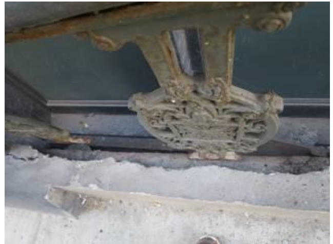
Failed Security Railing – Scarritt – E 9 th Street
