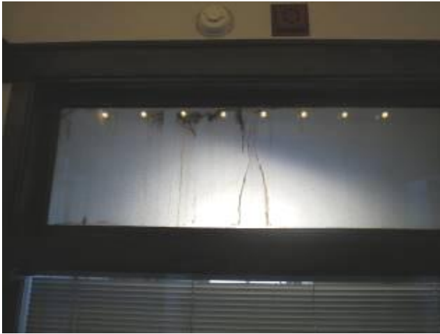
Water Damage From Ceiling Leak – Arcade
