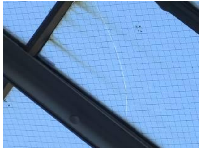
Broken Glass Pane In Skylight – Arcade
