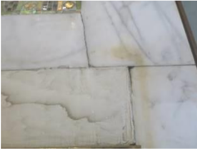
Water Damaged Marble – Scarritt Building
