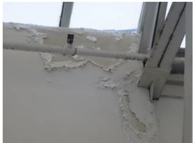
Water Damage From Skylight Leak – Arcade
