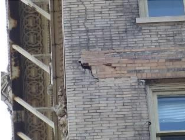
Dislodged Bricks – North Elevation Scarritt
