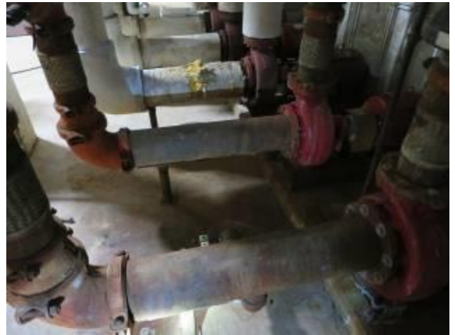
Compromised Pipe Wrapping – Scarritt
