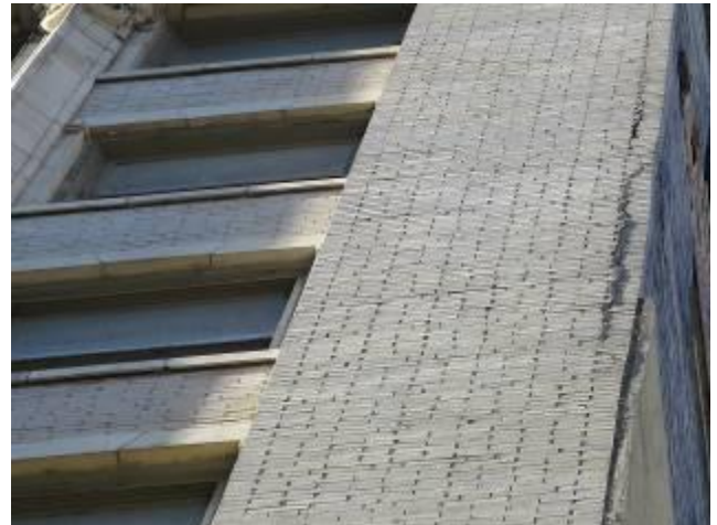
Vertical Brick Failure – East Elevation Scarritt
