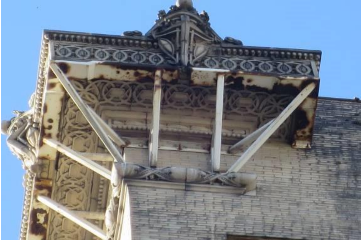
Rusting Bracing Added To Cornice Work – 11 th Floor Of Scarritt Building Above Grand Blvd.
