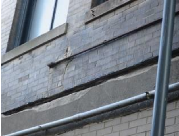
Spalling Ashlar – West Elevation Scarritt
