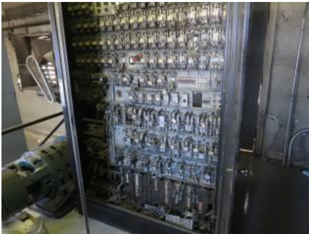
Obsolete Elevator Switchgear – Scarritt
