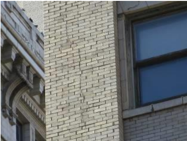
Vertical Brick Failure – East Elevation Scarritt
