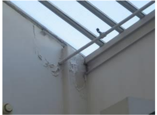
Water Damage From Skylight Leak – Arcade
