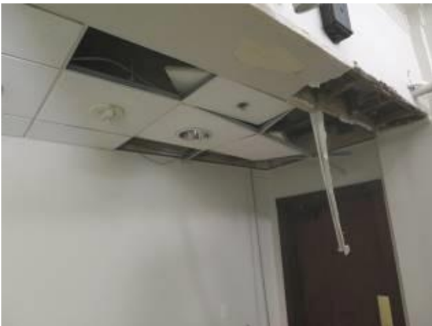
Collapsing Ceiling – Scarritt
