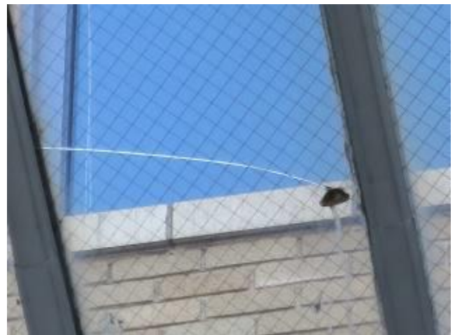
Broken Glass Pane In Skylight – Arcade
