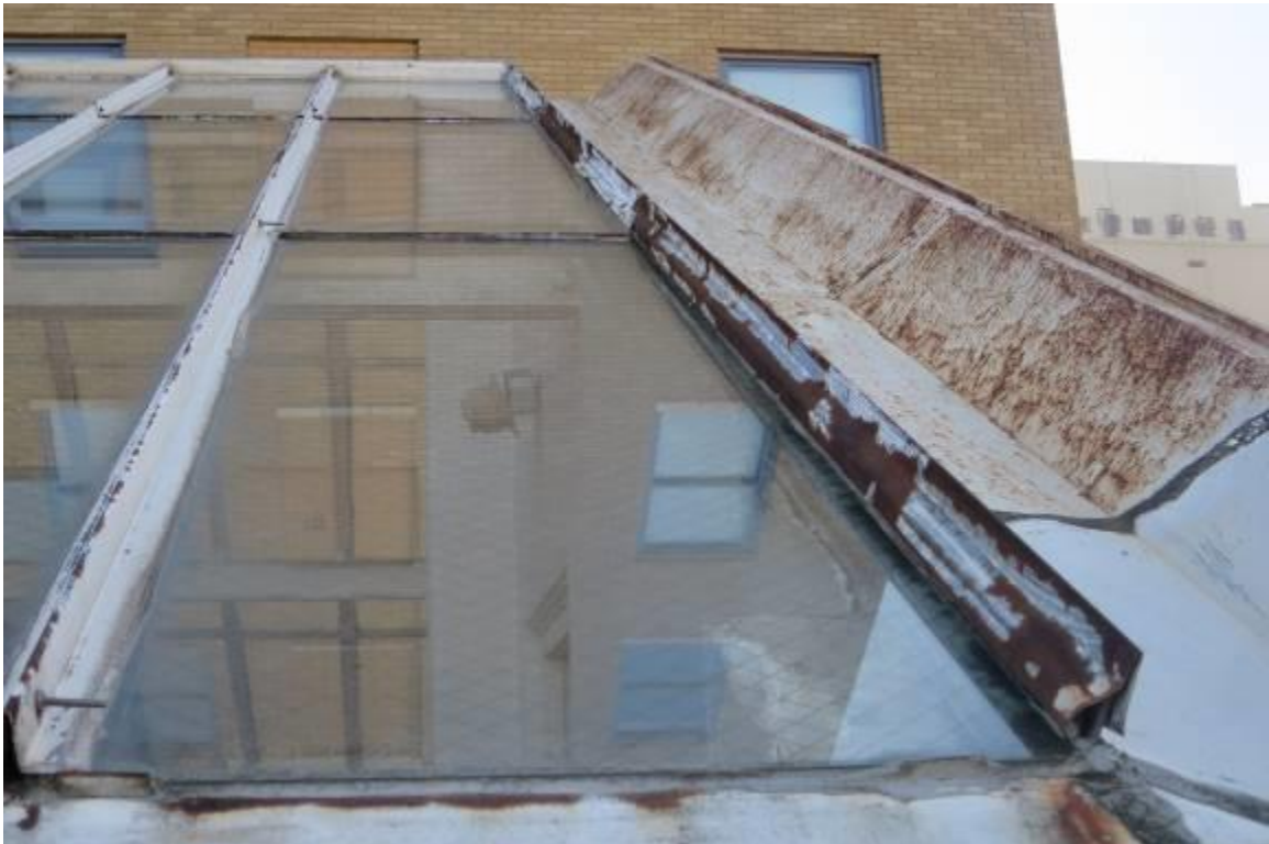
Deteriorating & Rusting Skylight Supports – Above Arcade Lightwell
