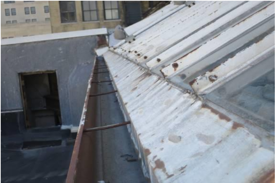
Deteriorating & Rusting Skylight Supports & Drainage – Above Arcade Lightwell
