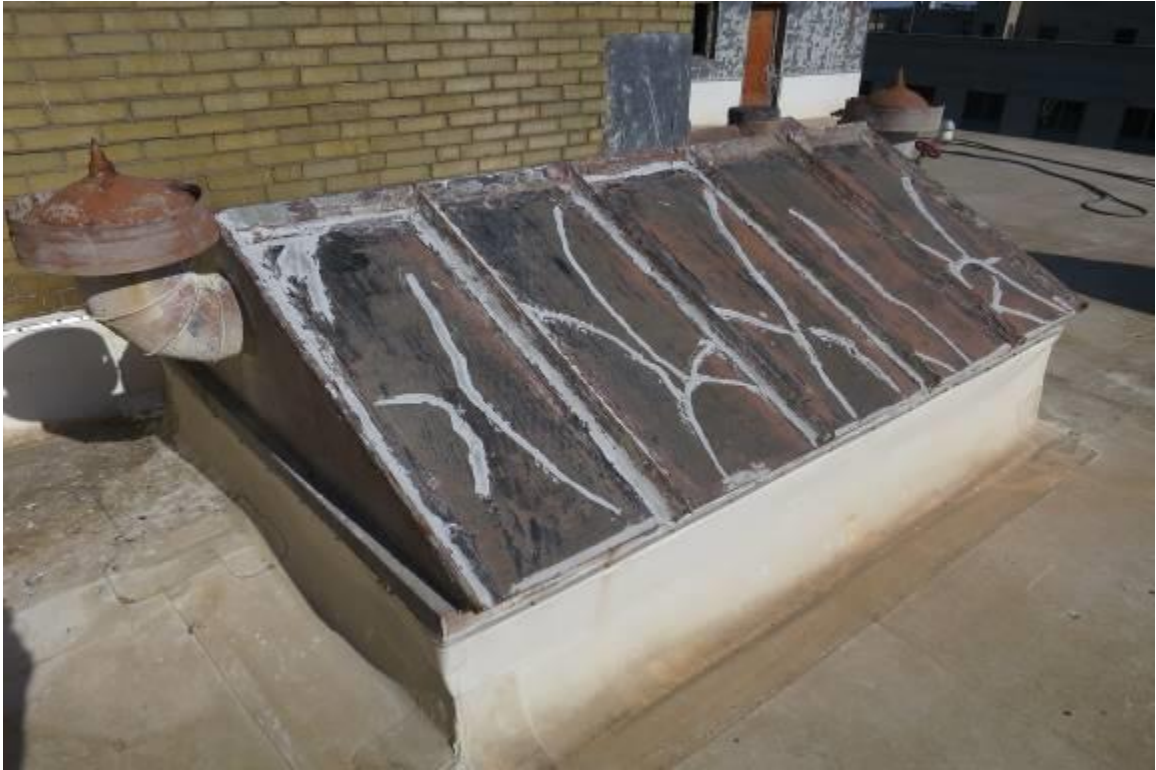
Deteriorating Freight Elevator Penthouse – Scarritt Building
