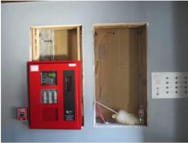
Fire Panel Replacement After Theft – Scarritt
