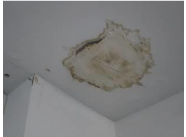
Ceiling Leak – Arcade
