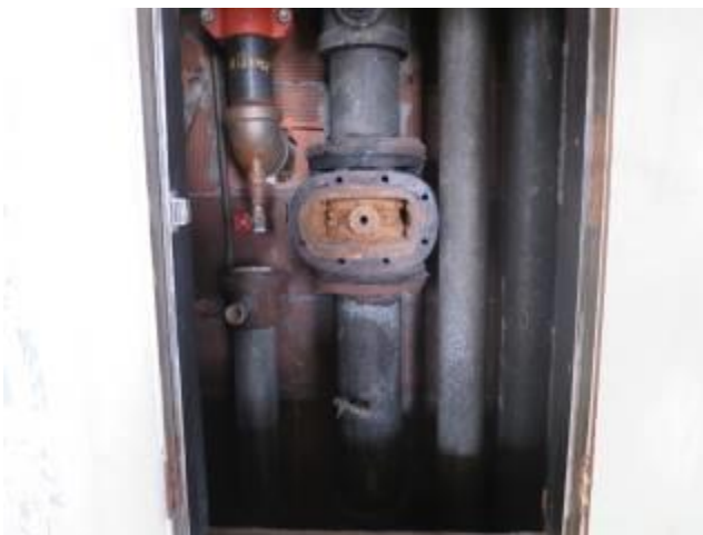
Potential Lead-Based Piping – Scarritt
