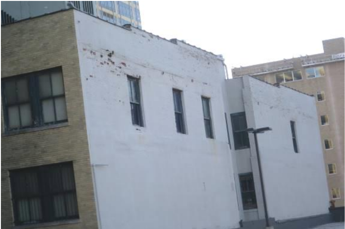
Deteriorating North & East Walls Of Arcade Lacking Window Space
