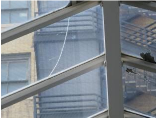
Broken Glass Pane In Skylight – Arcade
