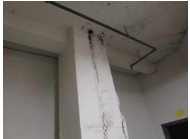
Water Damage – Scarritt Building
