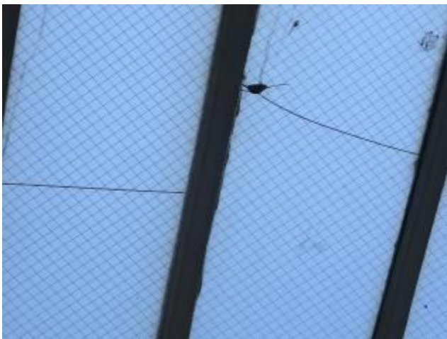
Broken Glass Pane In Skylight – Arcade
