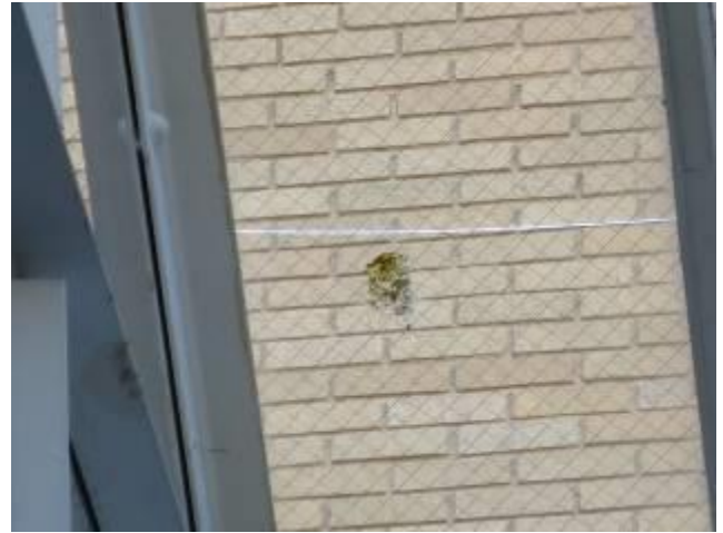
Broken Glass Pane In Skylight – Arcade
