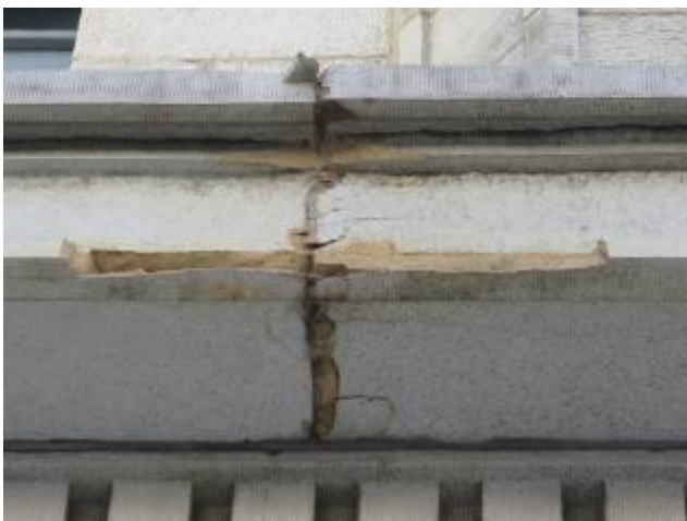
Spalling Ashlar – East Elevation Scarritt
