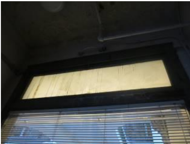
Water Damage From Ceiling Leak – Arcade
