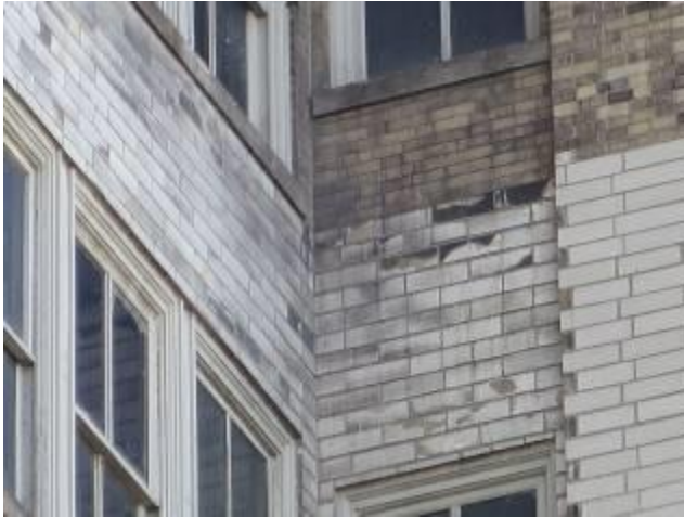
Spalled Brick Faces – North Elevation Scarritt
