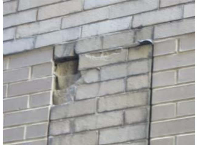
Dislodged Brick – West Elevation Scarritt
