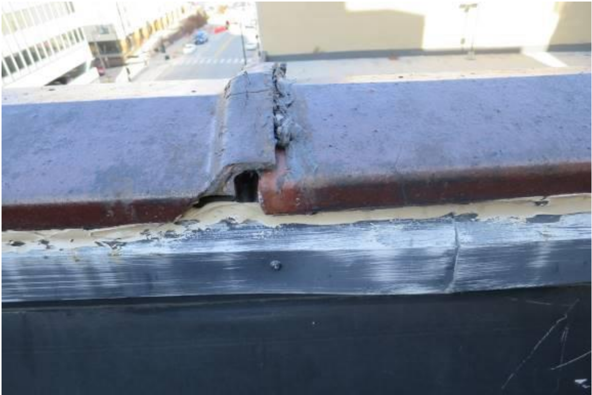
Tile Copping Damage – Arcade
