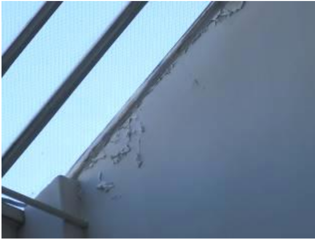
Water Damage From Skylight Leak – Arcade
