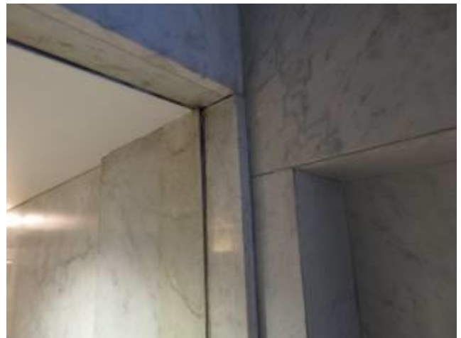
Shifting/Settling Marble Panels – Arcade
