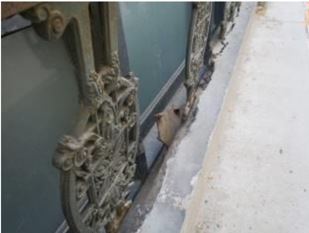
Failed Security Railing – Scarritt – E 9 th Street
