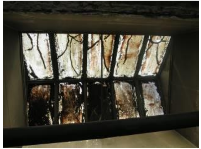
Scarritt Building – Aging Skylight
