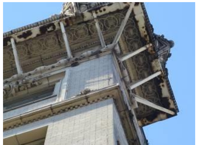
Deteriorating Cornice Work – 11 th Floor Of Scarritt
