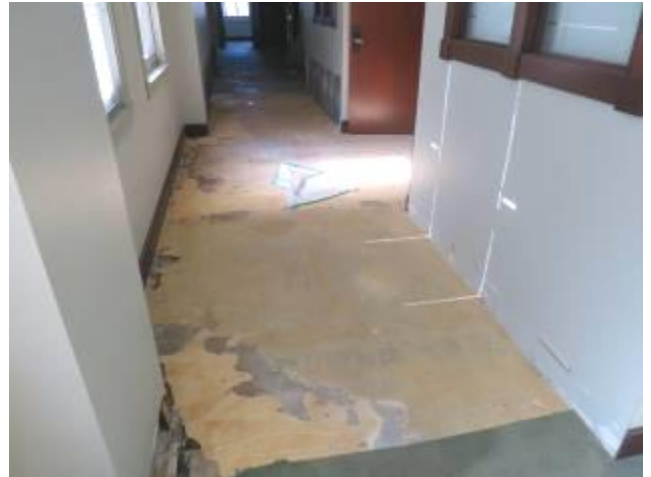
Water Damage – Scarritt Building
