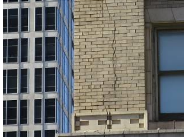
Vertical Brick Failure – East Elevation Scarritt
