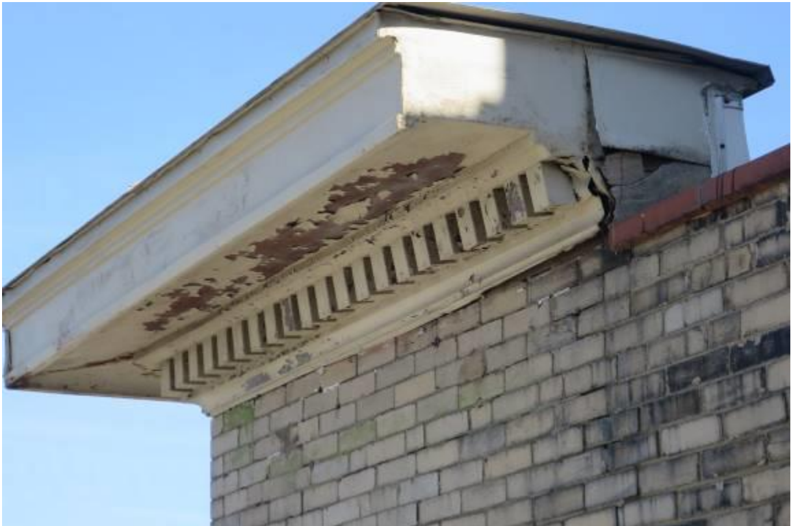
Deteriorating Cornice – 12 th Floor Scarritt Building
