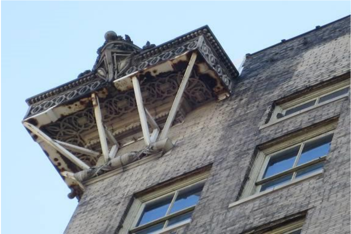
Deteriorating Cornice – 12 th Floor Scarritt Building
