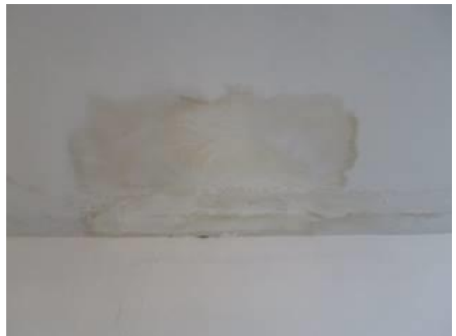
Water Damage From Ceiling Leak – Arcade
