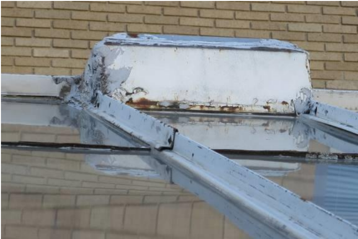
Deteriorating & Rusting Skylight Supports – Above Arcade Lightwell
