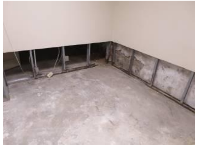
Water Damage – Scarritt Building
