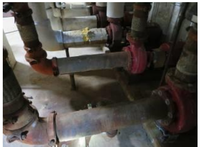
Potential Lead-Based Piping – Scarritt
