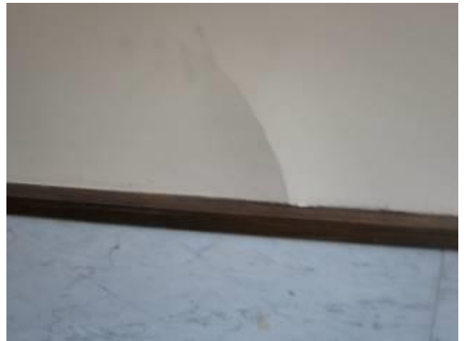
Water Damage From Ceiling Leak – Arcade
