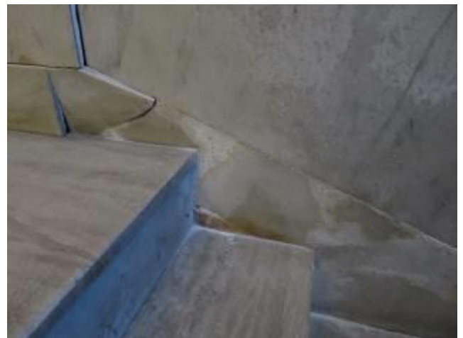
Water Damage – Scarritt Building
