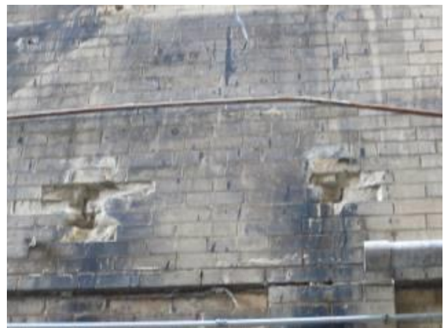
Dislodged Brick – West Elevation Scarritt
