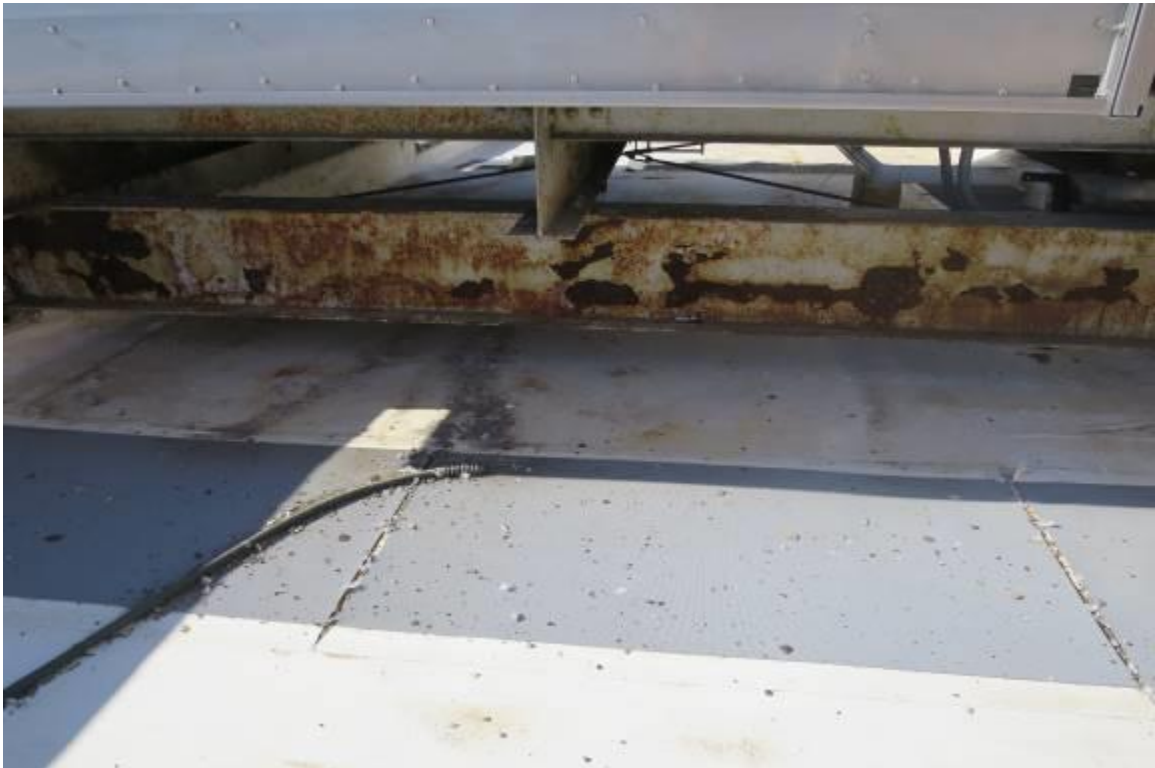
Deteriorating Cooling Tower Supports – Scarritt Building
