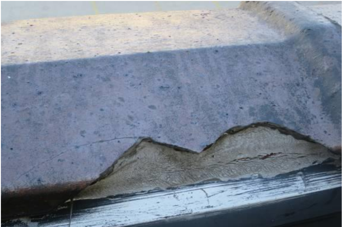
Tile Copping Damage – Arcade
