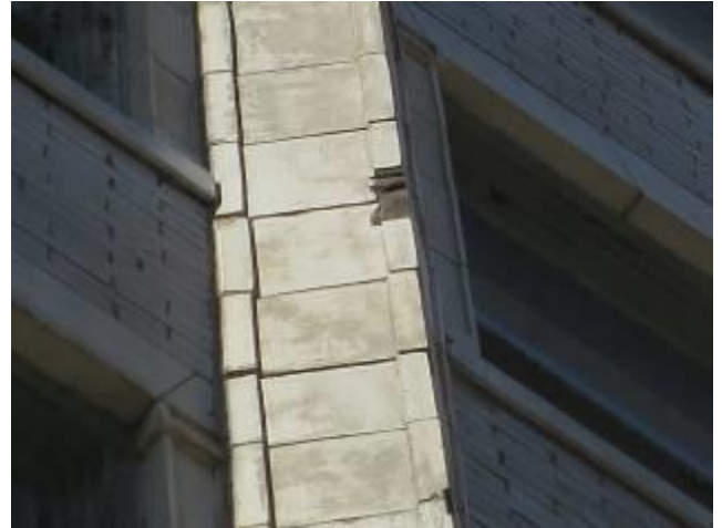
Dislodged Ashlar Face – East Elevation Scarritt
