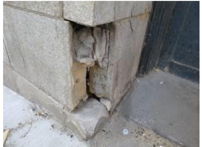
Dislodged Ashlar – South Elevation Scarritt
