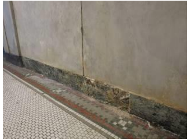
Water Damaged Marble – Arcade
