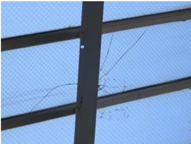
Broken Glass Pane In Skylight – Arcade
