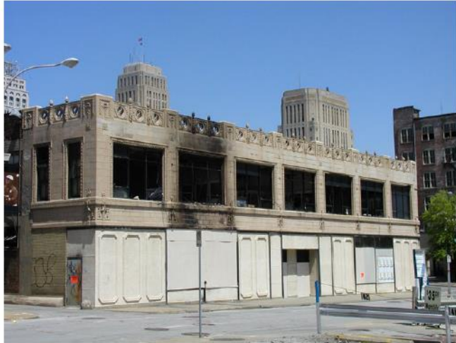
NW Corner of 14 th & Walnut Street
