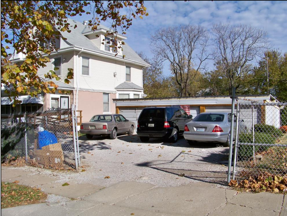
3043 Park Avenue – Poor vehicular access; deterioration of parking surface; trash/debris
