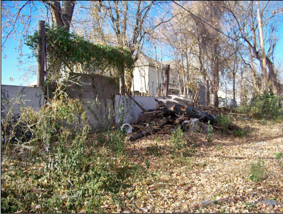
2926 Euclid Avenue – Trash/debris; overgrown vegetation
