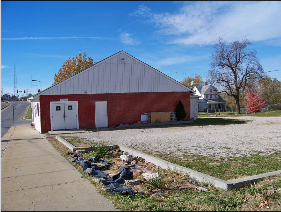
2108 E. 31 st Street – deterioration of parking surface
