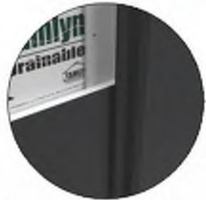
Fiber Cement Siding, Typ
