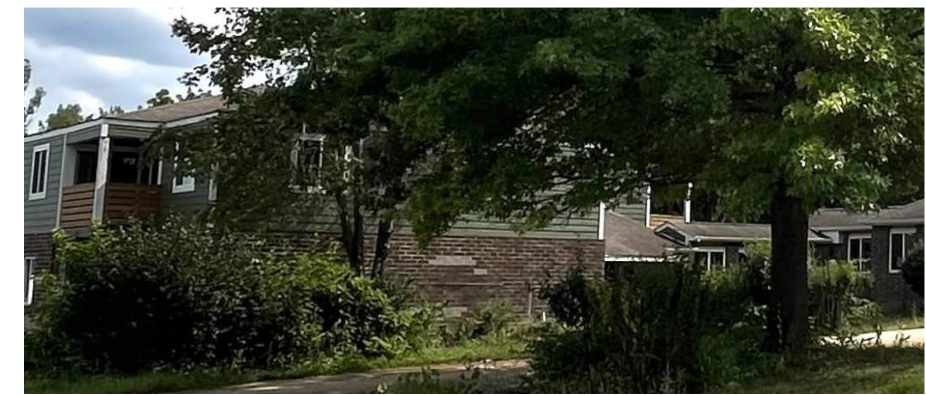
BUILDING 400 NORTHWEST ELEVATION
