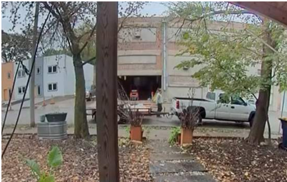
1/12/26 9:05AM; 10/7/25: Select examples of dispatch center and materials loading, spilling onto street/blocking street.
