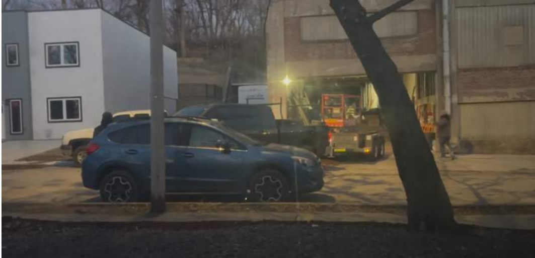
1/21/26 5:47PM: Select example of over-sized construction equipment being backed into northern-most bay with multi-point turns next to residential traffic.
