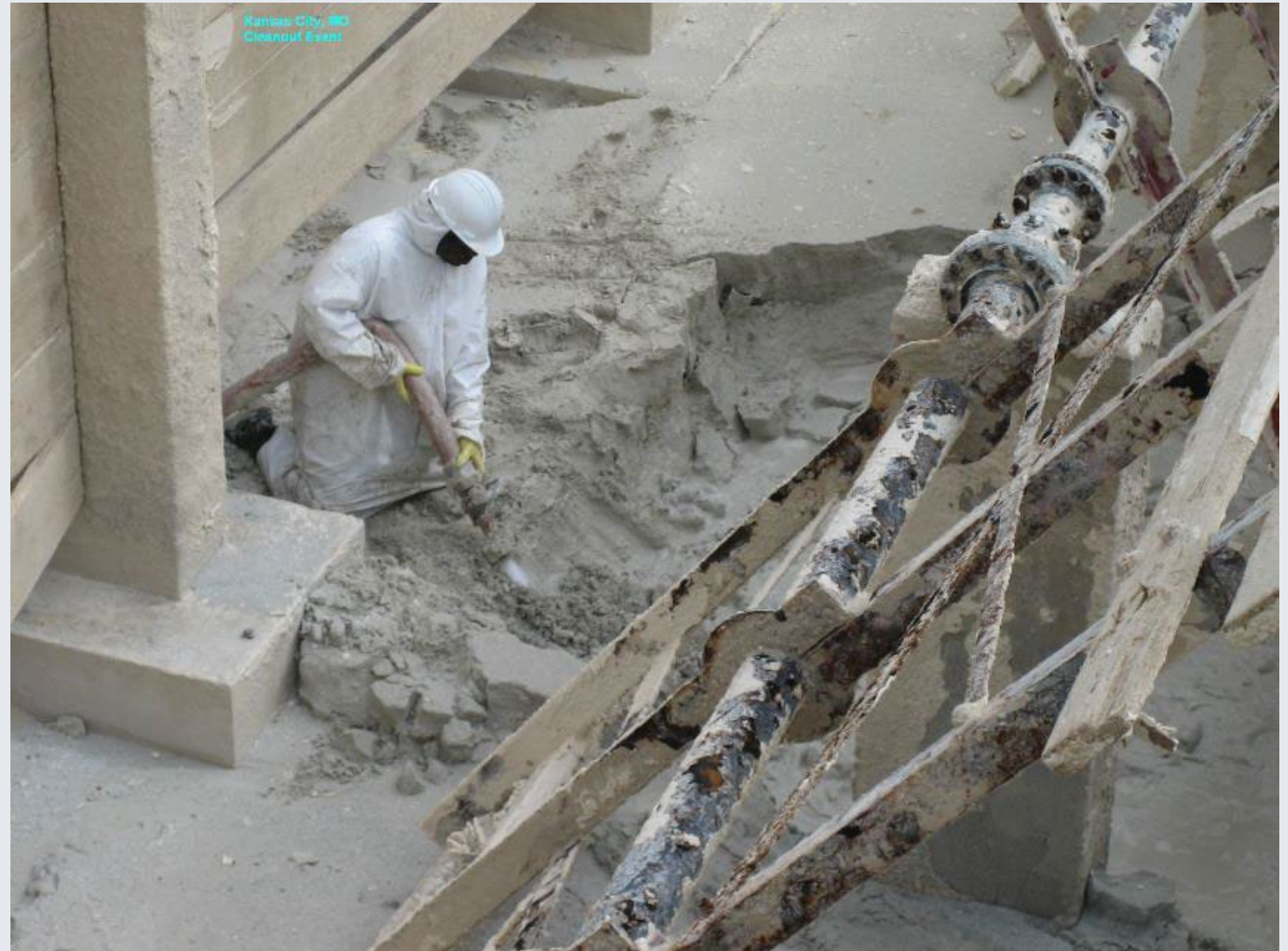
Water Treatment Plant Basin Cleanout Event
