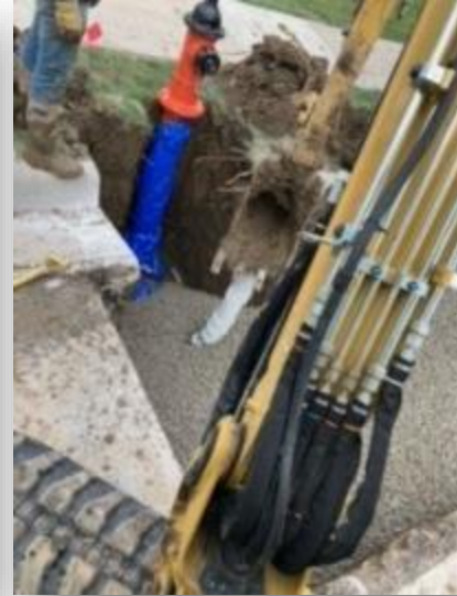
Installing a New Fire Hydrant
