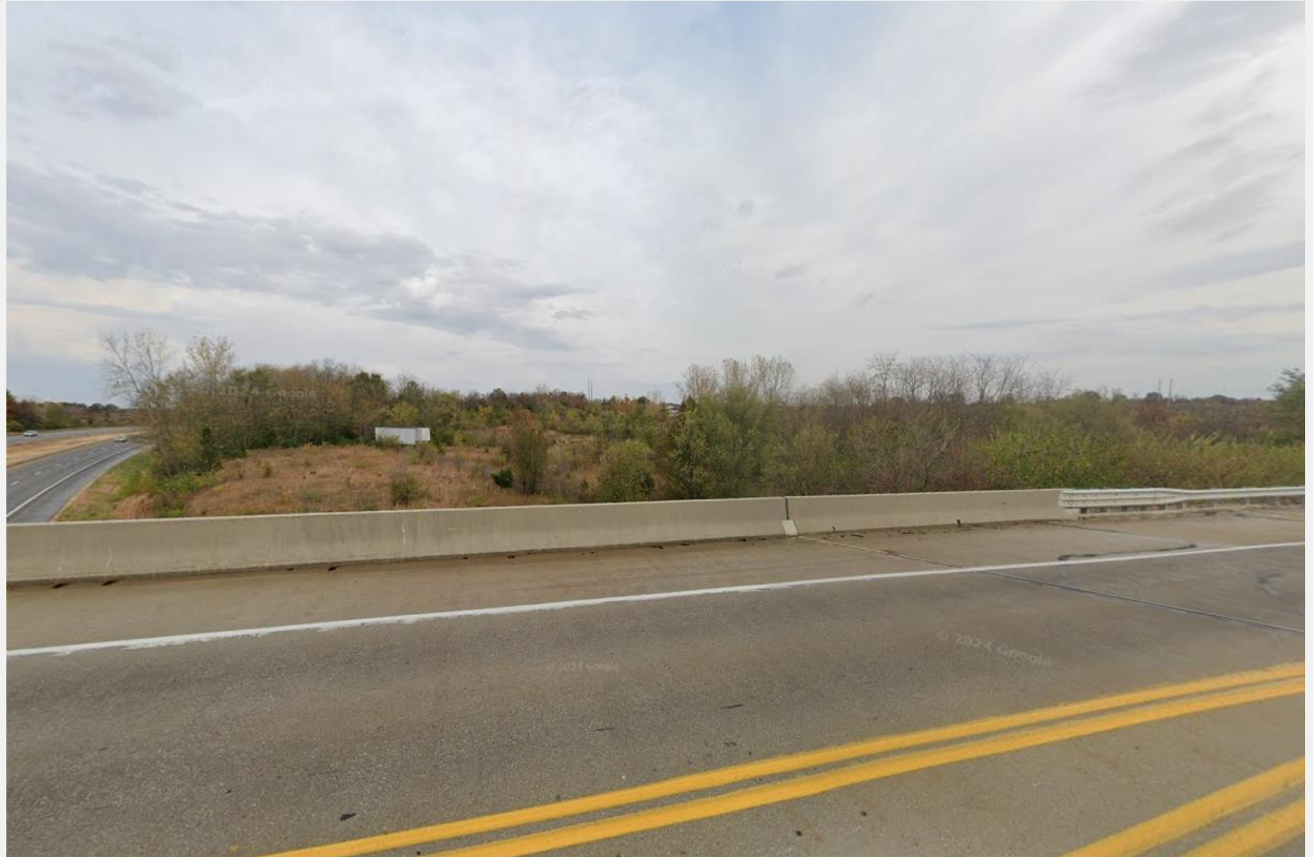
Looking north on NE Barry Rd. (Oct 2024)
