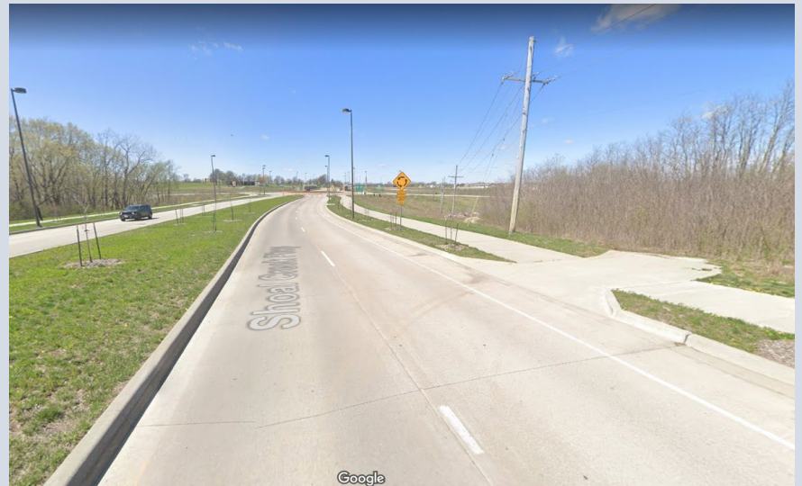
Shoal Creek Parkway looking west 7
