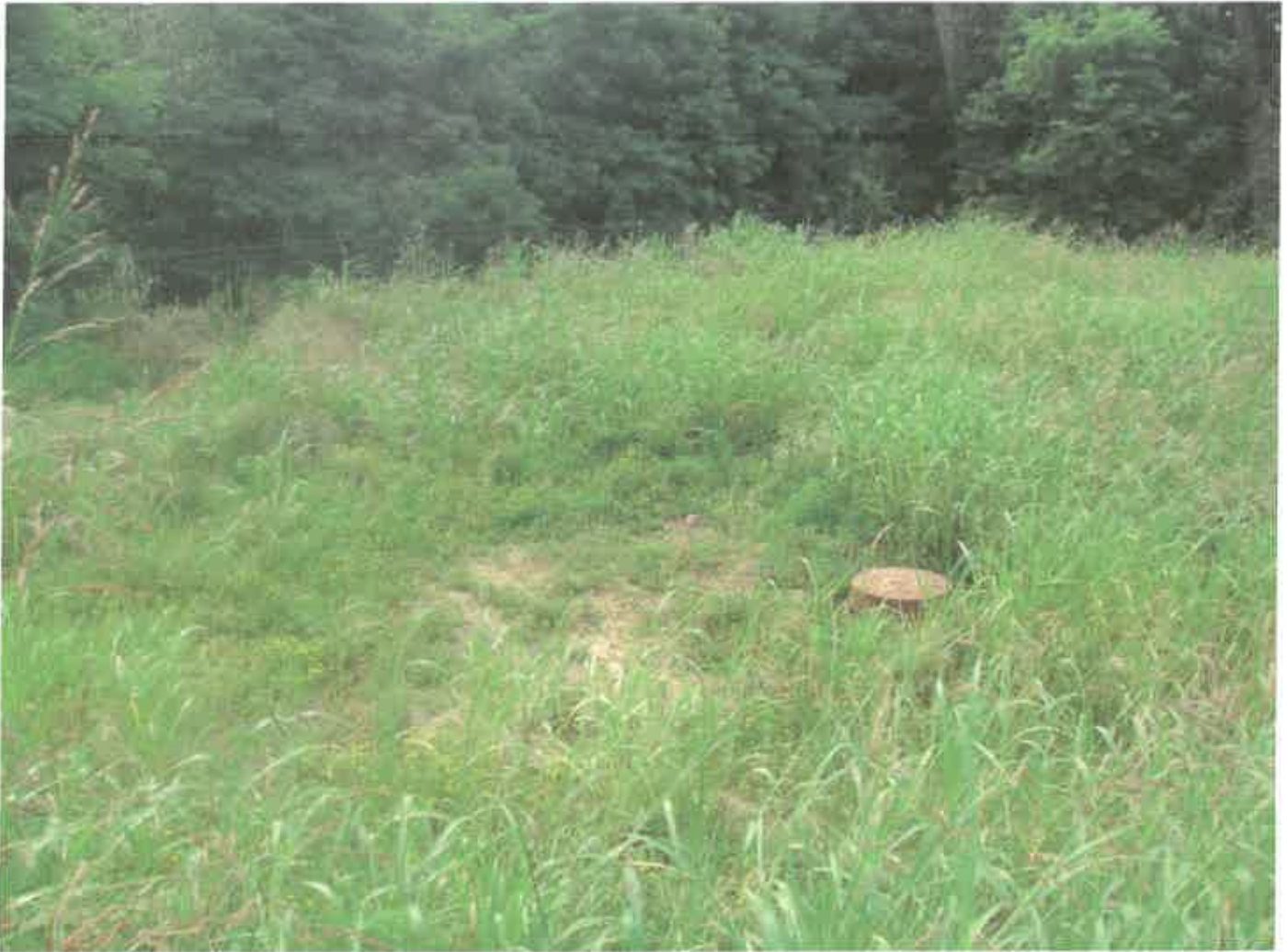
Photo 10 - Storm water sewer manhole access location at eastern portion of site.
