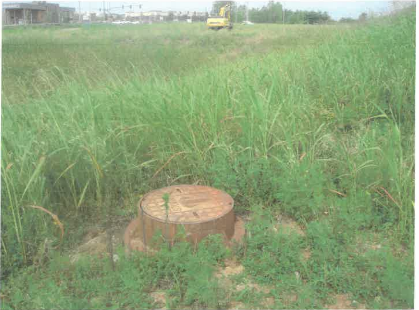
Photo 11 - View of storm sewer access looking west.
