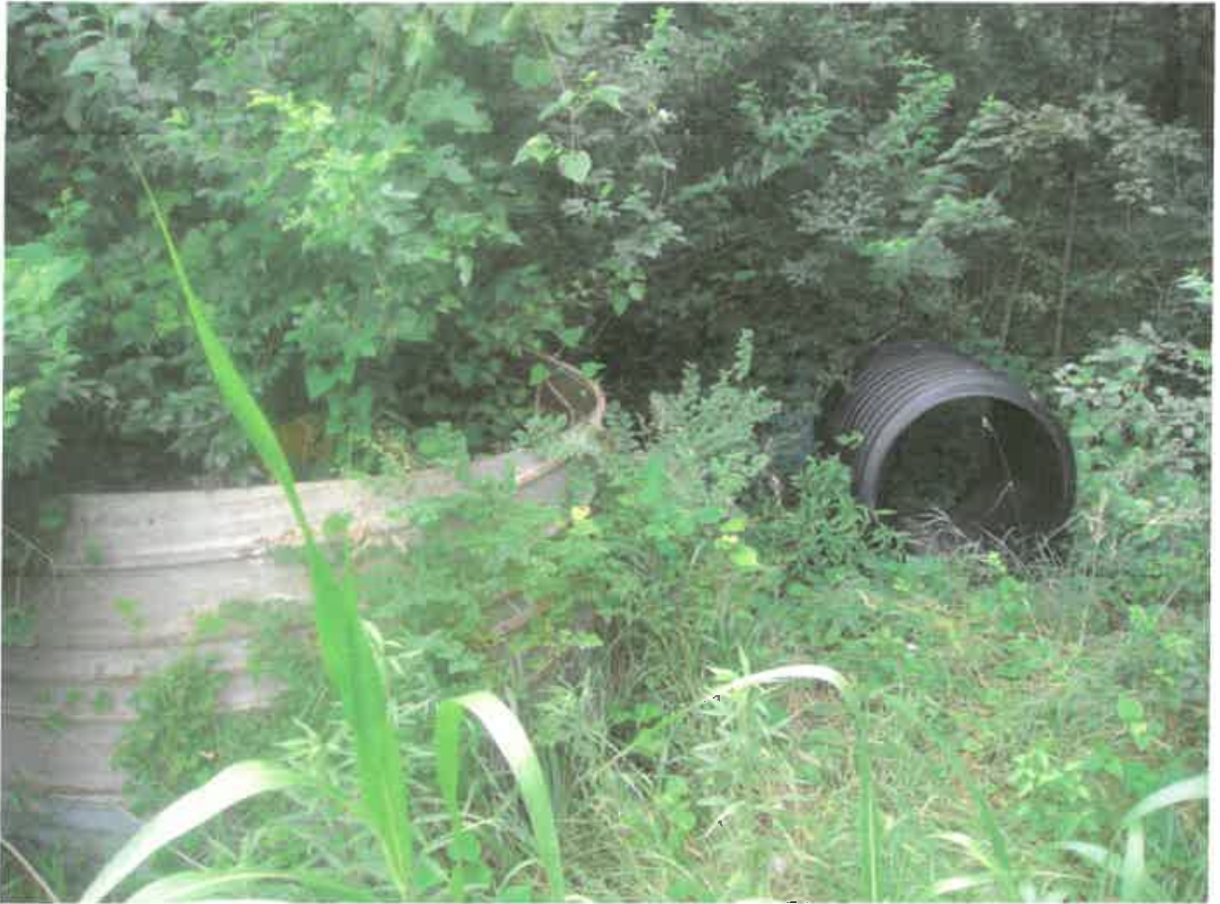
Photo 8 - Excess storm water culvert left in this location.
