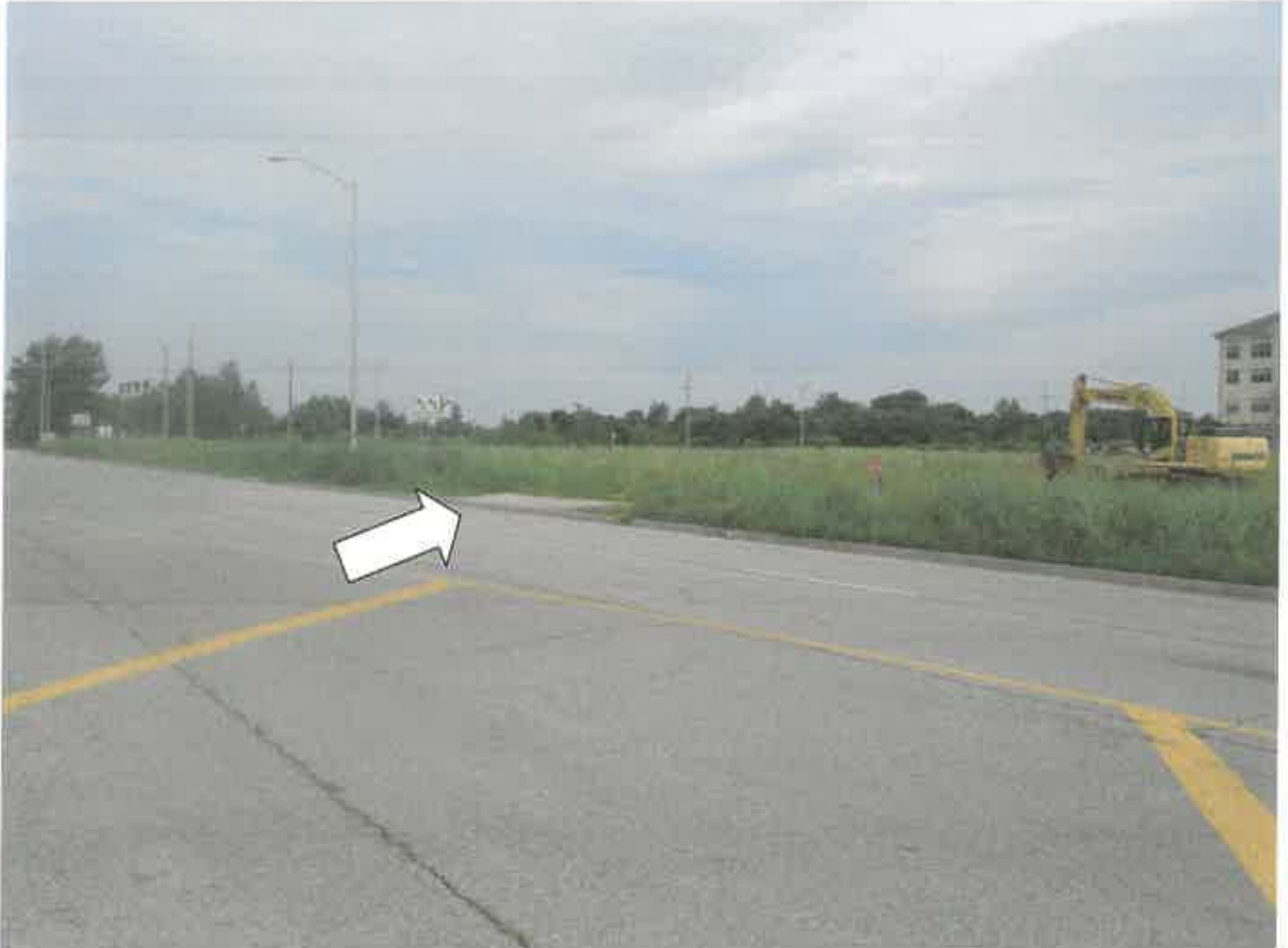
Photo 9 - View of southern property boundary as it meets NW 88 th Street. Arrow indicates where vehicular access will have to be constructed.
