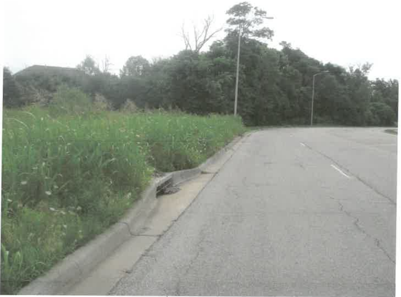
Photo 4 - View east along NW 88 th Street. Note storm-water inlet. Also note absence of sidewalk, pedestrian connectivity.
