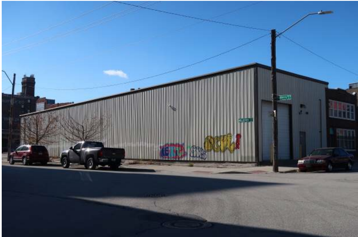
Looking Southwest At The East (Mulberry Street) & North Elevation Of 1301 Union Avenue
