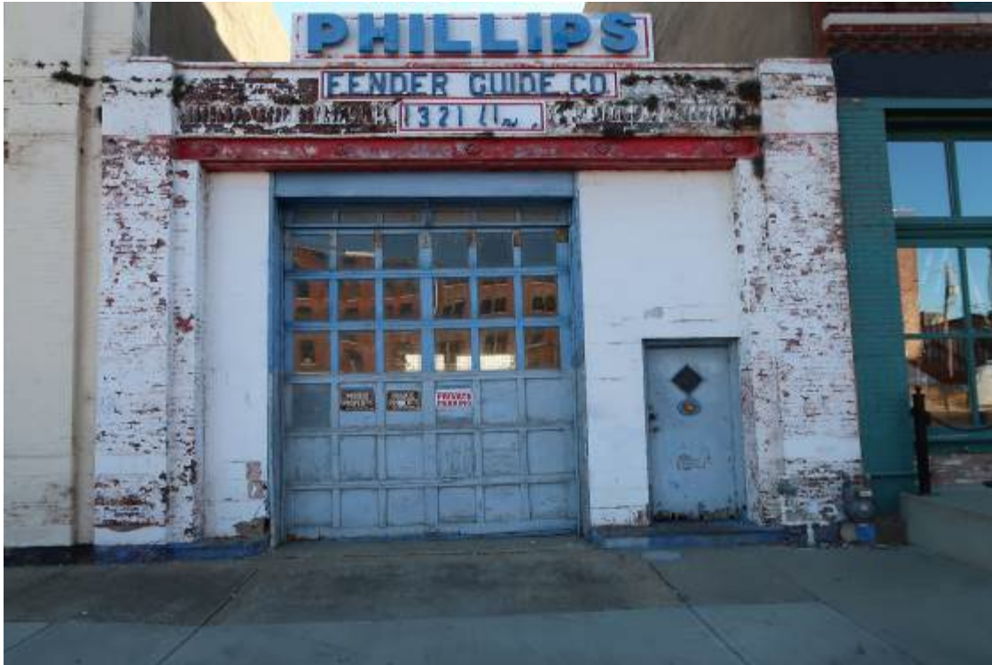
The Front Elevation Of The Westerly Adjoining Blighted Property
