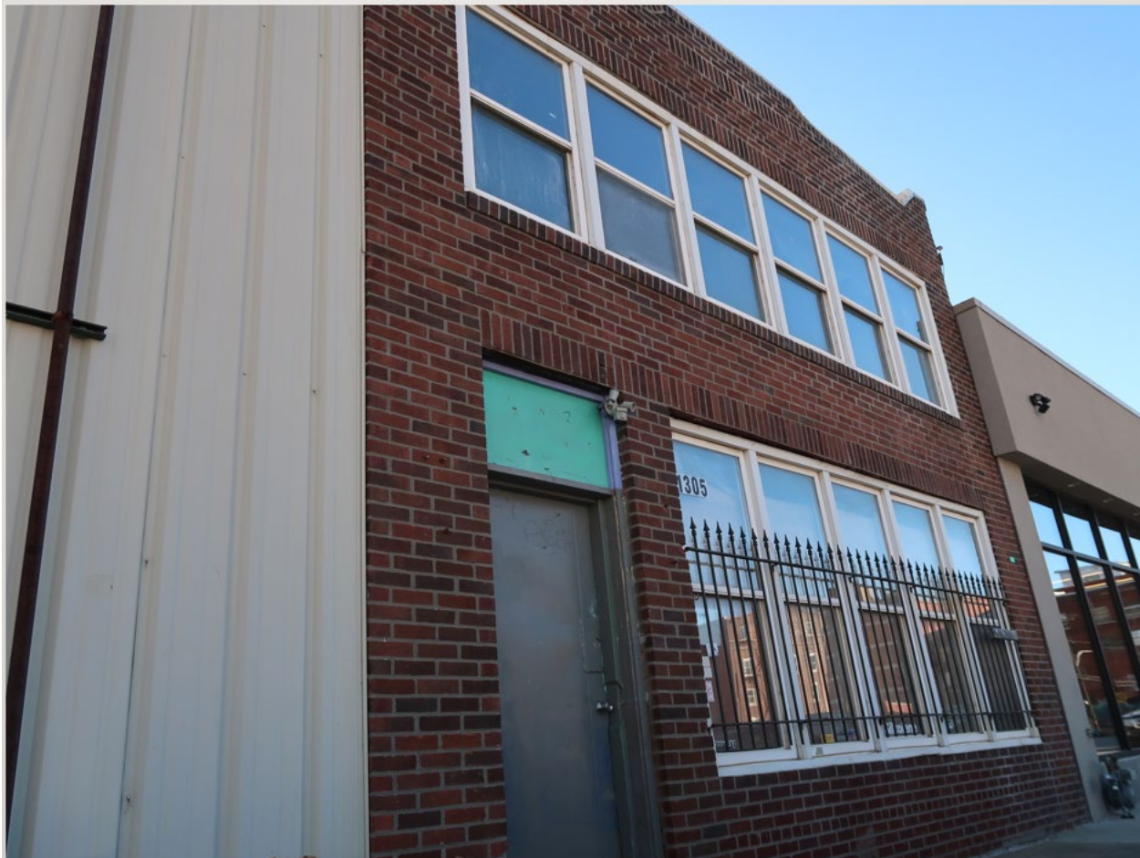
Looking Southwest At The Front (North) Elevation Of 1305 Union Avenue
