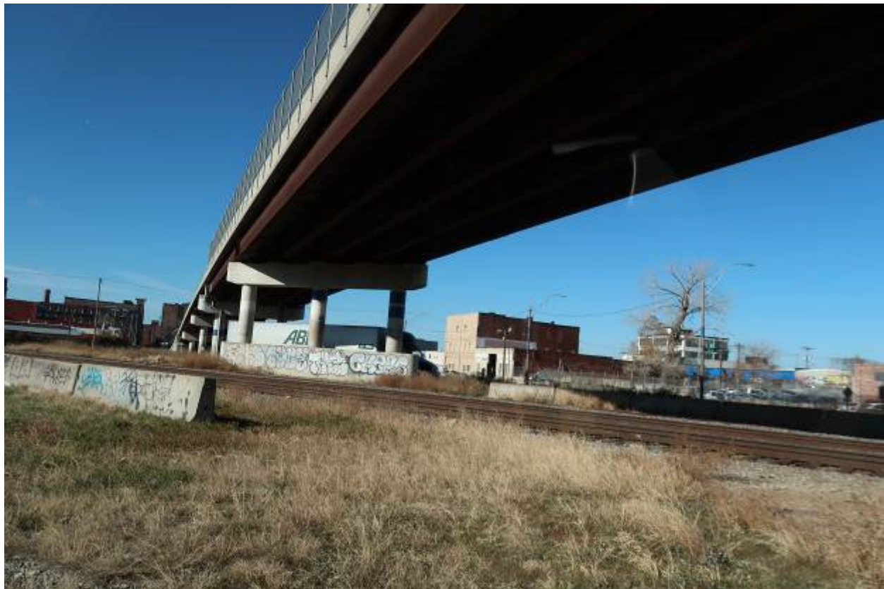
Looking Northwest Across 912 Santa Fe Street
