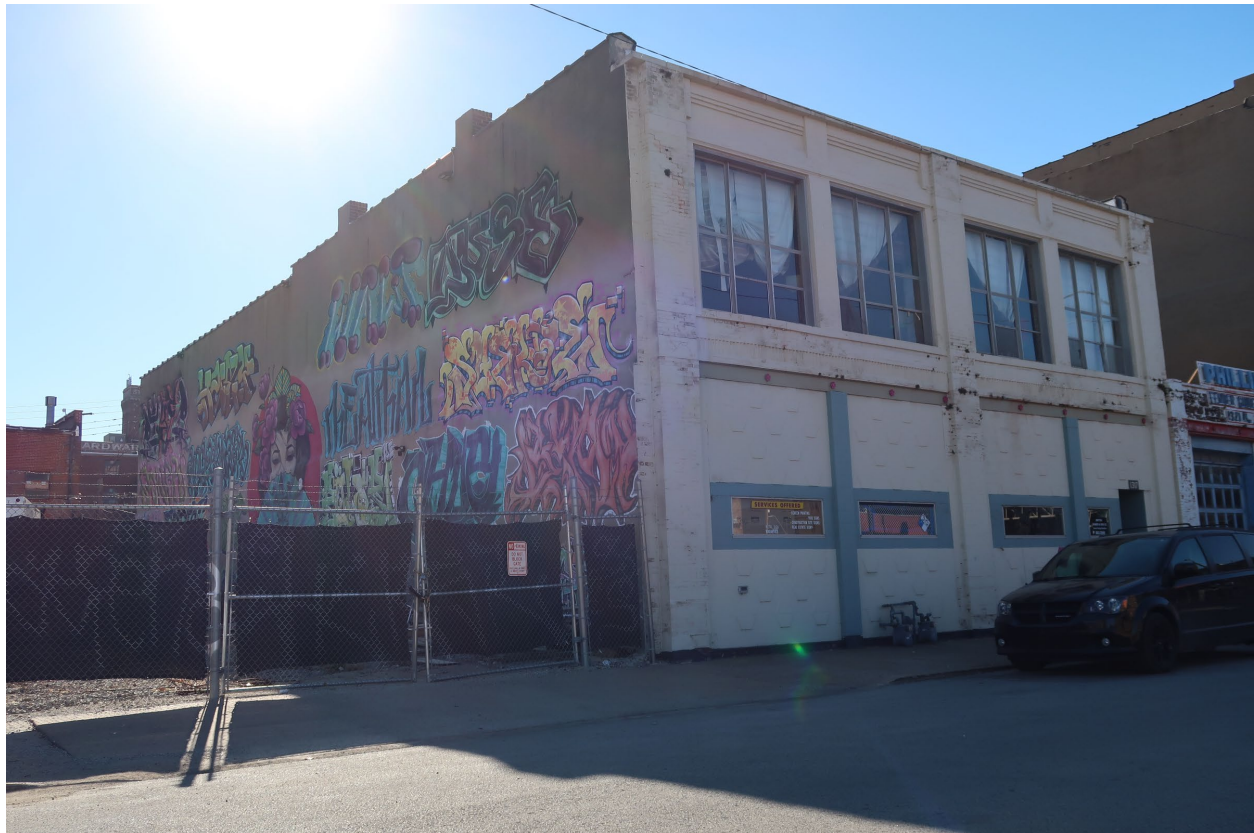
Looking Southwest At The Front (North) & East Elevations Of 1317 Union Ave. & Adjoining Storage Yard
