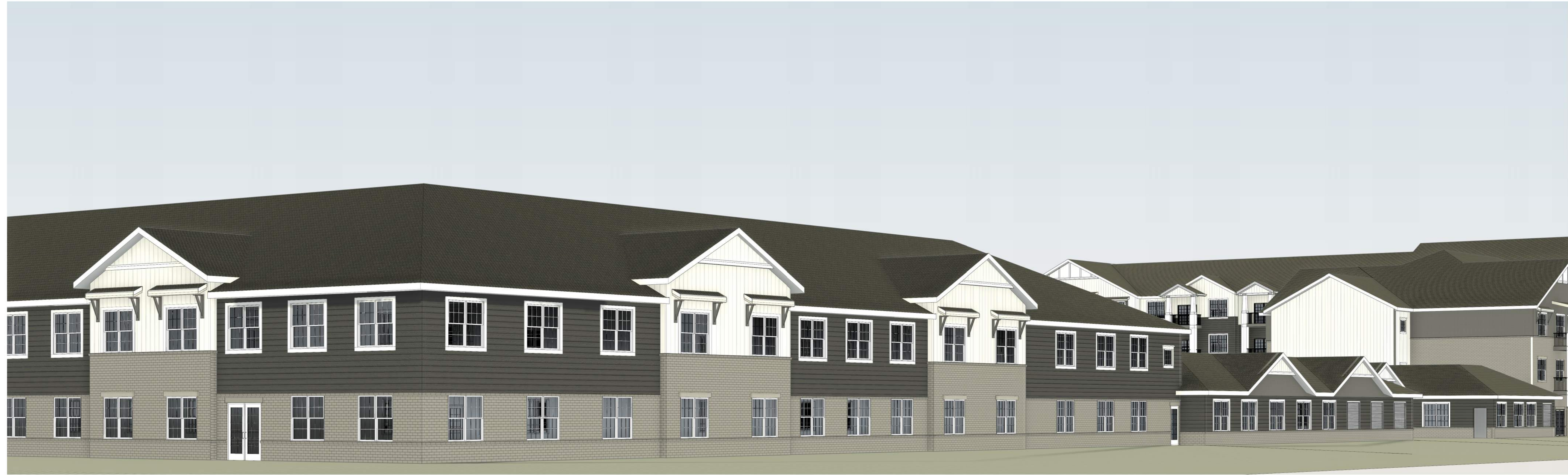
2 FROM BARRY RD LOOKING NORTHEAST
