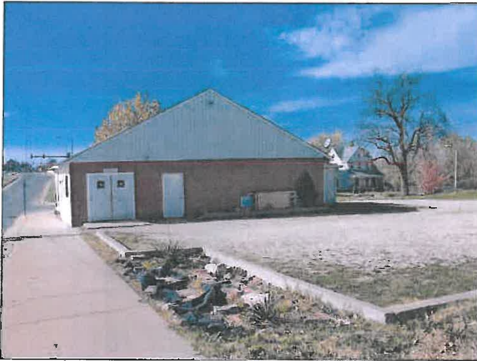
2108 E. 31 st Street – deterioration of parking surface
