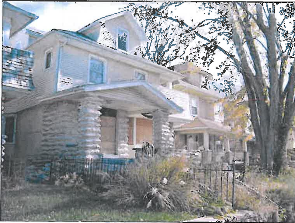
2805 Brooklyn Avenue – Inadequate lot size (narrow lot)
