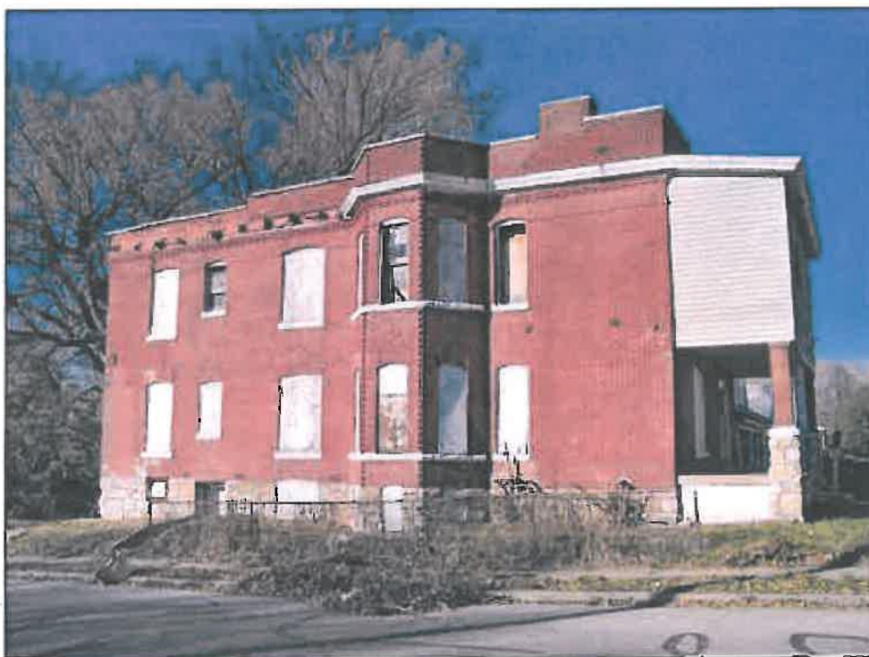
2944 Wabash Avenue – Deterioration of windows, walls, fence; trash/debris
