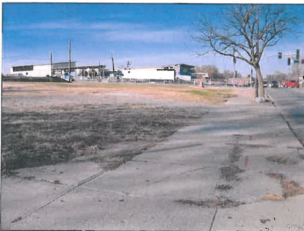
2700 block of Prospect Avenue – deterioration of parking surface; lack of landscaping; trash/debris
