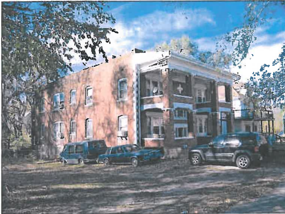
3016 Olive Street – inadequate lot size (unable to accommodate off-street parking for tenants)
