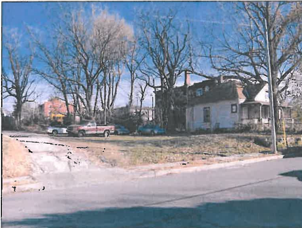
2935 Wabash Avenue – Improper parking surface; deterioration of driveway, parking surface
