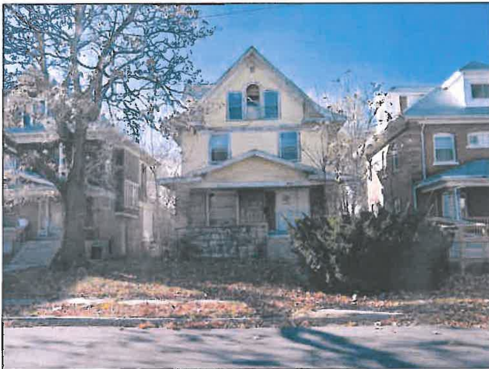
2920 Olive Street – Deterioration of roof, walls, doors, windows; failure of exterior finishes
