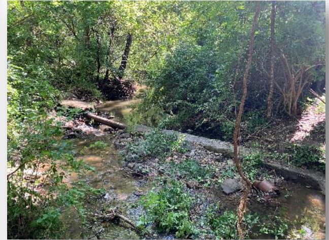
Site 41 - N039-100 / $173,000 estimated cost / temporary emergency repair already completed
