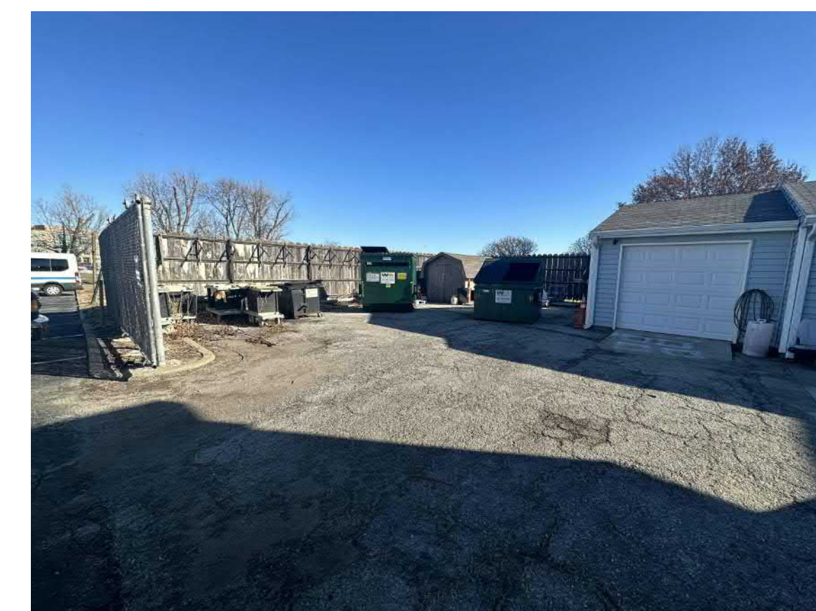
SERVICE AREA LOOKING NORTH WITH EXISTING WORKSHOP (RIGHT) AND ENCLOSING FENCE TO BE REWORK FOR NEW TOWER 'B'
