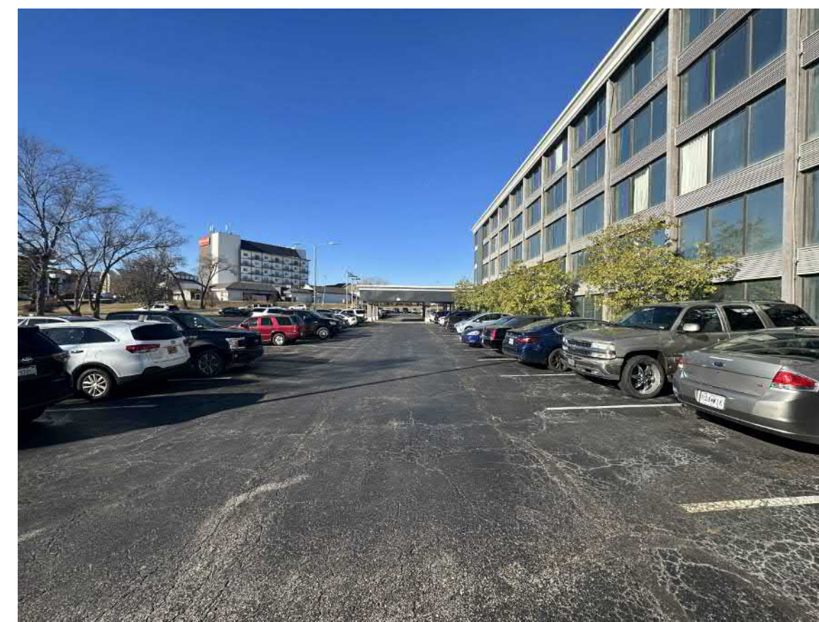
VIEW LOOKING WEST TOWARD PORT COCHERE IN THE DISTANCE AND SOUTH FACADE OF THE EXISTING GUEST TOWER 'A'
