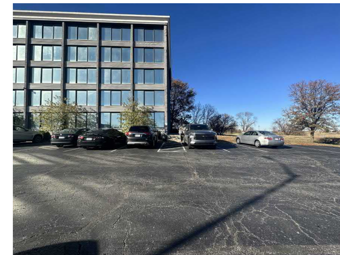
VIEW LOOKING EAST TOWARD GUEST TOWER 'A' (NORTH END) WITH EXISTING GREENSPACE WHERE NEW TOWER WILL CONNECT.
