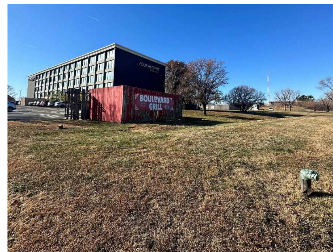
VIEW FROM NORTHEAST CORNER OF PROPERTY LOOKING TOWARD THE EXISTING TRASH ENCLOSURE (TO BE REMOVED FOR NEW REAR DRIVE LANE) AND EXISTING GREENSPACE WHERE NEW TOWER 'B' WILL BE LOCATED.
