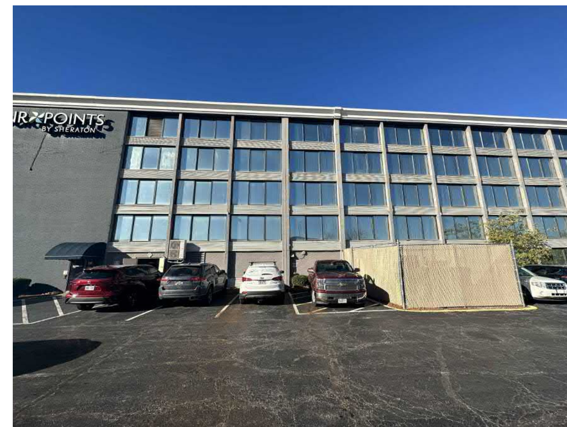
VIEW LOOKING EAST TOWARD GUEST TOWER 'A' WITH EXISTING BRANDING, CANOPY, AND SCREENING FENCE AROUND TRANSFORMER YARD.
