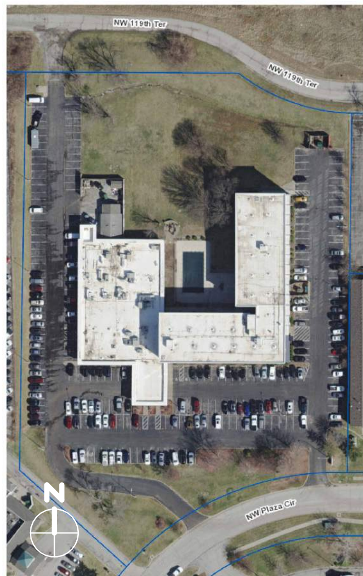
Existing Site View
