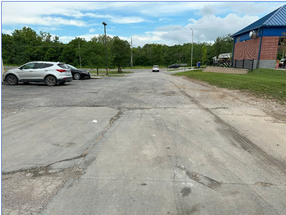
Looking west – deterioration of pavement; lack of curb/gutter along north edge of Study Area
