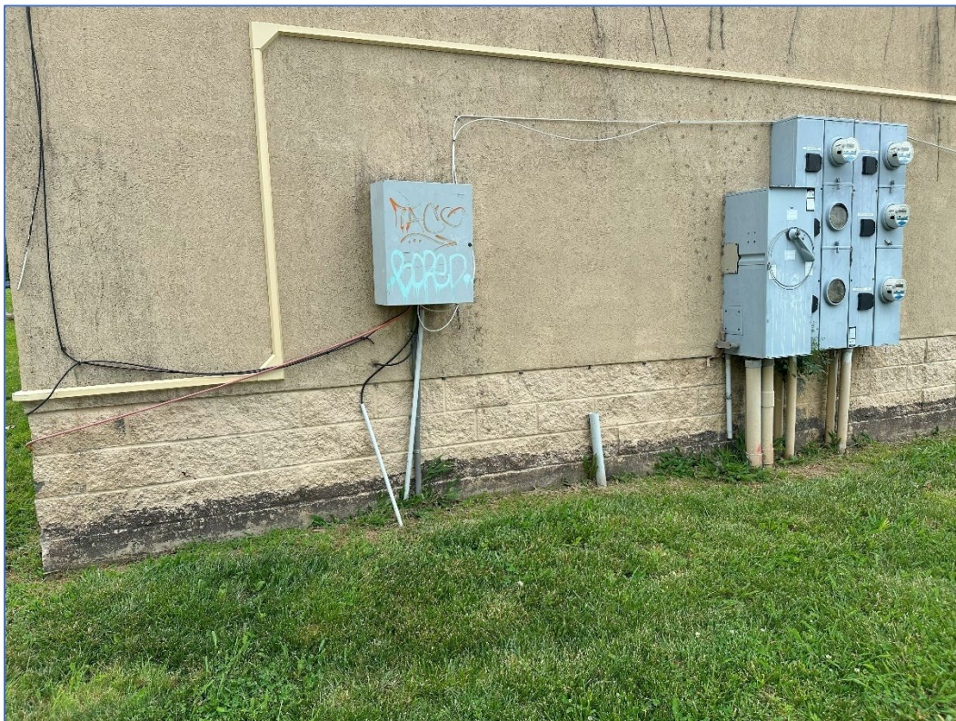
Looking west – graffiti; lines not in conduit
