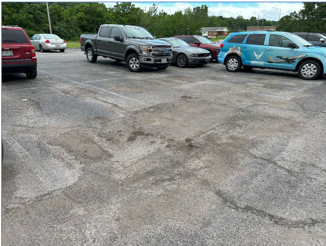
Looking northwest – deterioration of pavement
