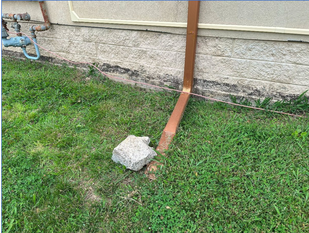
Looking north – poor drainage (blocked downspout)
