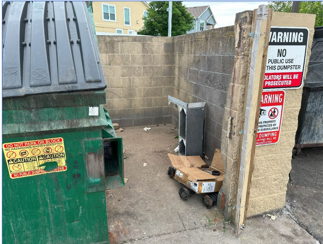
Looking east – deterioration of trash enclosure
