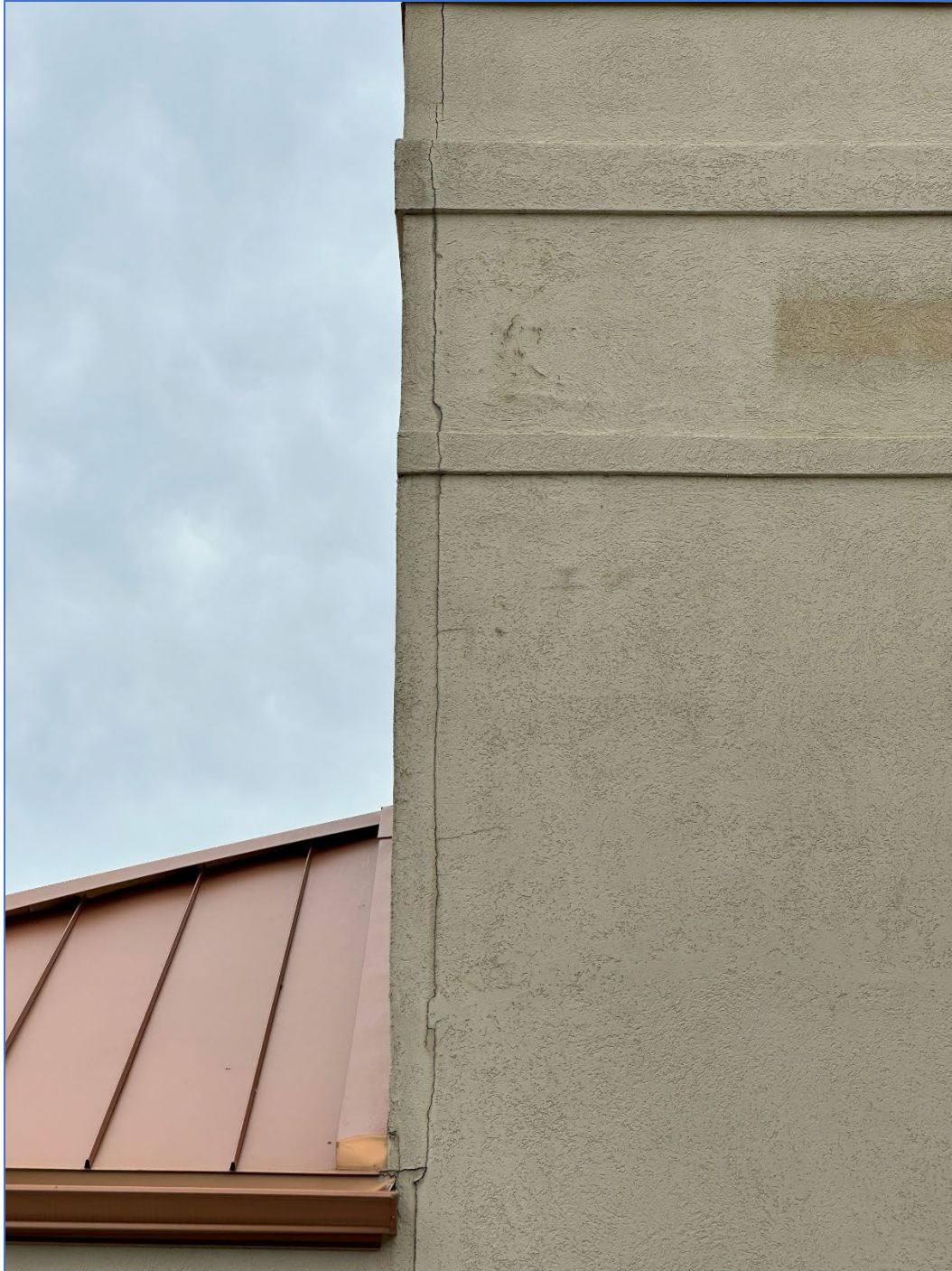
Looking east – cracking of EIFS
