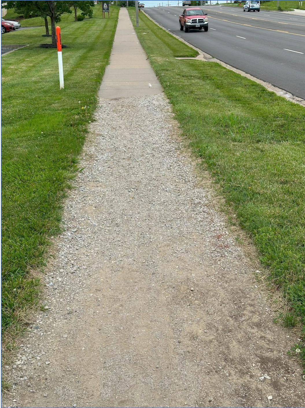
Looking south – deterioration of sidewalk (fall/trip hazard)
