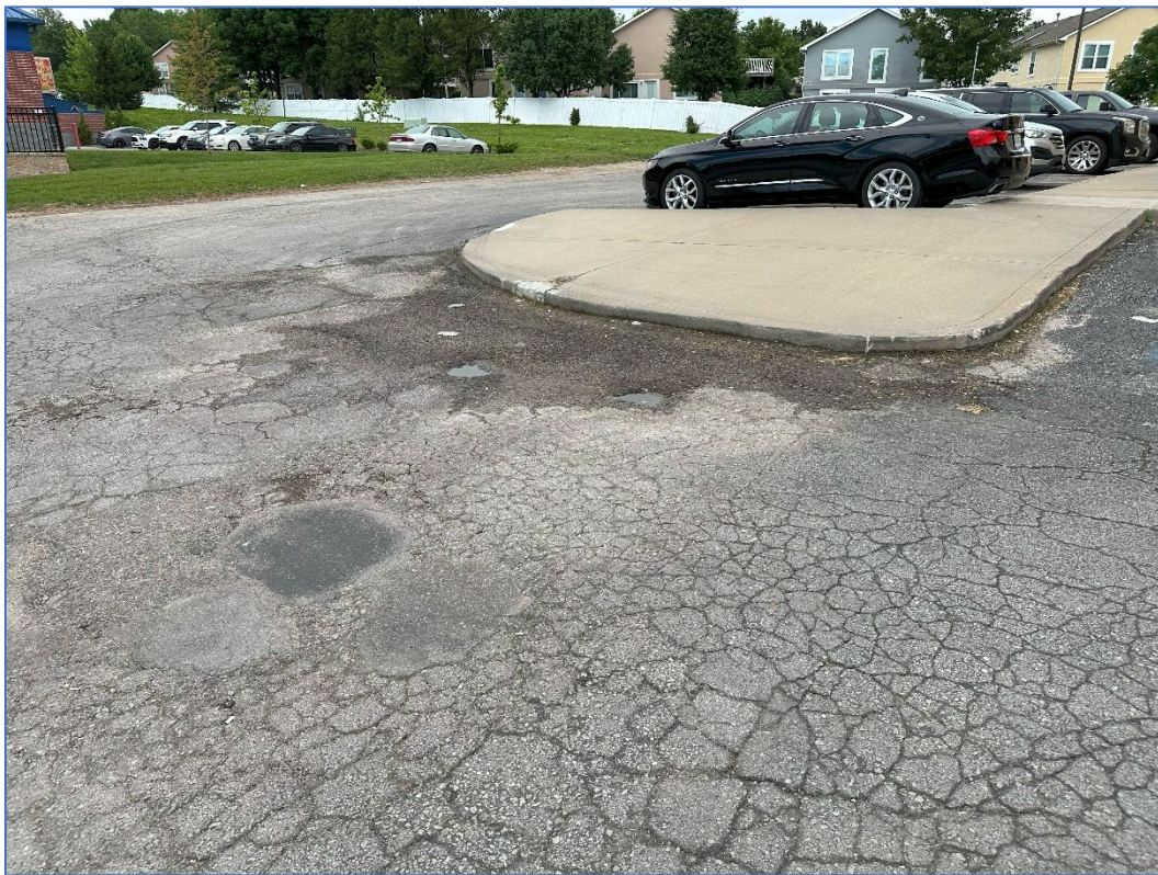
Looking northeast – deterioration of pavement
