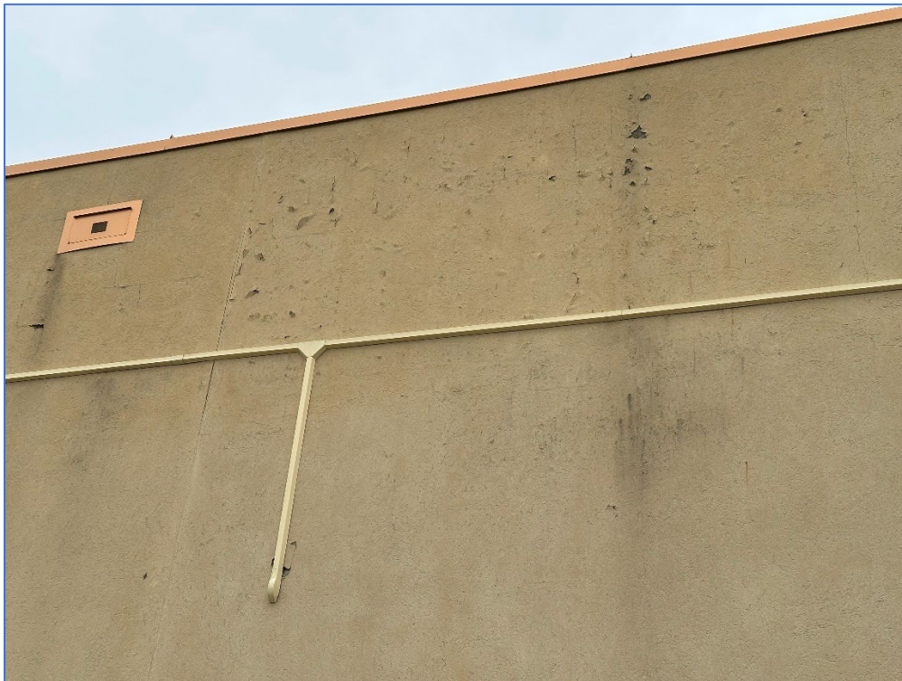
Looking west – failure of finishes
