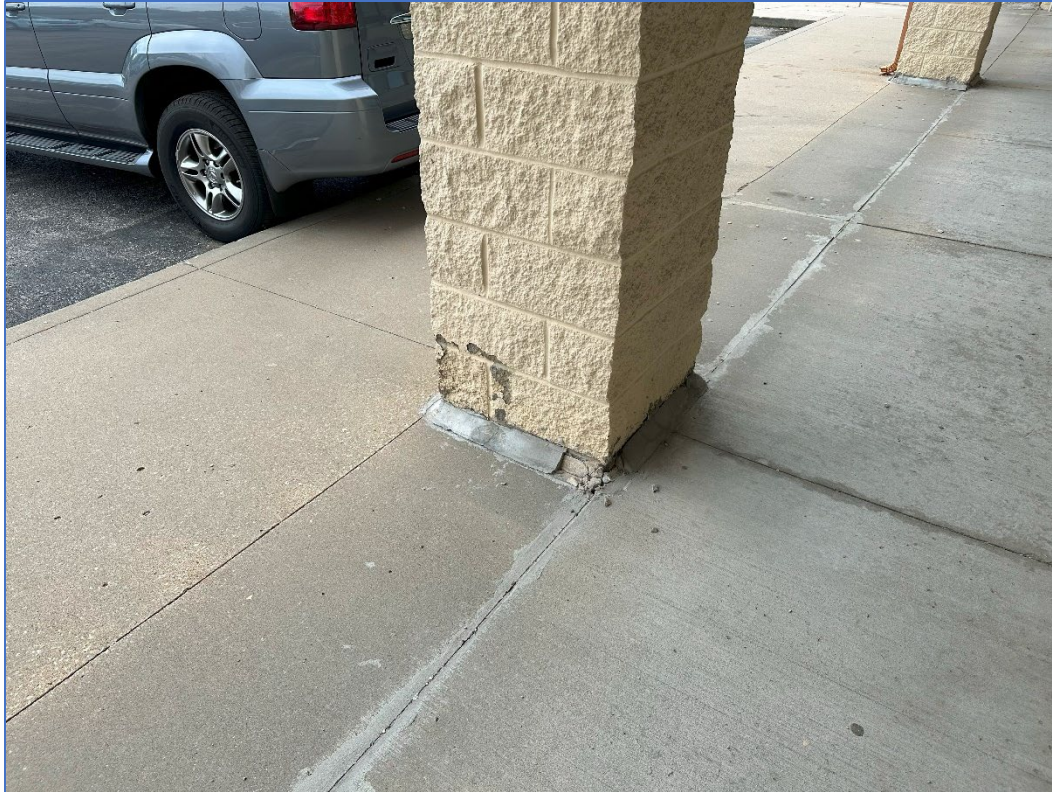
Looking south – deterioration of sealant at masonry/concrete joint
