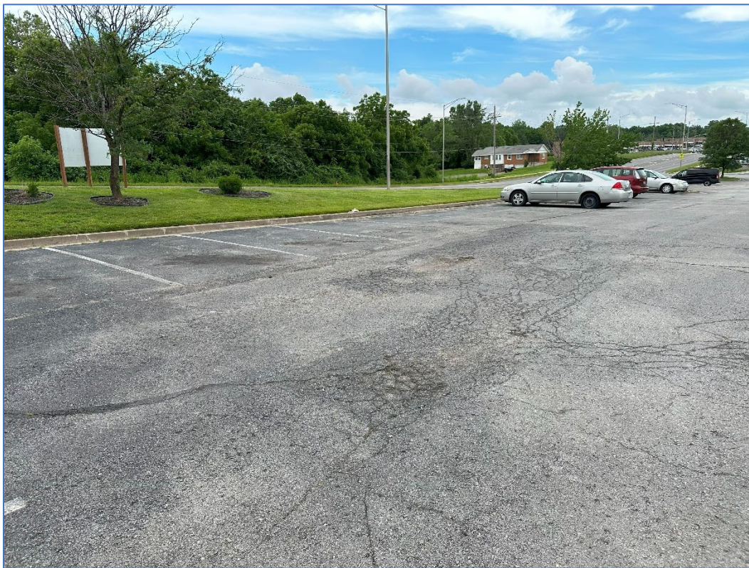
Looking northwest – deterioration of pavement
