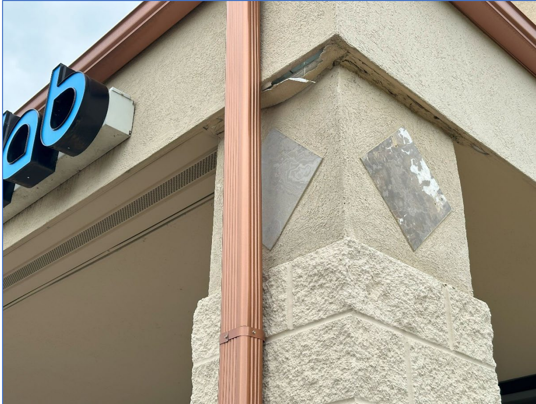
Looking southeast – deterioration of soffit
