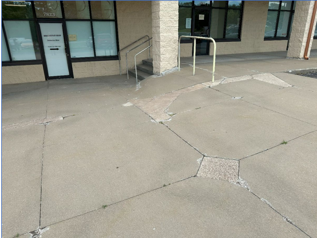
Looking east – uneven pavement (fall/trip hazard)
