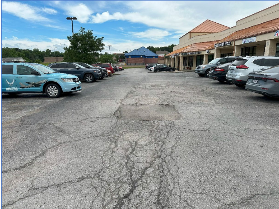
Looking north – deterioration of pavement
