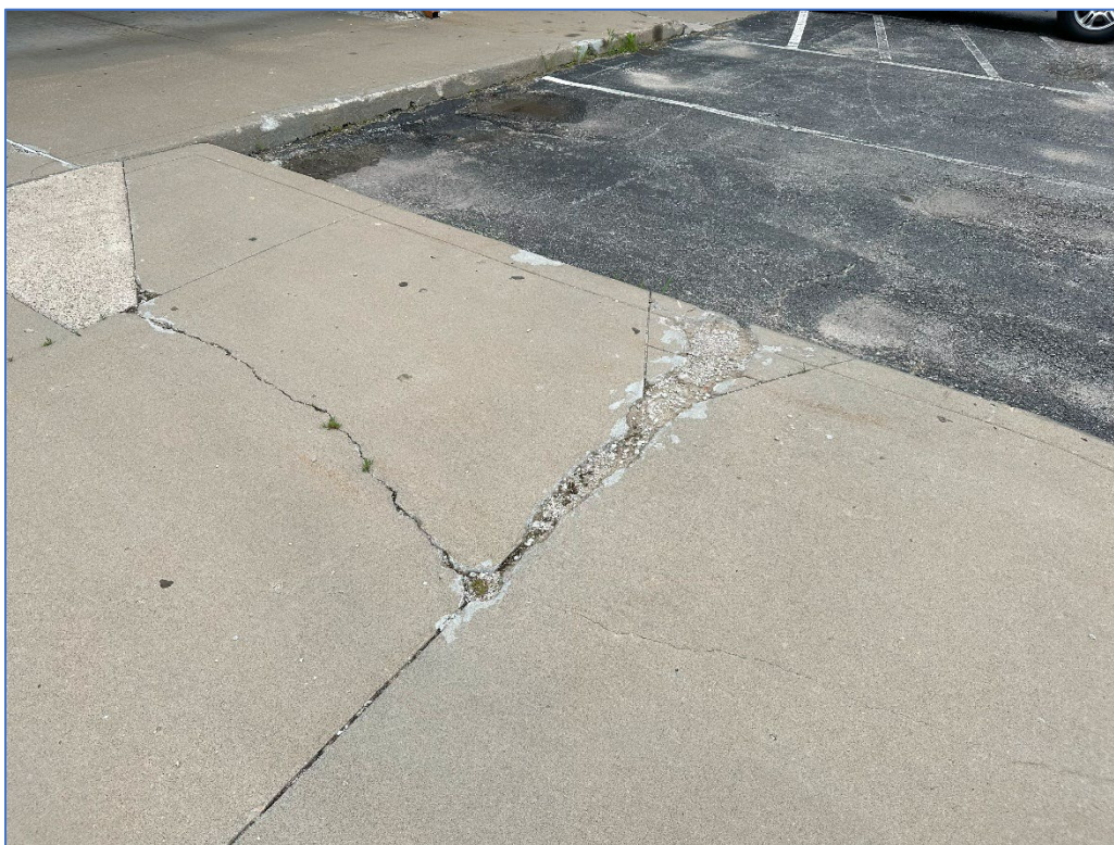
Looking south – cracked/uneven sidewalk (fall/trip hazard)
