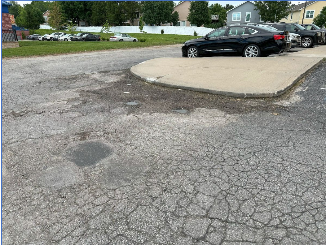
Looking northeast – deterioration of pavement (trip/fall hazard)
