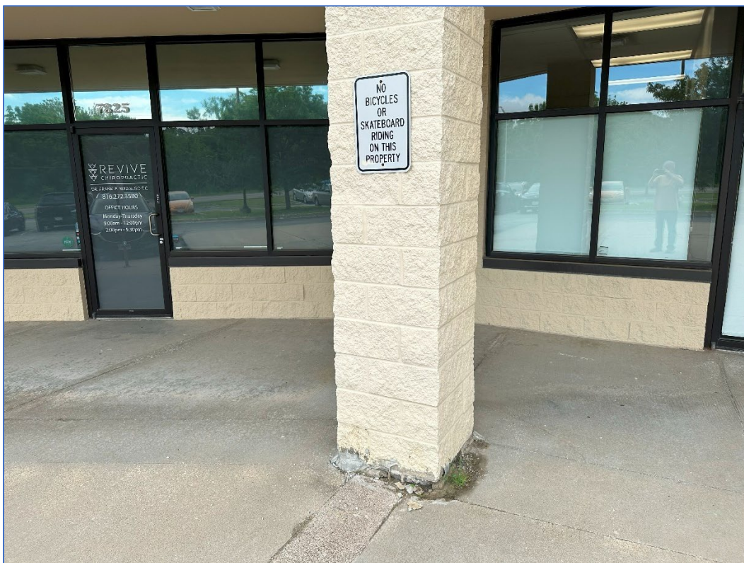
Looking east – deterioration of sealant at masonry/concrete joint
