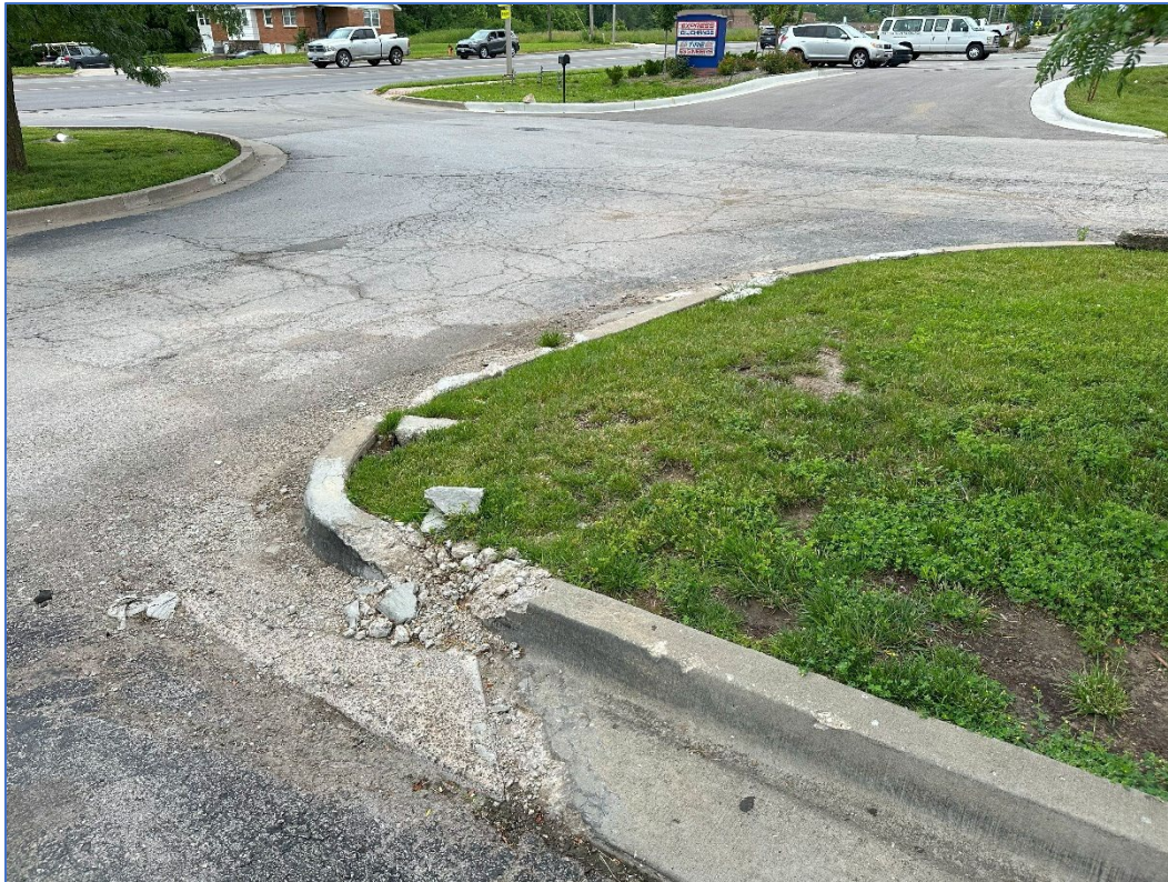
Looking northwest – deterioration of pavement and curb
