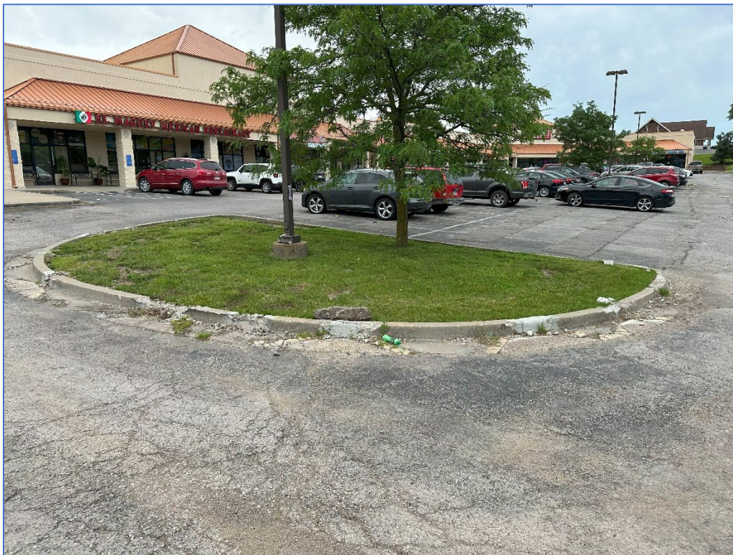
Looking southeast – deterioration of pavement and curb
