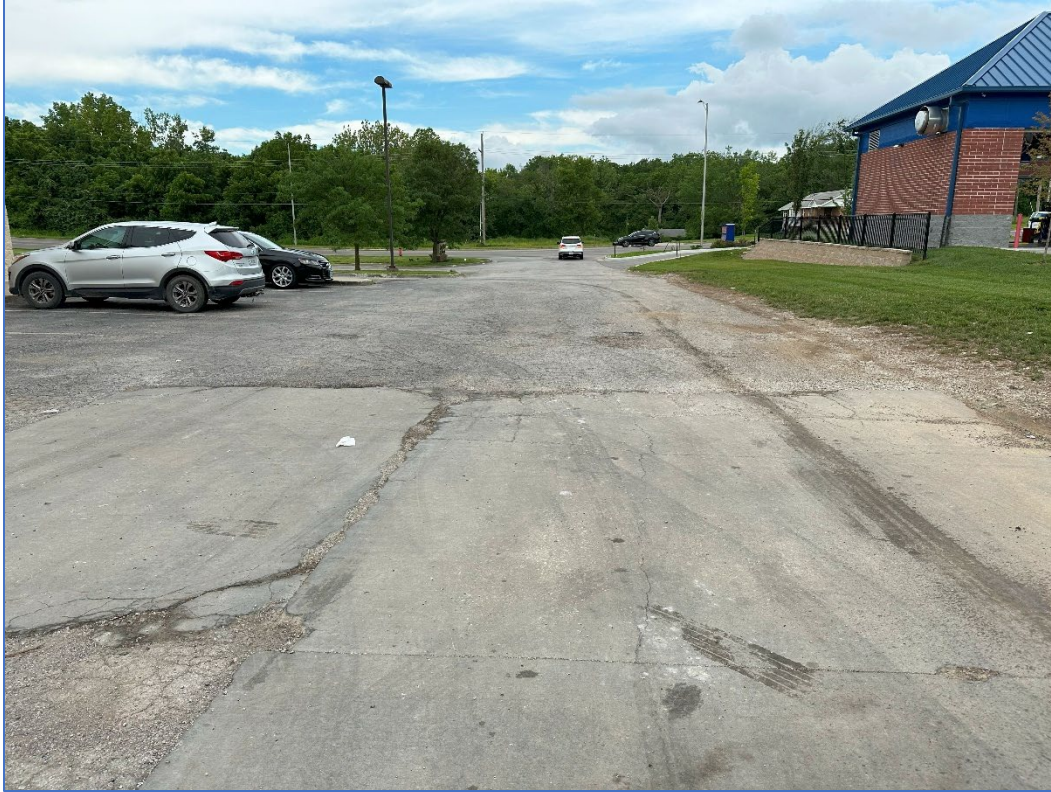
Looking west – deterioration of pavement, poor drainage (tripping/fall hazard)
