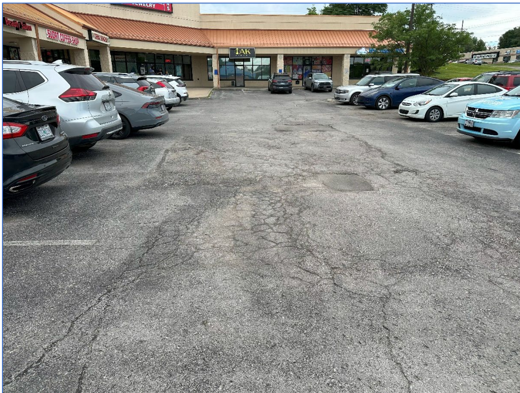
Looking south – deterioration of pavement (fall/trip hazard)
