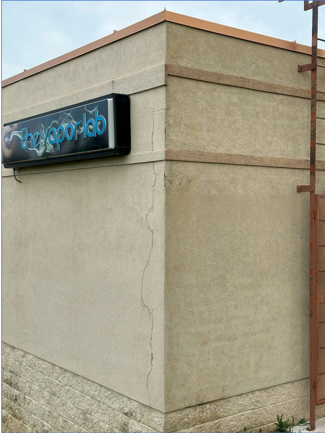
Looking northeast – cracking of EIFS
