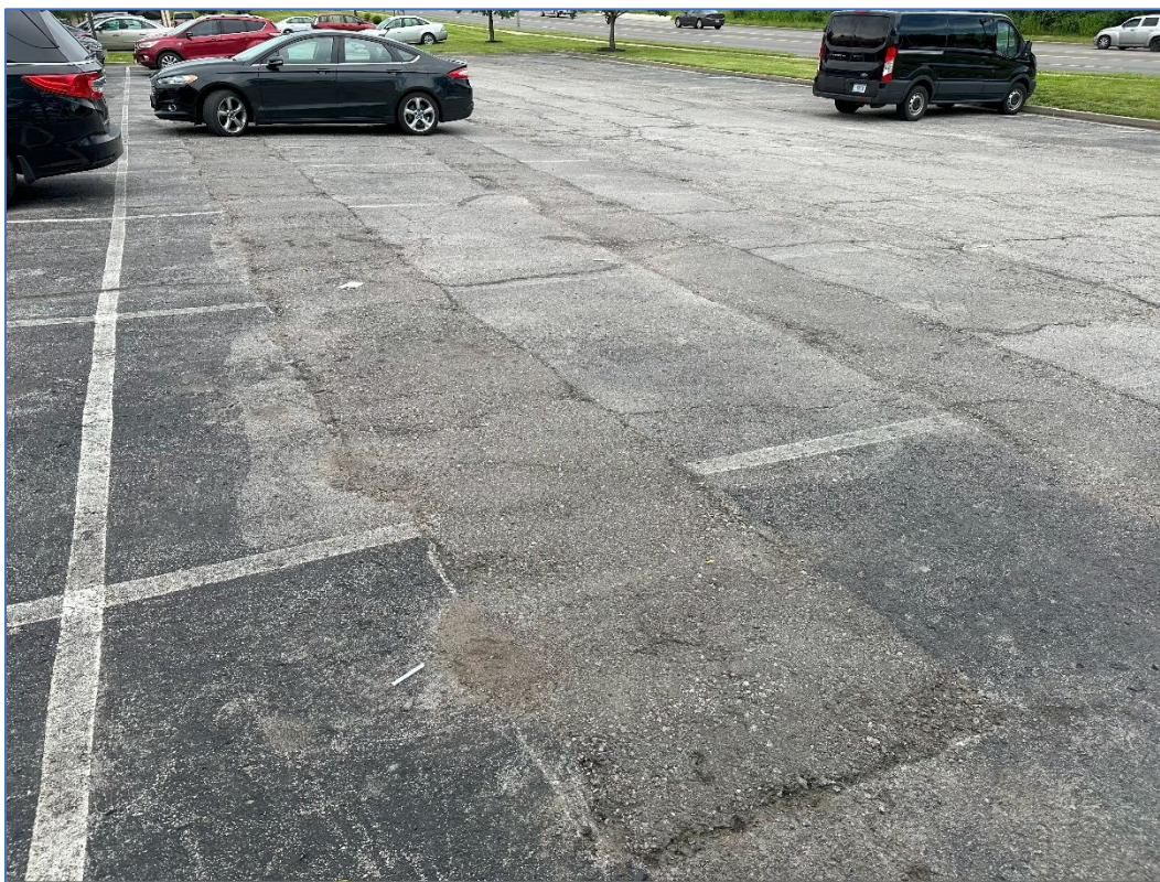
Looking southwest – deterioration of pavement
