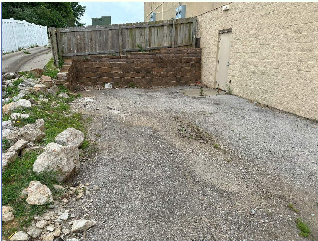
Looking south at end of service drive – deterioration pavement, drainage armor (trip/fall hazard)
