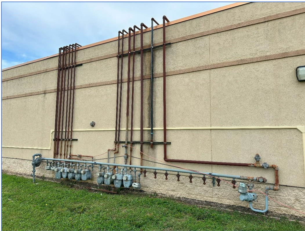
Looking north – rusting/corrosion of gas lines
