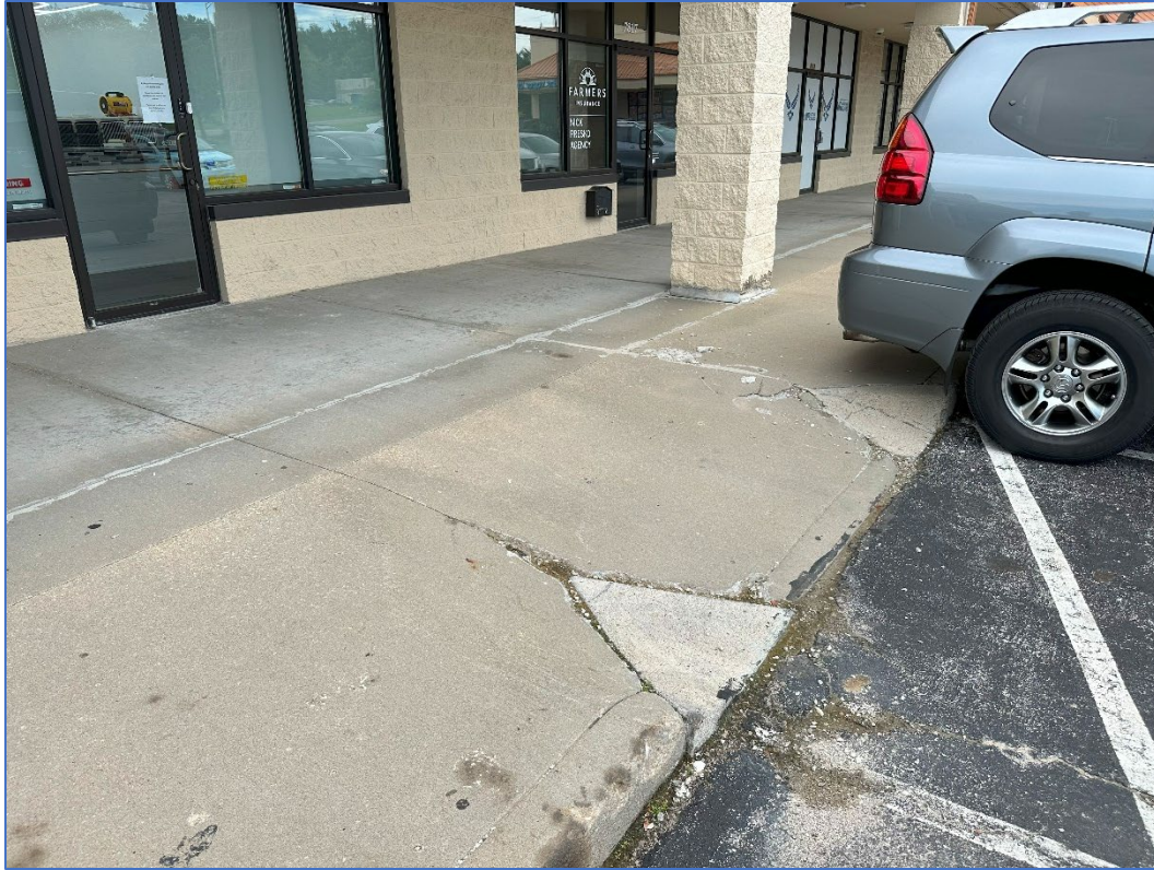
Looking southeast – uneven/deteriorated sidewalk (fall/trip hazard)
