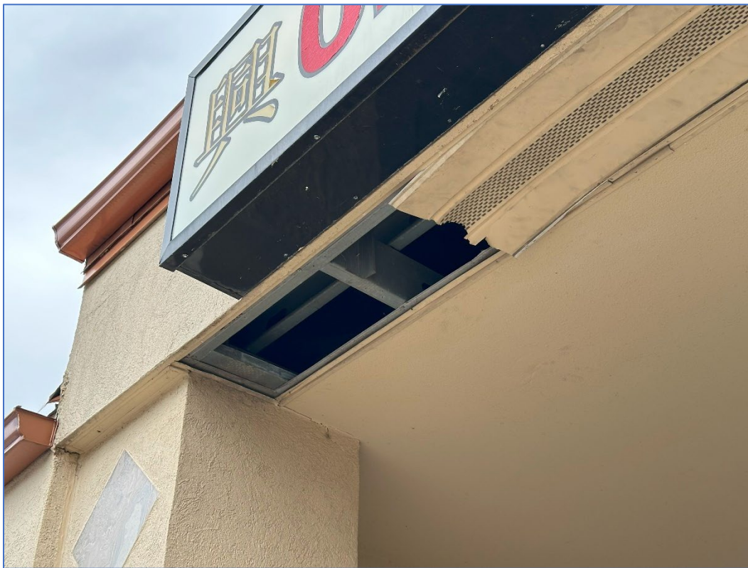
Looking east – deterioration of soffit
