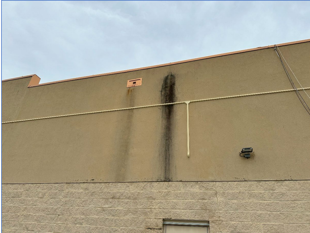
Looking west – water damage at parapet; failure of finishes
