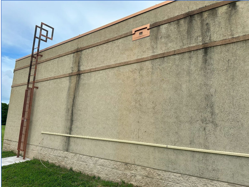
Looking northwest – rusting of ladder/enclosure; water damage to EIFS; failure of finishes
