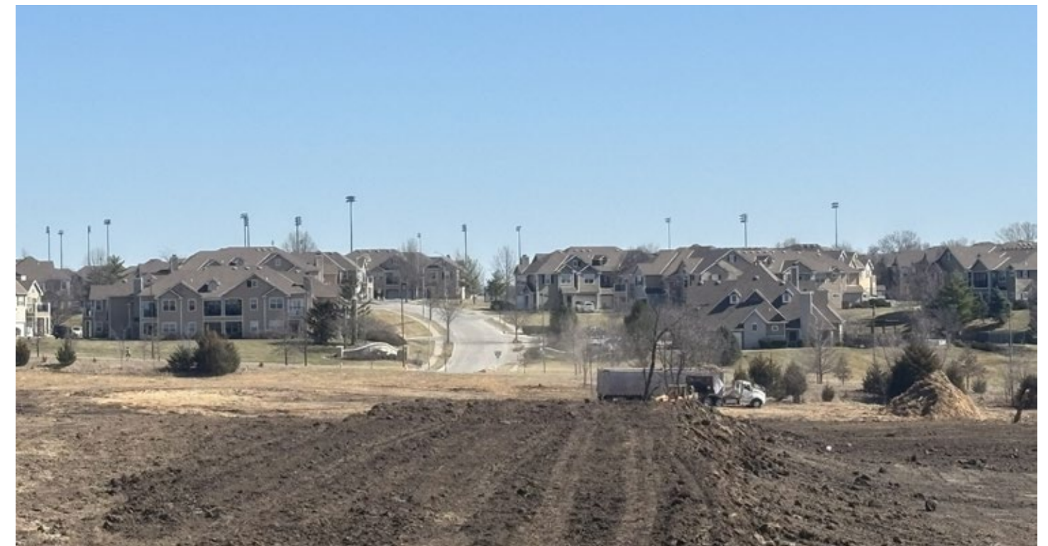
A new residential subdivision under construction, January 2026.
