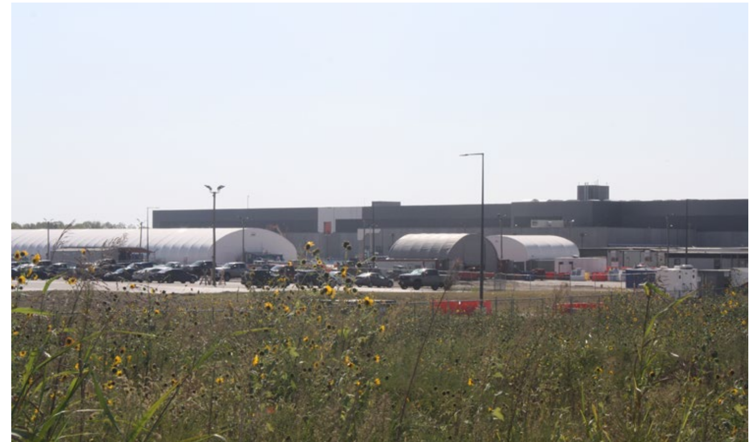
Meta Data Center located at 1800 NW 128 th Street. October 2025.
