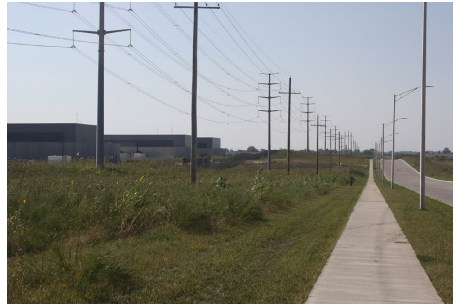
Newly constructed sidewalk in KCI Area, October 2025.
