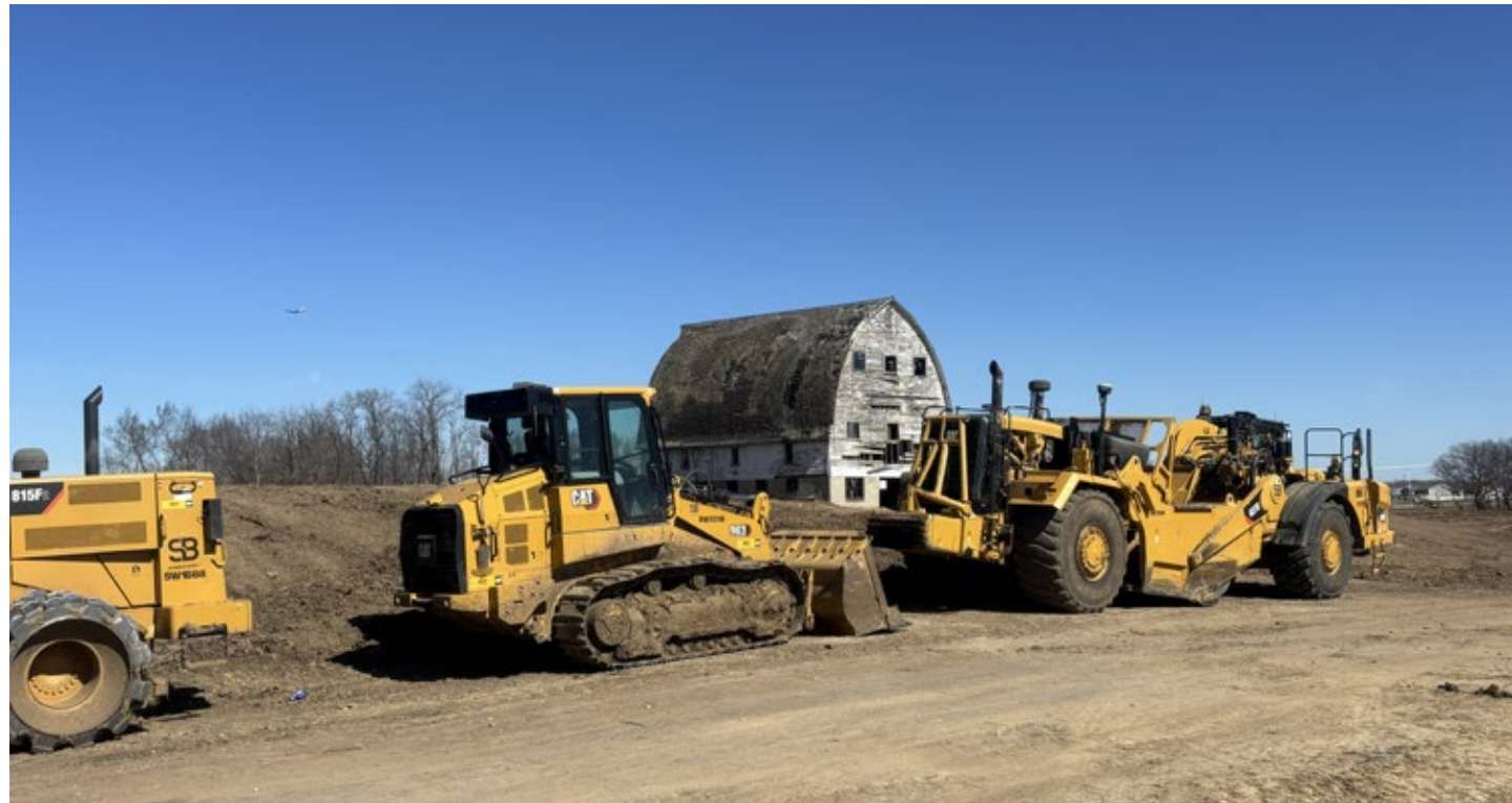
Grading land for new subdivision, January 2026.
