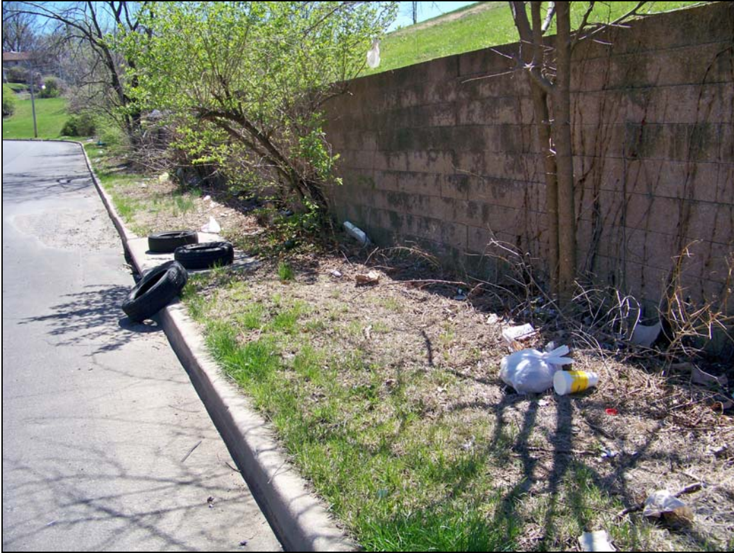
4900 block of Montgall Avenue – illegal dumping; trash/debris
