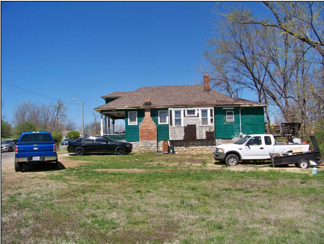
4900 block of Montgall Avenue – vehicles parked in yard
