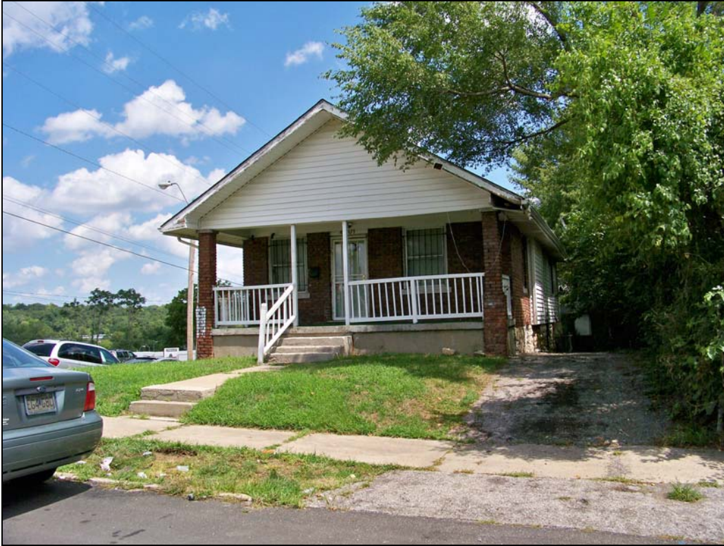
4900 block of Montgall Avenue – deterioration of driveway, fence
