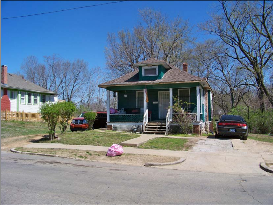
4900 block of Montgall Avenue – deterioration of driveways
