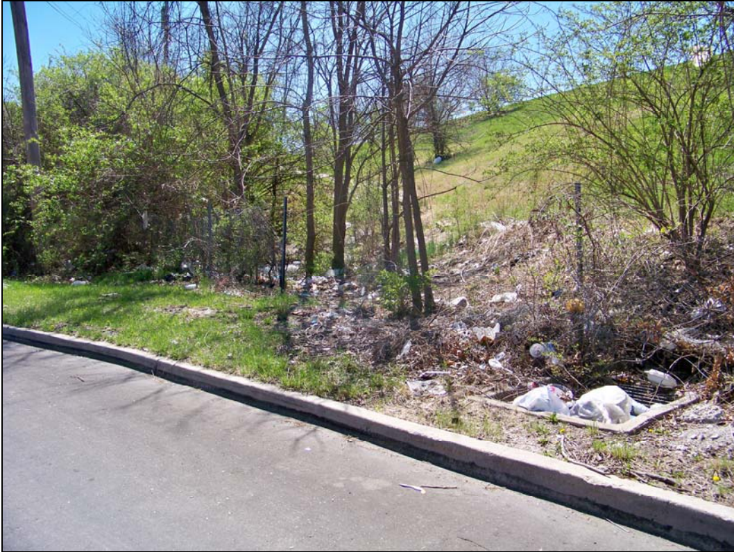
4900 block of Montgall Avenue –trash/debris; overgrown vegetation; graffiti; deterioration of fence
