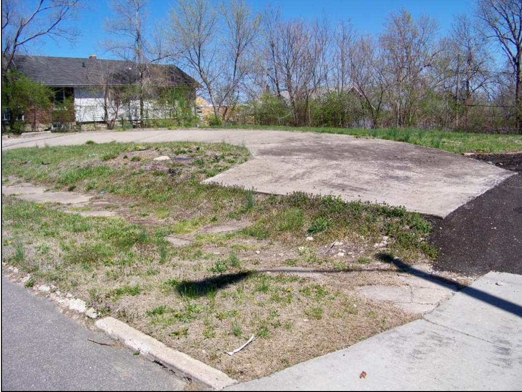
4900 block of Montgall Avenue – deterioration of sidewalk
