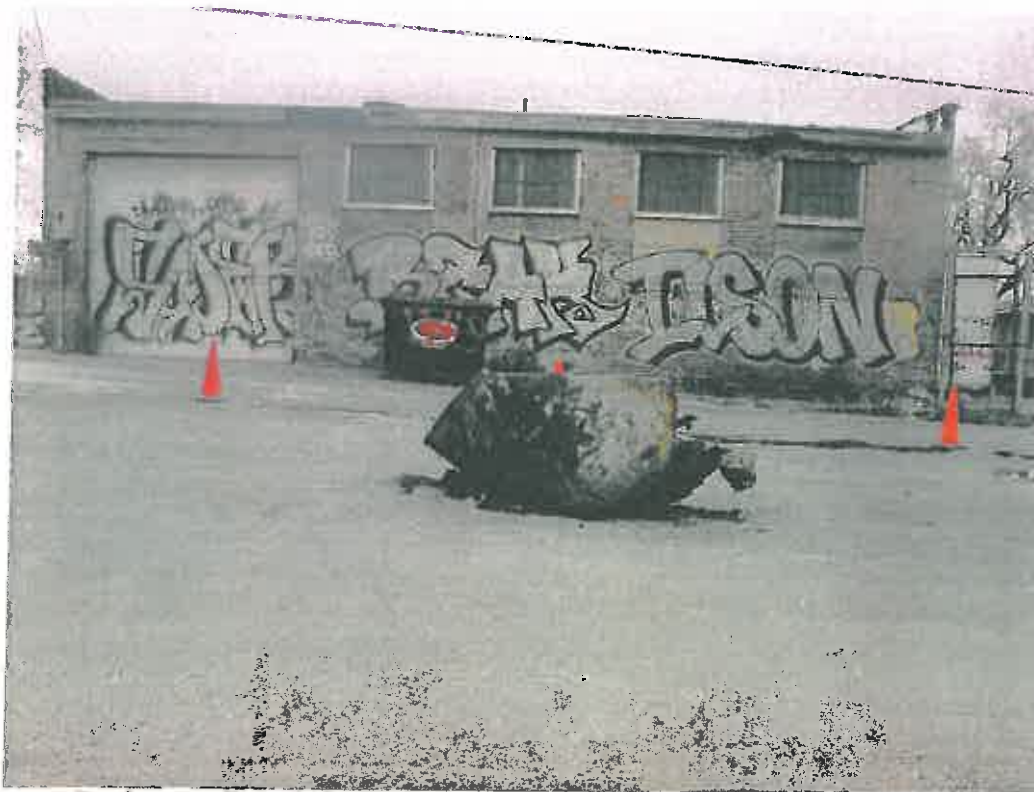
Significant graffiti and what appears to be scrape metal debris (1600 block Locust St.)
