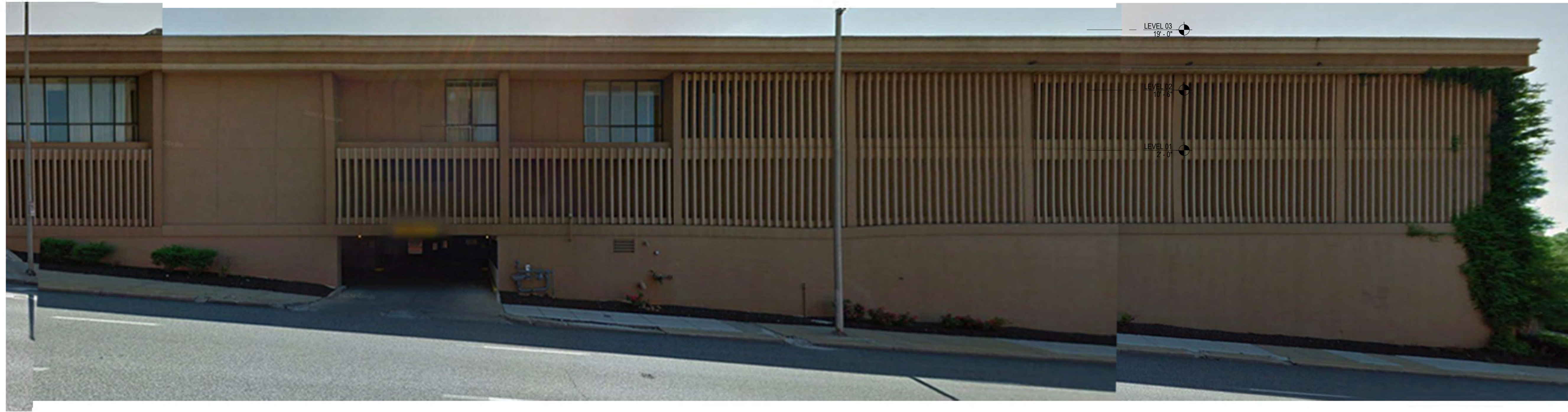
WEST ELEVATION / GUESTROOM TOWER DEMOLITION
