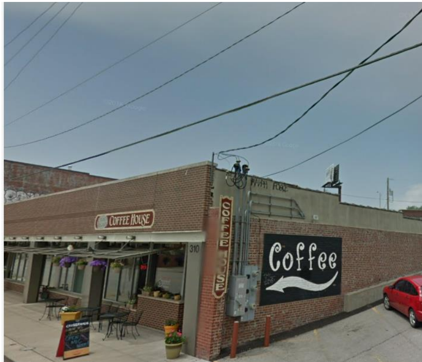
Project 17 – Sierra Building
