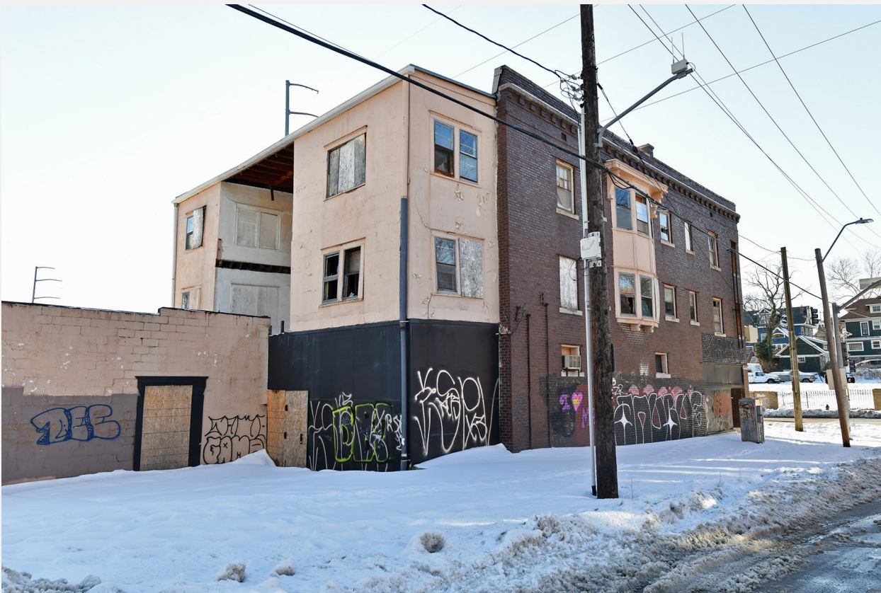
View from 43 rd St (North)
