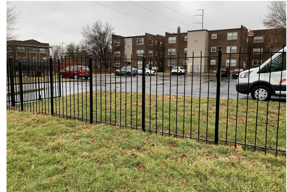
4' OR 6' TALL ANTI-CLIMB, ORNAMENTAL BLACK METAL FENCE EXAMPLE REF: PLAN FOR HEIGHT
