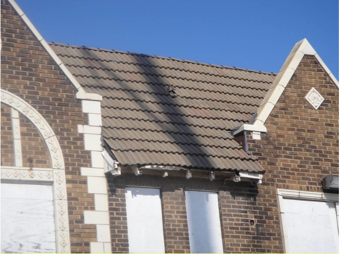
Photo 5 – View of the parapet detail along the eastern façade of the subject building.
