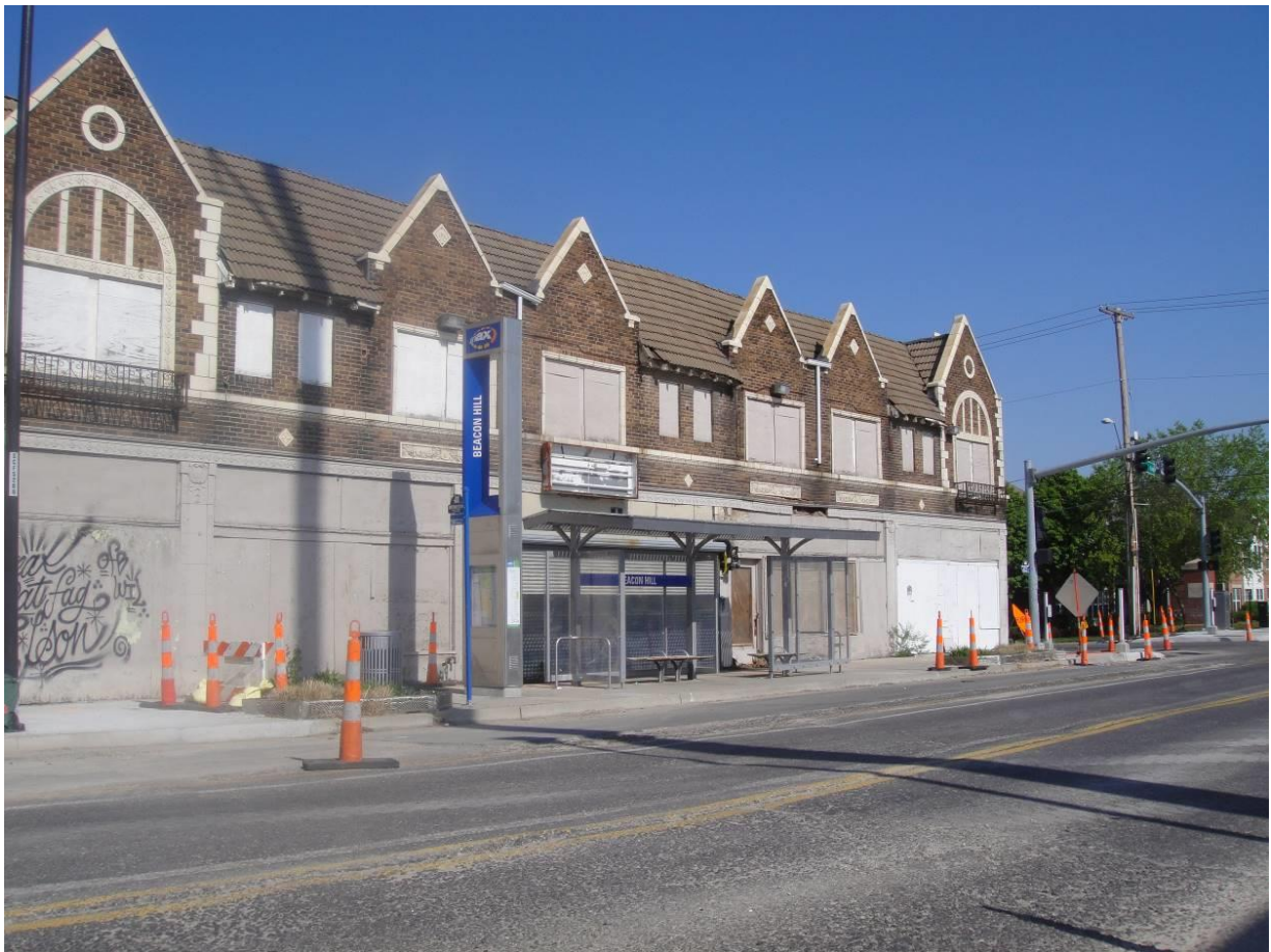
Photo 2 - Photo indicates facility entirely vacant.
