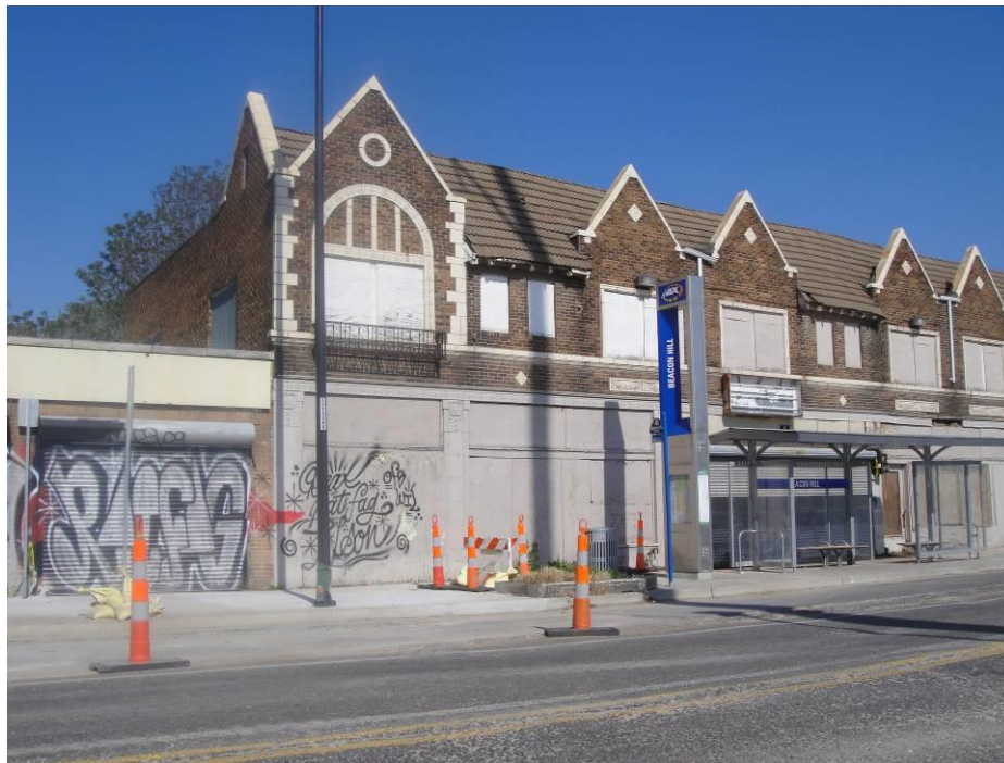
Photo 7 – View of the eastern façade of the subject building. Note graffiti present. The presence of graffiti continues the perception of a underutilized and vacant facility and can cause a economic and social liability to the surrounding neighborhood.
