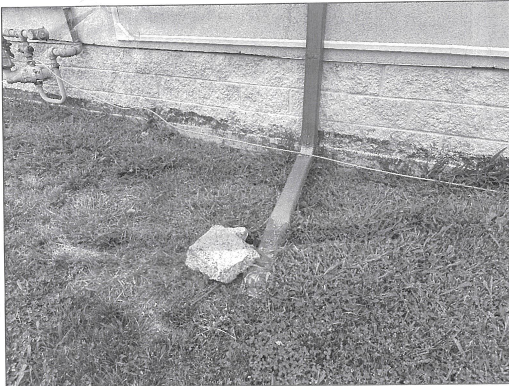
Looking north – poor drainage (blocked downspout)
