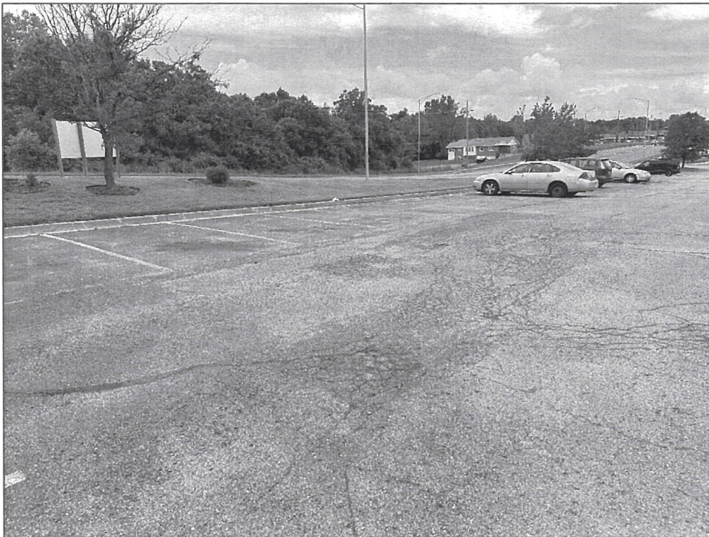
Looking northwest – deterioration of pavement
