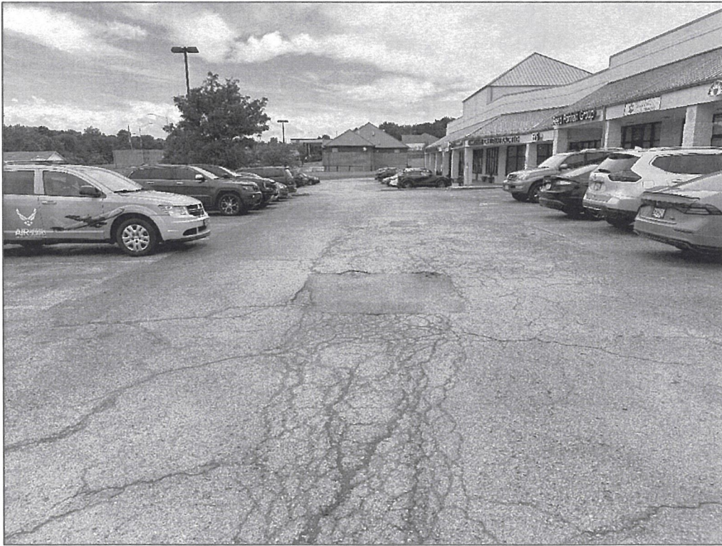
Looking north – deterioration of pavement
