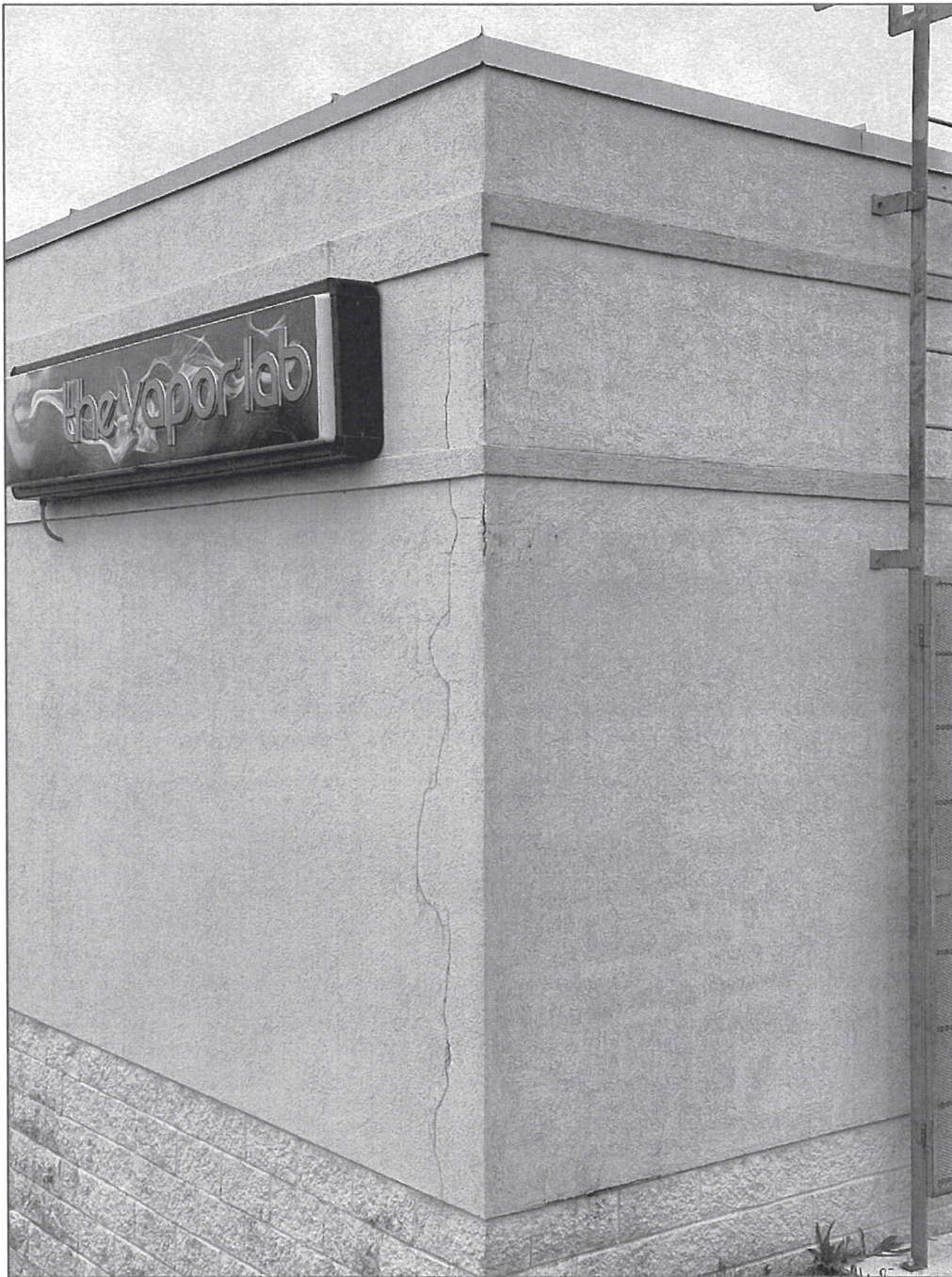
Looking northeast – cracking of EIFS
