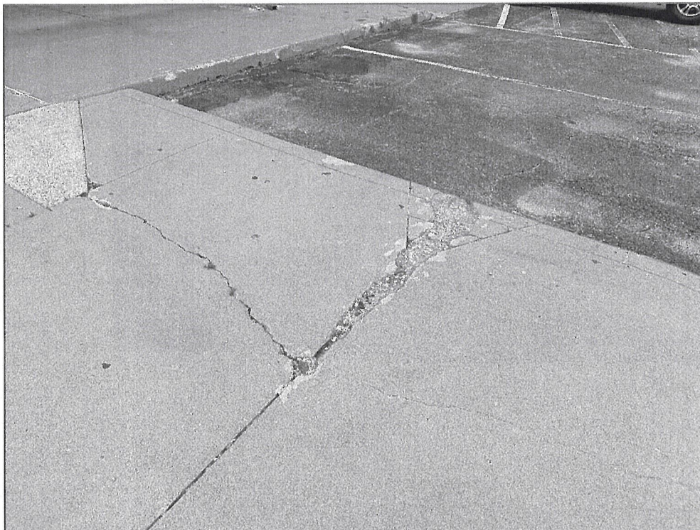
Looking south – cracked/uneven sidewalk (fall/trip hazard)
