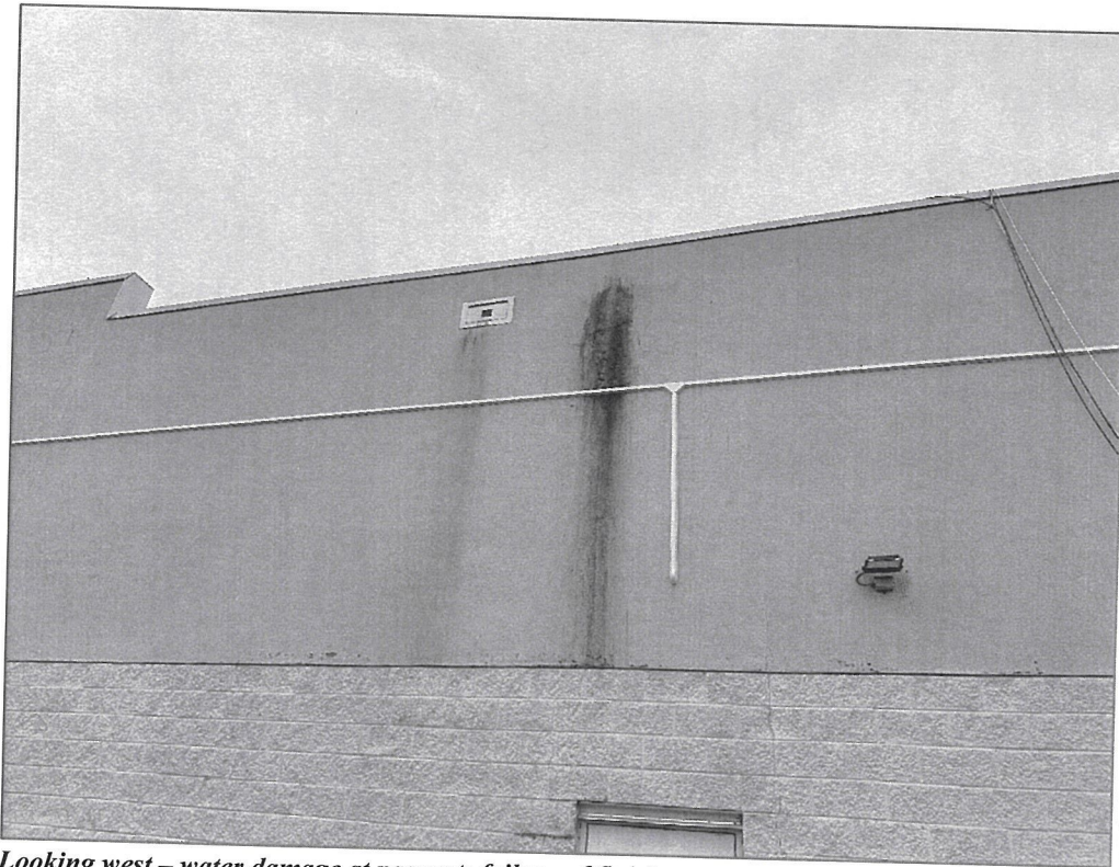
Looking west – water damage at parapet; failure of finishes
