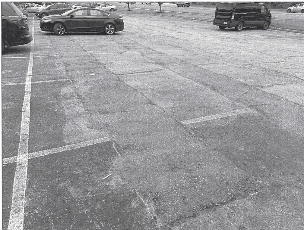
Looking southwest – deterioration of pavement
