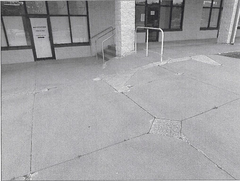
Looking east – uneven pavement (fall/trip hazard)
