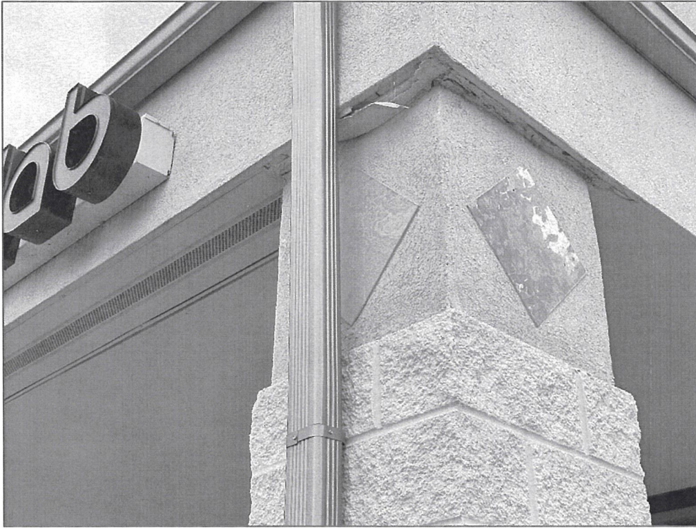
Looking southeast – deterioration of soffit
