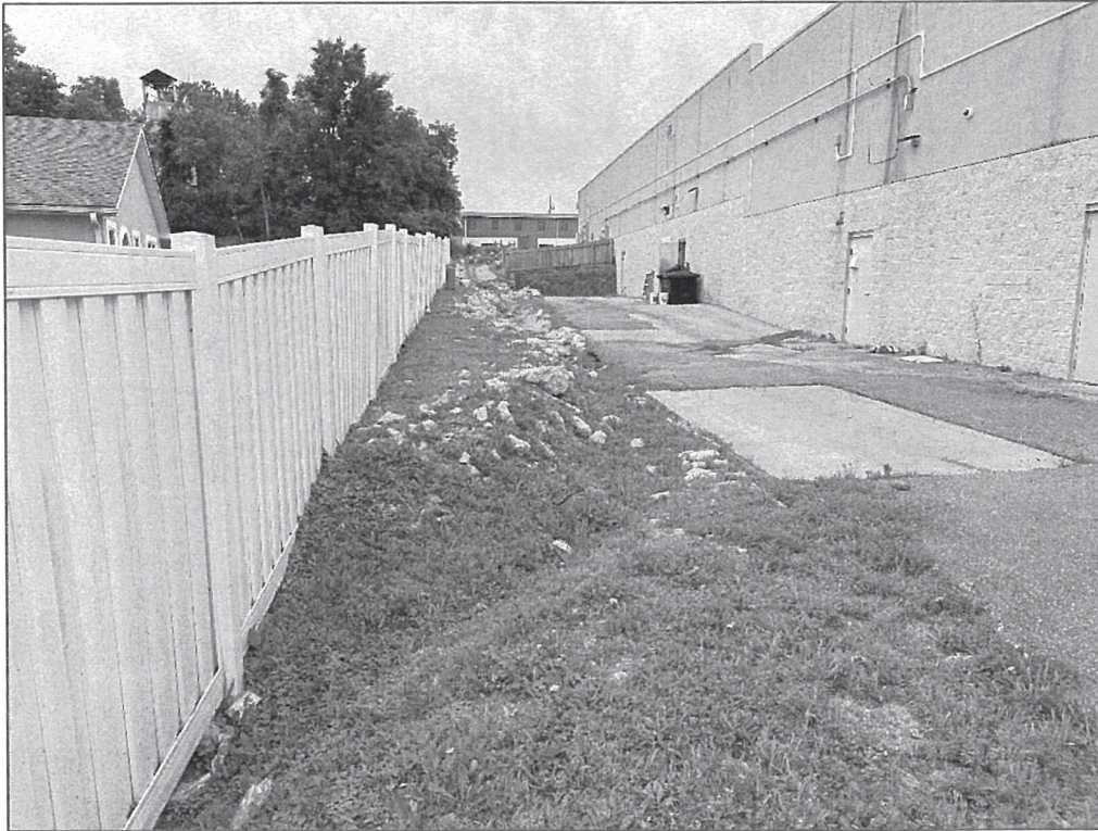
Looking south at service drive – poor drainage; uneven pavement (trip/fall hazard)
