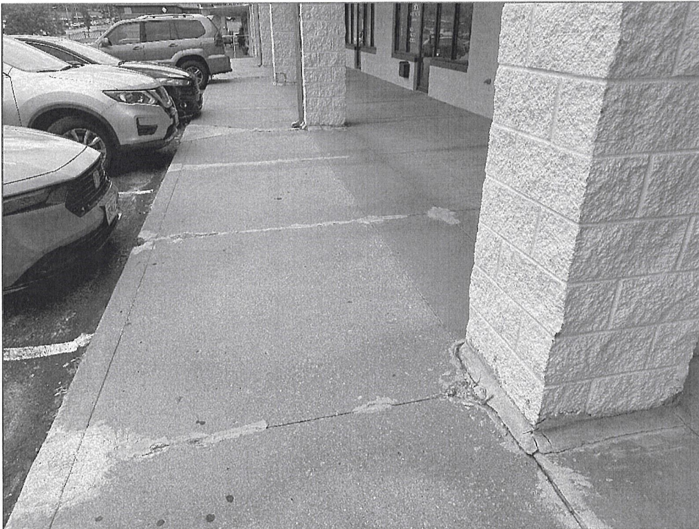
Looking north – poor drainage across sidewalk, uneven pavement
