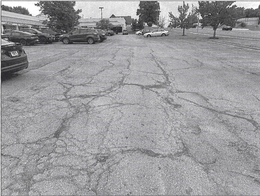
Looking south – deterioration of pavement
