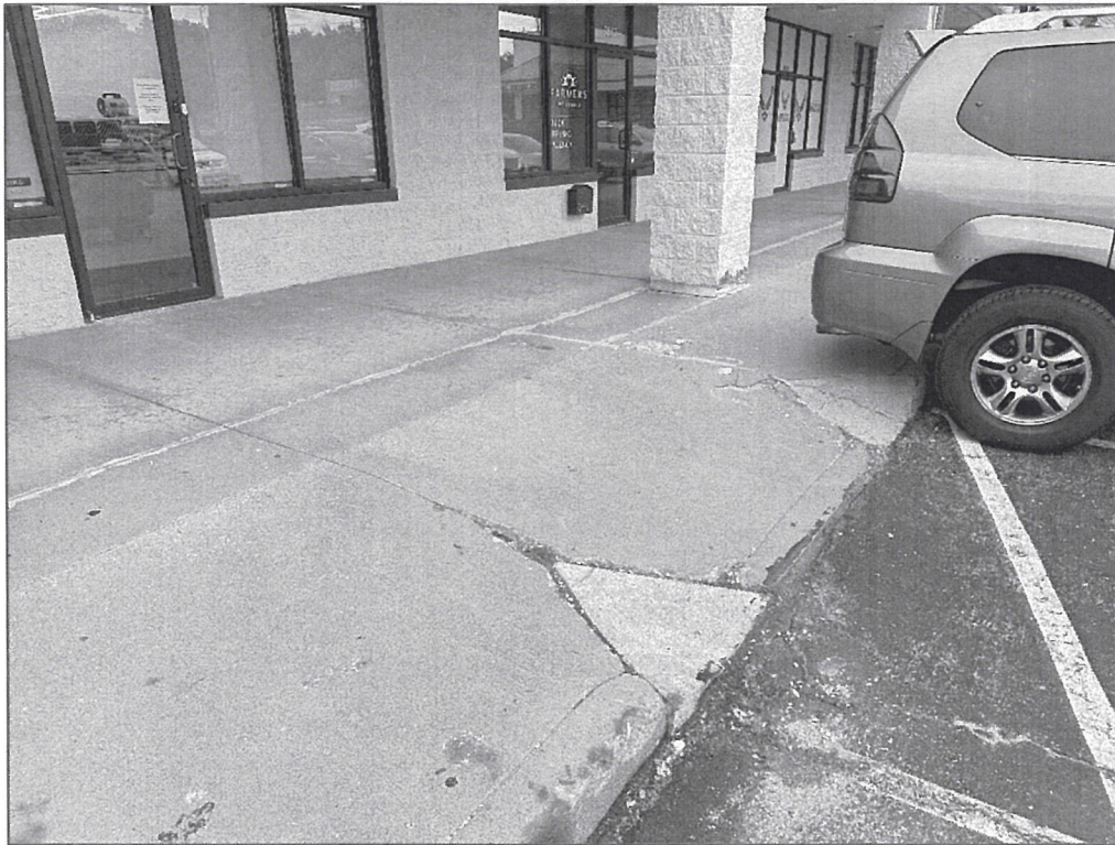
Looking southeast – uneven/deteriorated sidewalk (fall/trip hazard)
