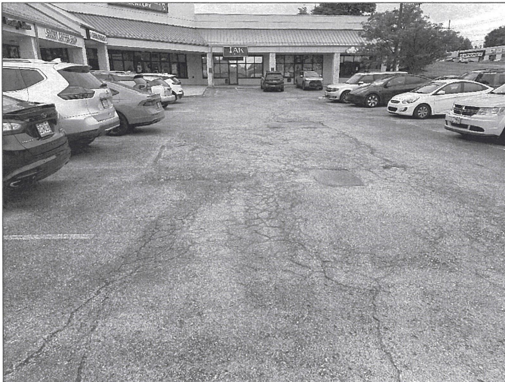
Looking south – deterioration of pavement (fall/trip hazard)
