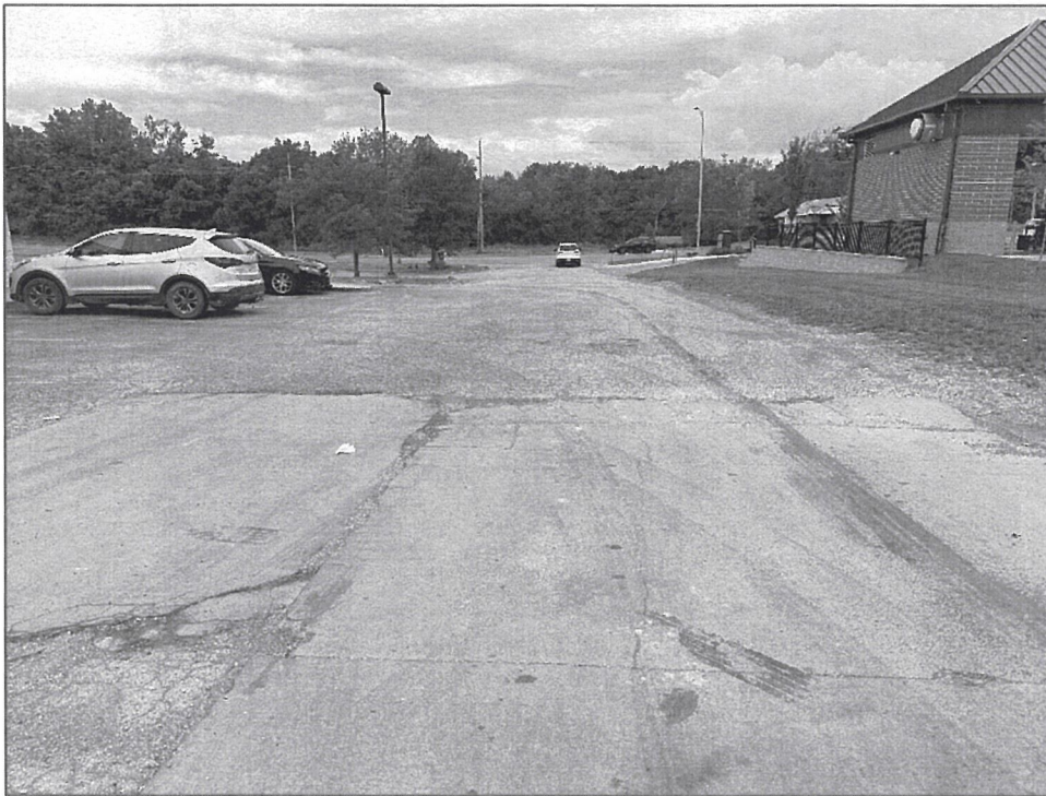
Looking west – deterioration of pavement; lack of curb/gutter along north edge of Study Area
