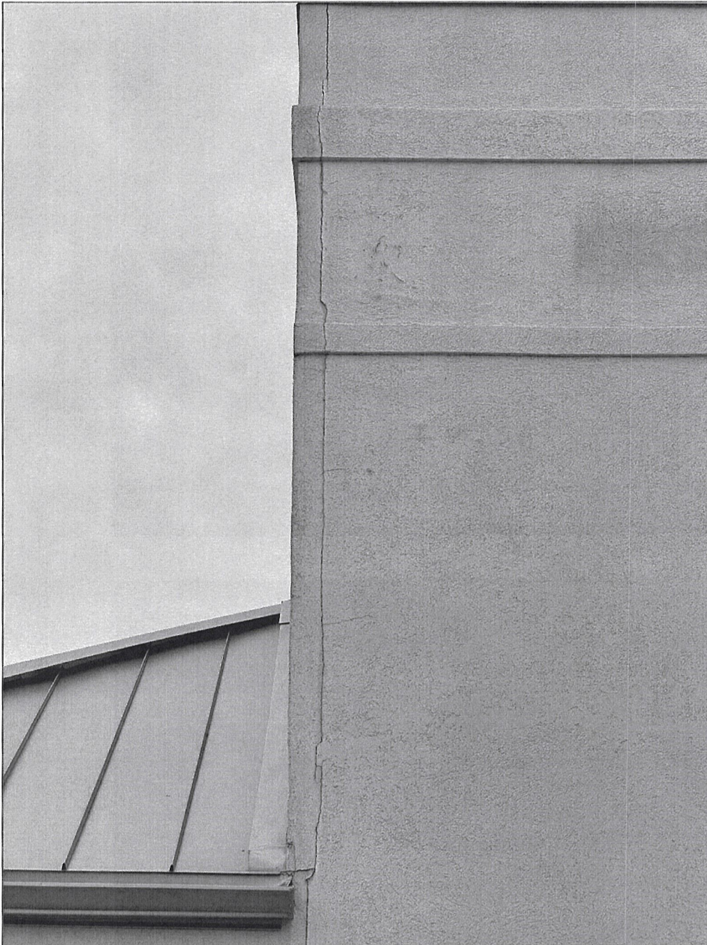
Looking east – cracking of EIFS
