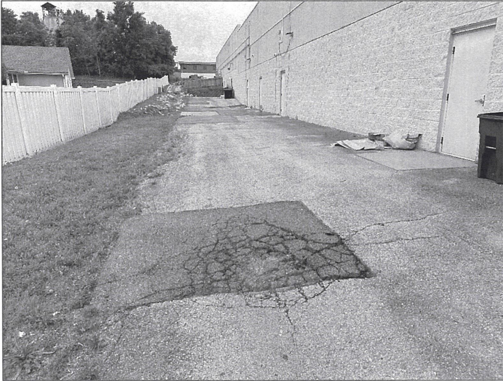
Looking south – deterioration of pavement; lack of curb/gutter; trash/debris
