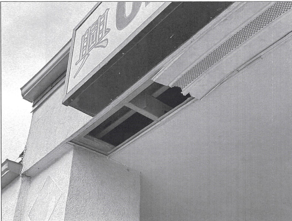
Looking east – deterioration of soffit
