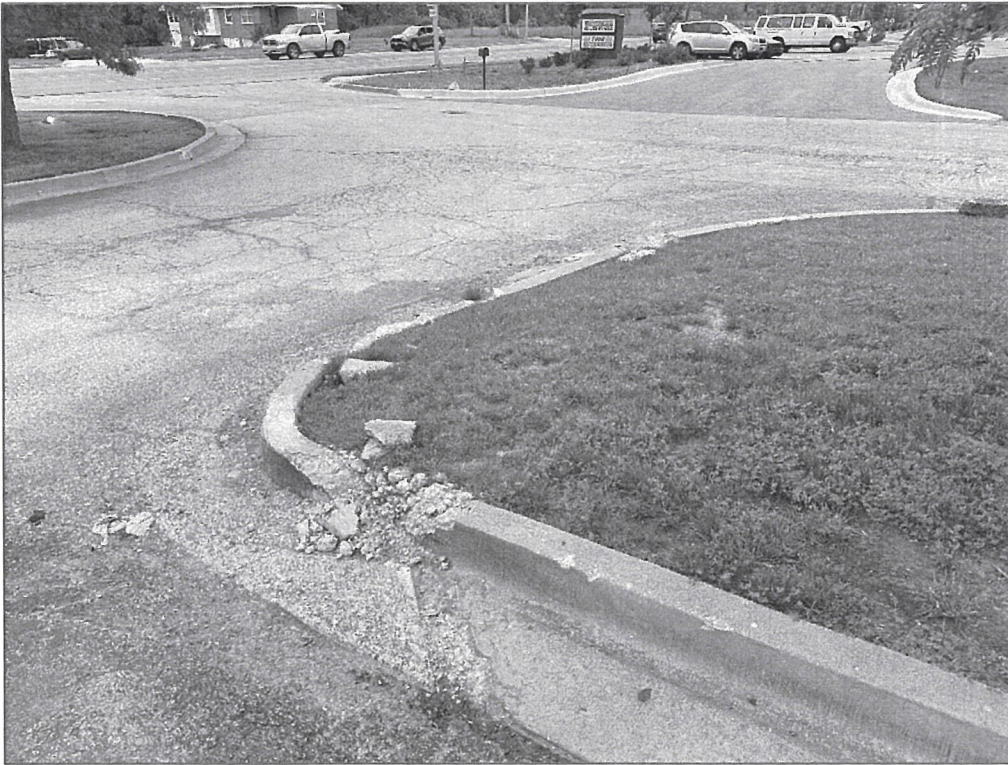
Looking northwest – deterioration of pavement and curb
