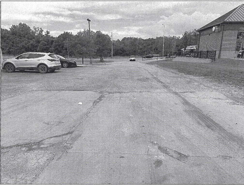
Looking west – deterioration of pavement, poor drainage (tripping/fall hazard)
