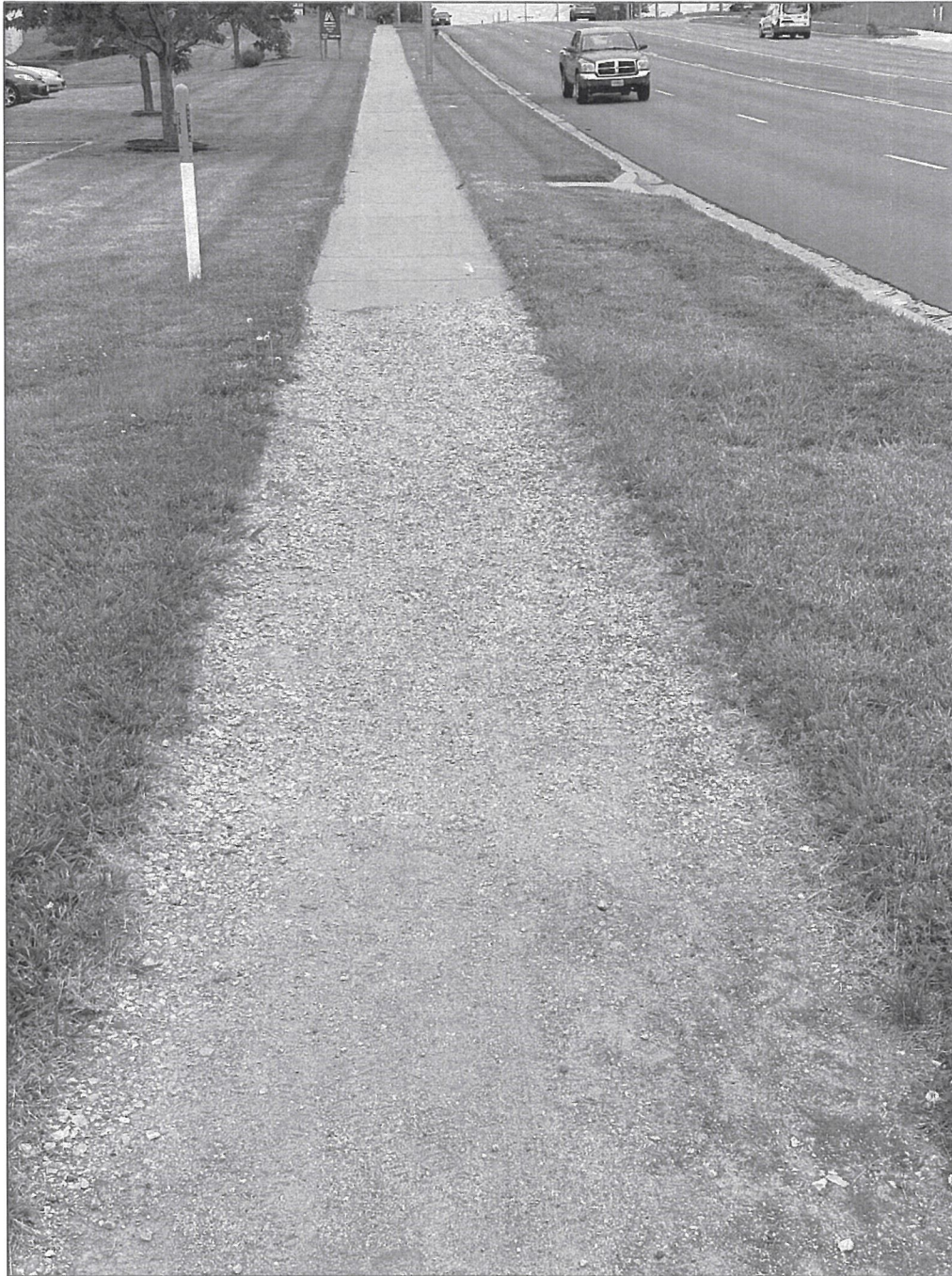
Looking south – deterioration of sidewalk (fall/trip hazard)
