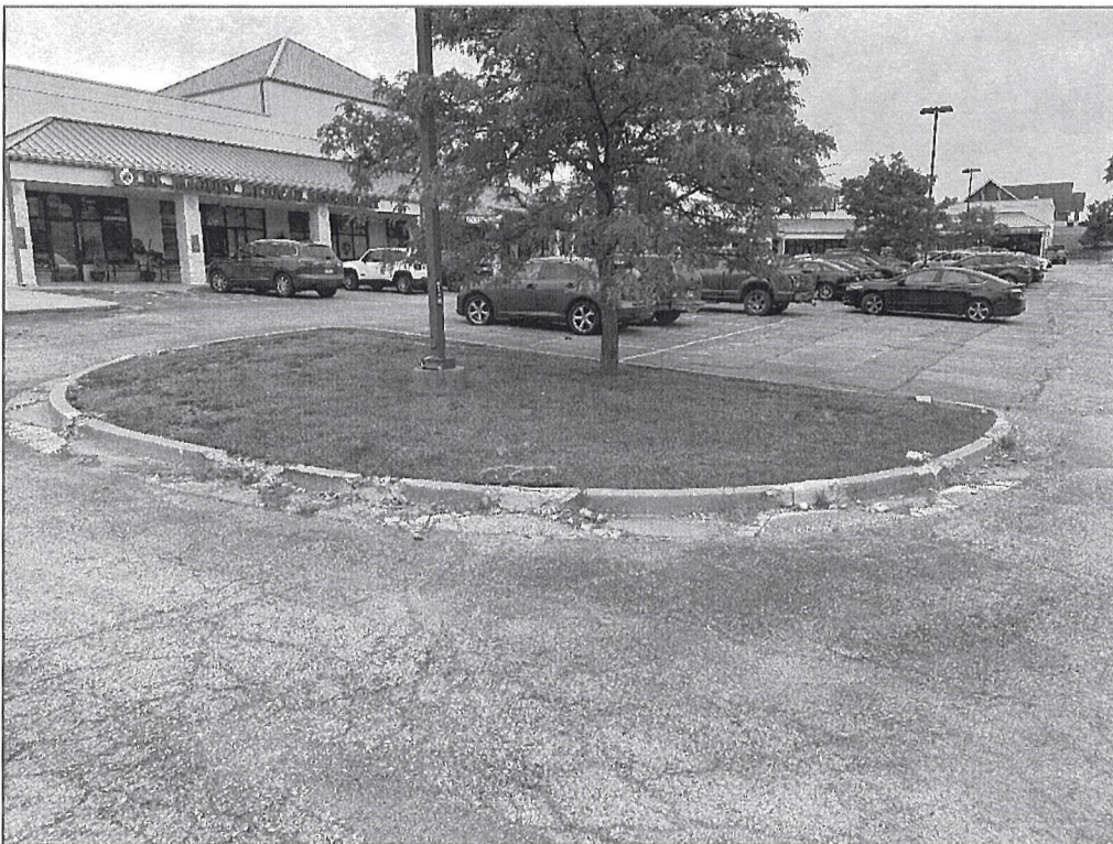
Looking southeast – deterioration of pavement and curb
