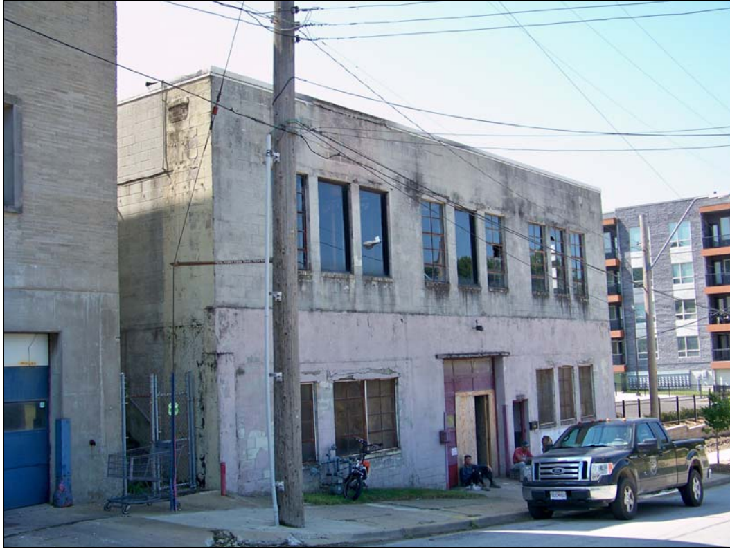
1015 E. 65 th Street – north elevation
