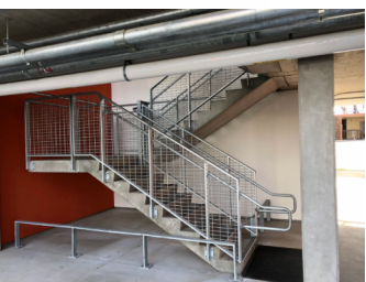
GALVANIZED STEEL GUARDRAIL WITH MESH INFILL
