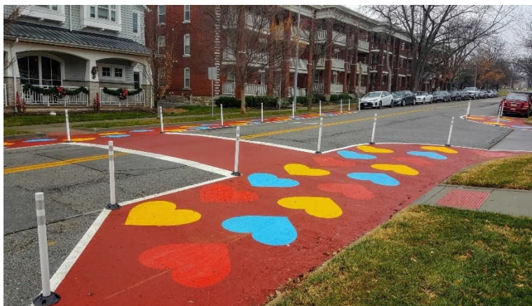
Figure 74: Neighborhood Traffic Calming on Cherry Street (Image Source: Street Smarts Design + Build)
