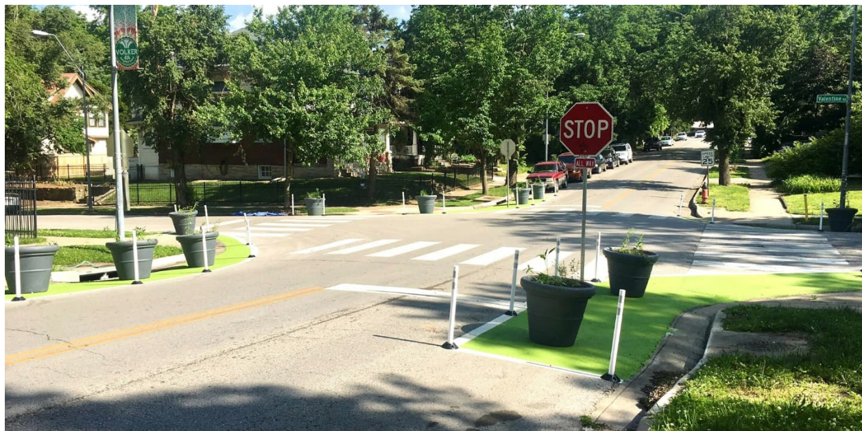
Figure 77: All way stop and traffic calming installation at Wyoming St and Valentine Rd (Image source: Street Smarts Design + Build)
