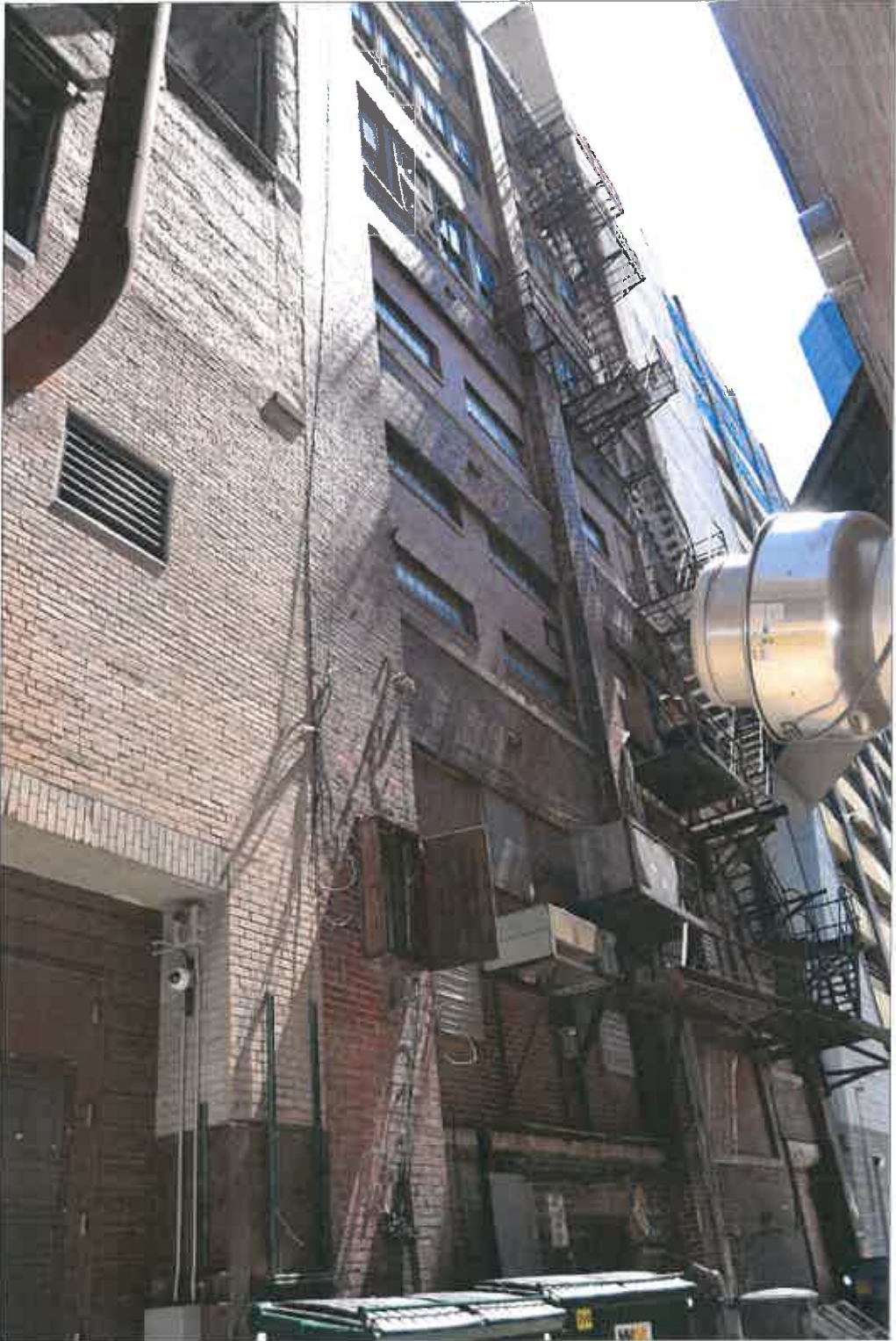
1108-1110 Grand Boulevard – West Elevation (back of building facing north/south alley)
