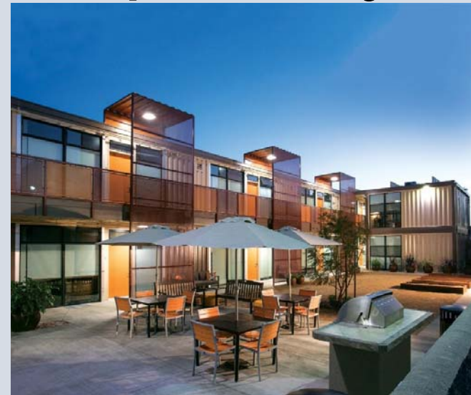
California Shipping Container Apartment Community
