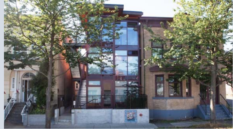
Vancouver Shipping Container Apartment Building
