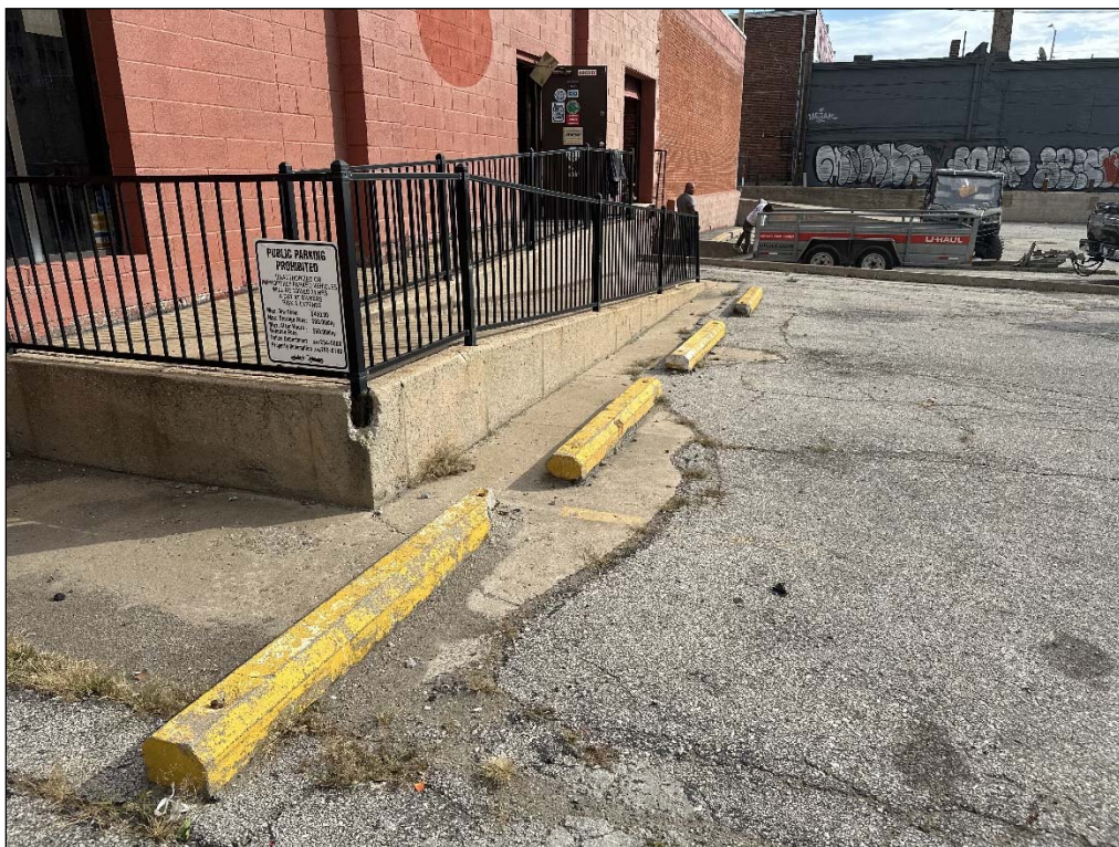
1905 Walnut Street – looking east – uneven pavement; lack of handrails for ramp; narrow ramp
