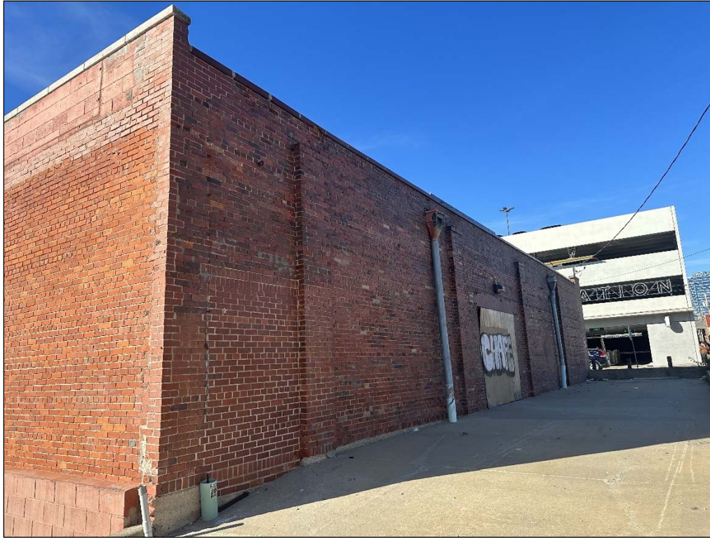
1905 Walnut Street – looking northwest at east elevation
