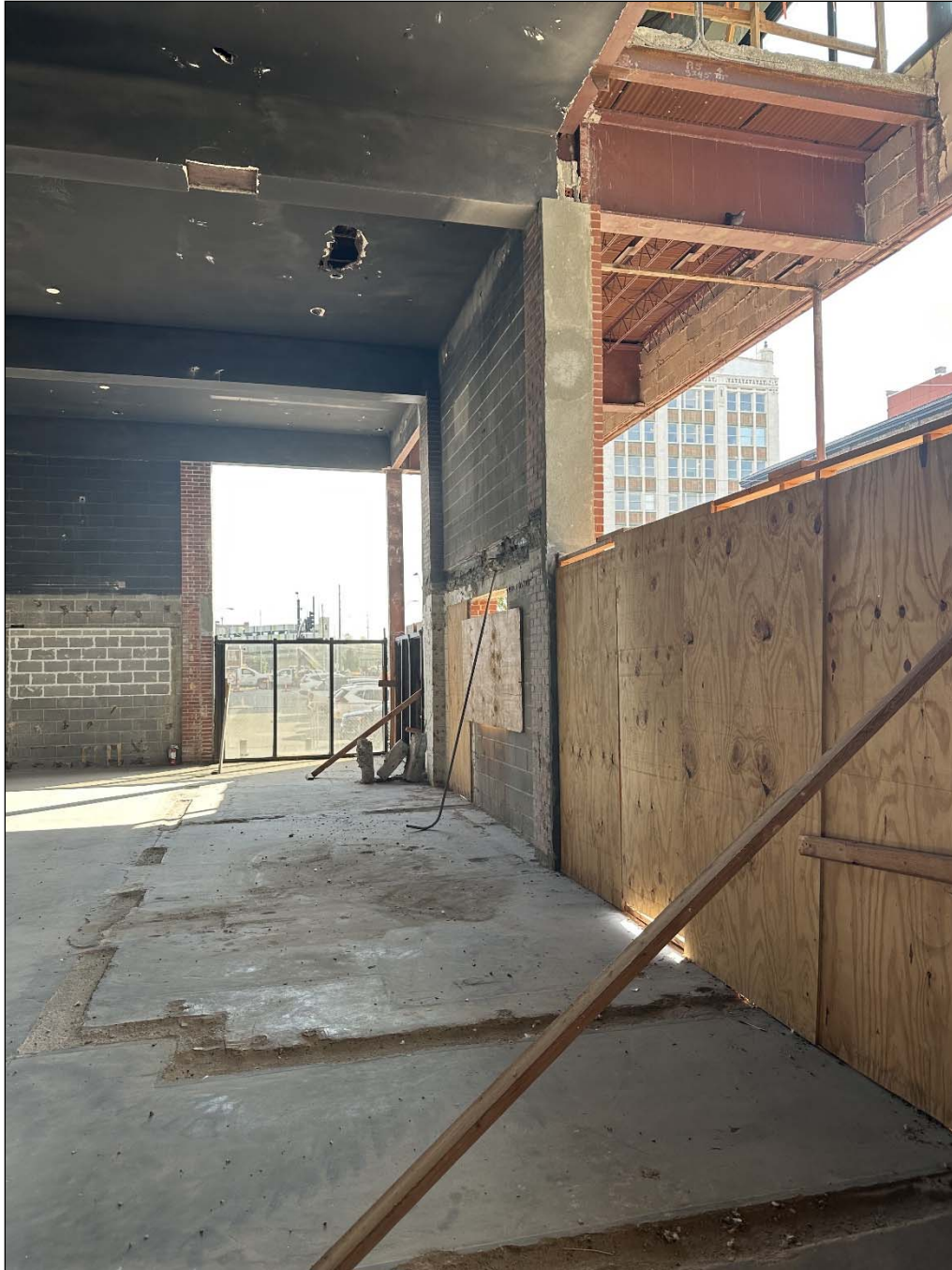
100 E. 20 th Street – interior – uneven floor; open building (lack of windows, doors)
