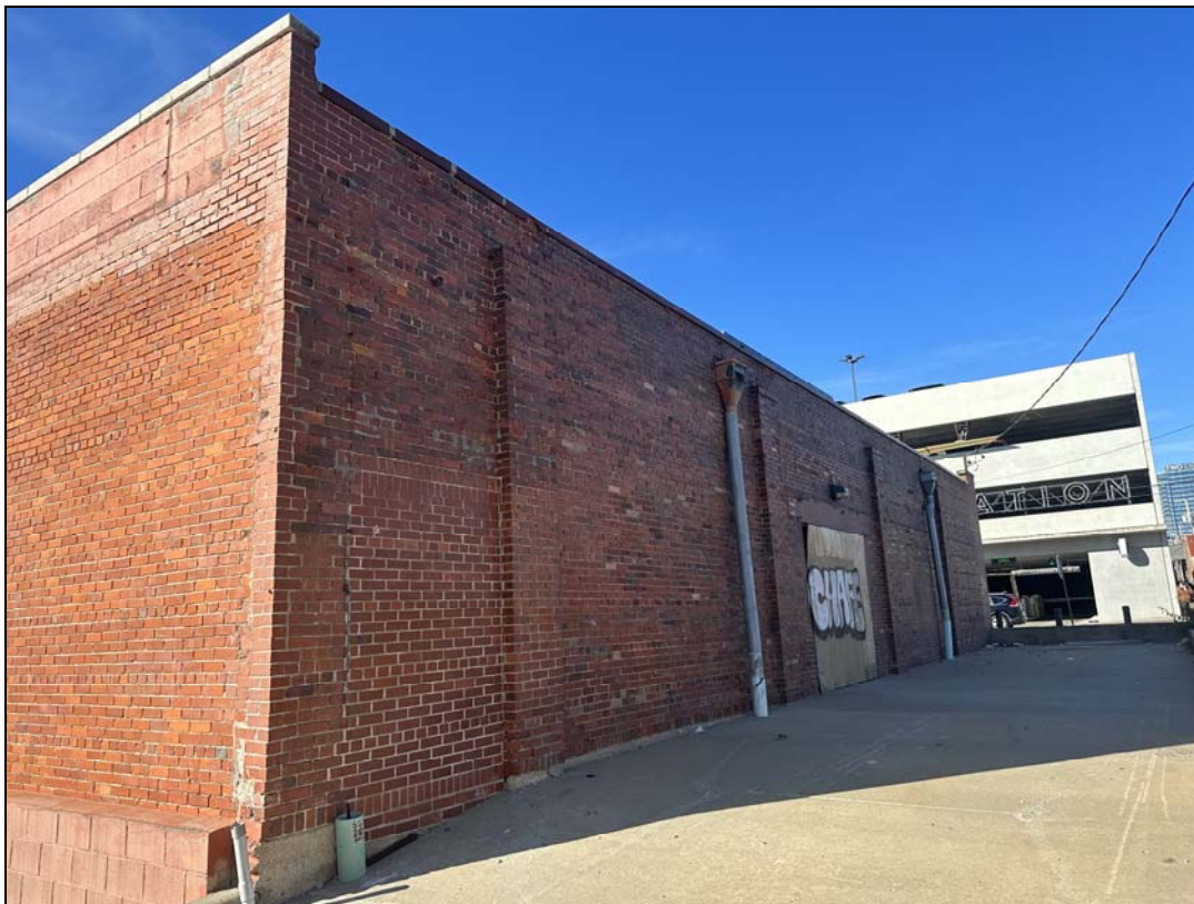
1905 Walnut Street – looking northwest at east elevation
