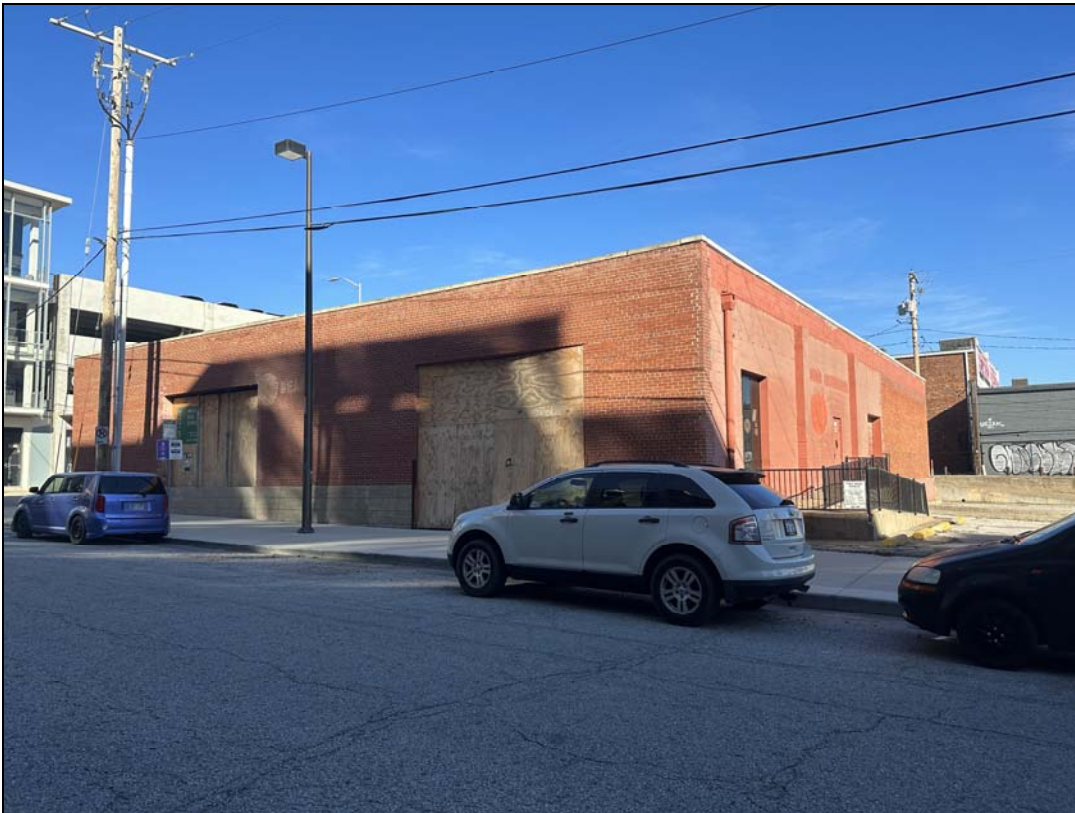
1905 Walnut Street – looking northeast at west elevation
