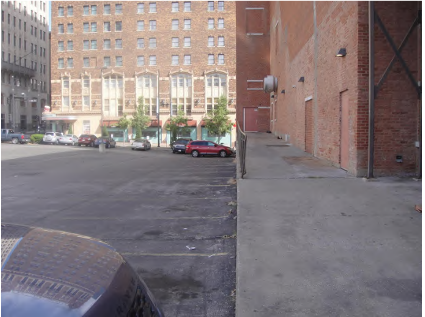
Photo 9 – Block 138. View of western location of Mainstreet Theater. New structure at this location would abut this structure.
