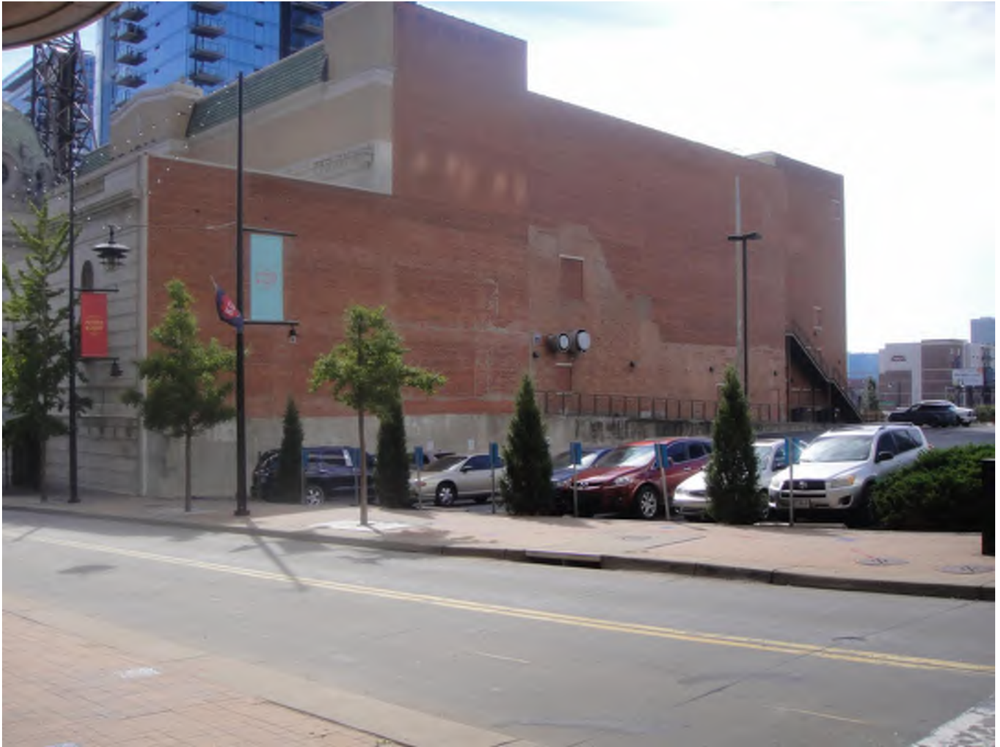
Photo 2 – Block 138. View of southwest corner of Baltimore Avenue and 14 th Street. Note B & B Mainstreet Theater to the left (not located within the Redevelopment Area).
