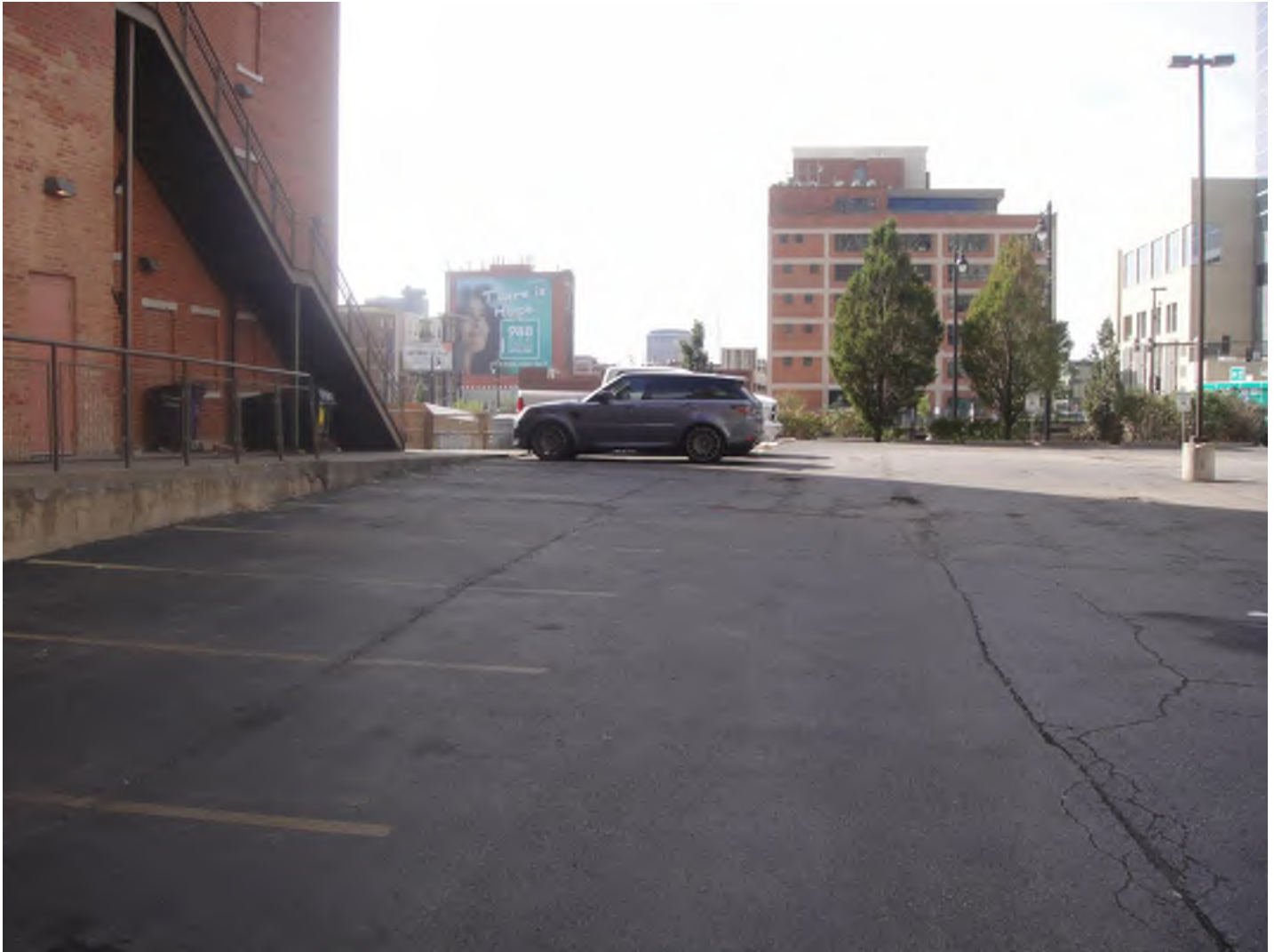
Photo 12 – Block 138. View south of eastern boundary. New structure at this location would abut the theater structure to the left.
