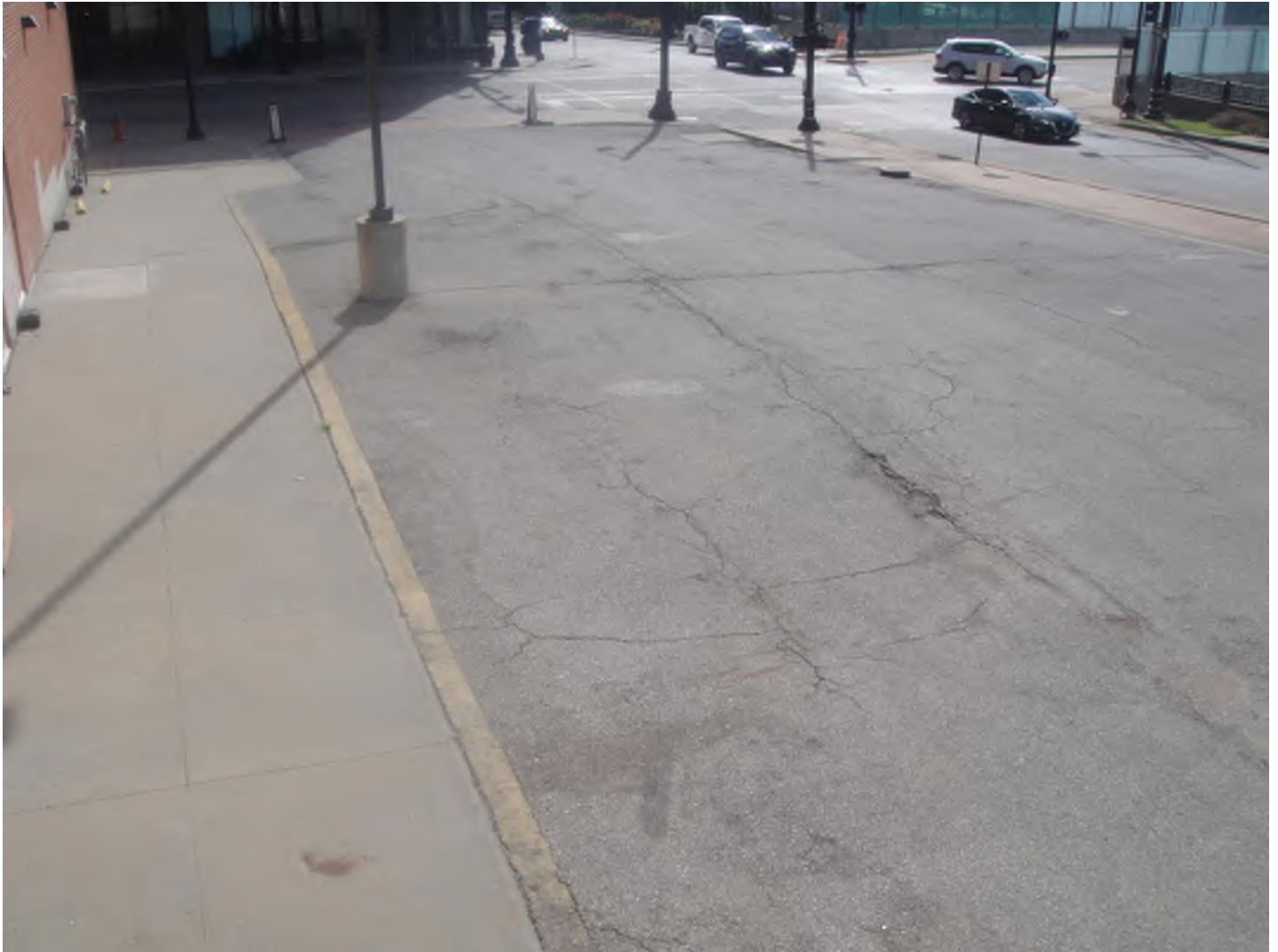
Photo 8 – Block 138. View of surface lot at the northwest corner of Main Street and Truman Road. Mainstreet Theater to the left.
