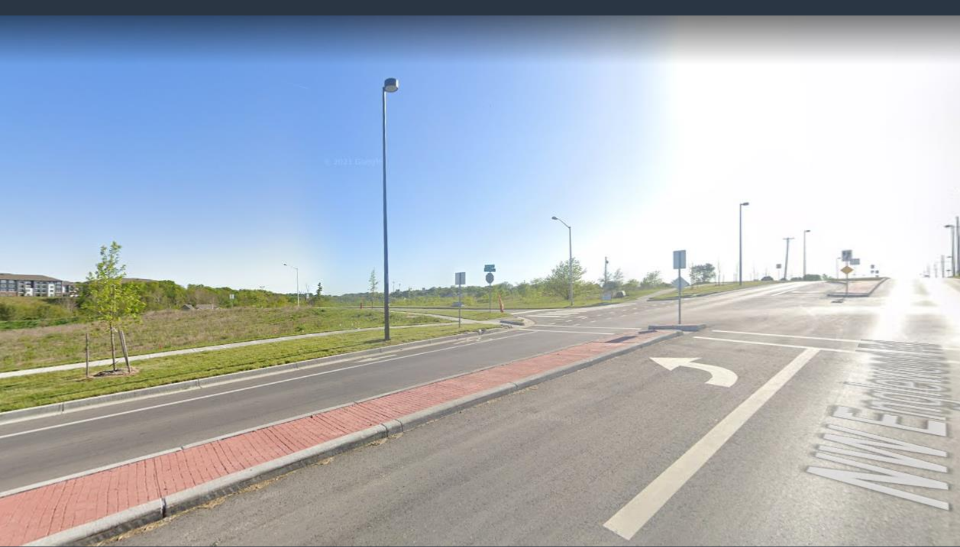
View looking southwest from NW Englewood Road
