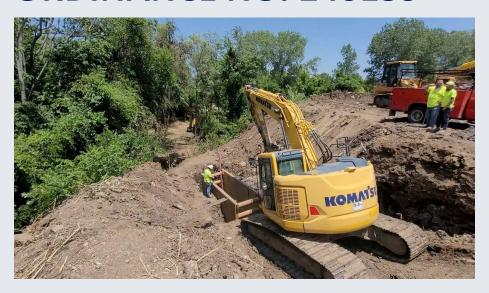
Emergency repair at 15600 E. U.S. Highway 40 due to a sewer main collapse causing an overflow to a nearby creek.
