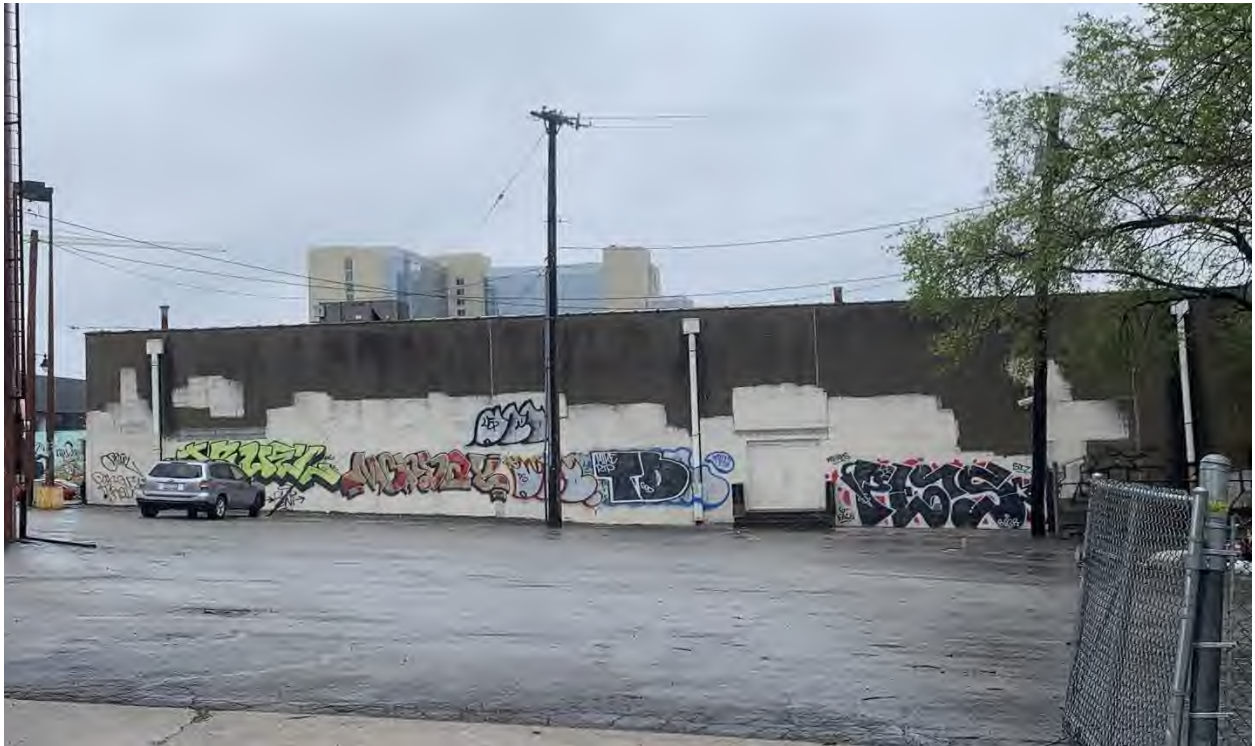
Figure 16. 1616 Broadway Blvd. Graffiti to rear of building.
