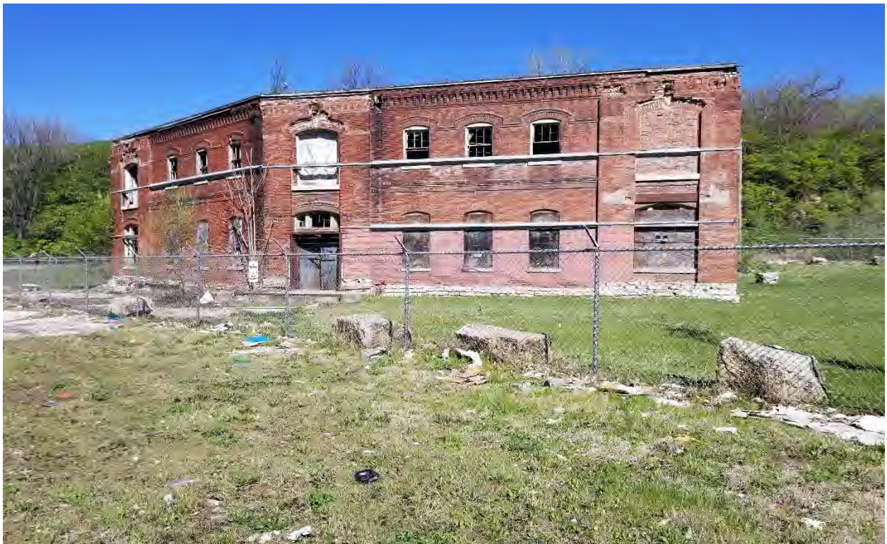
Figure 16. Imperial Brewing Building.
