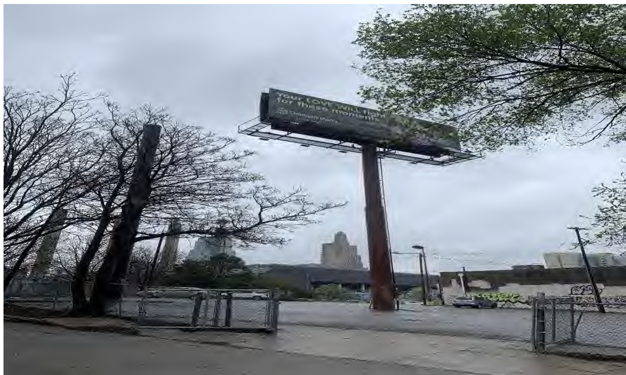
Figure 6. North end of Washington St. Billboard.
