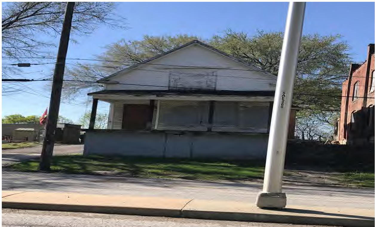
Figure 14. Vacant home on Cesar E. Chavez.
