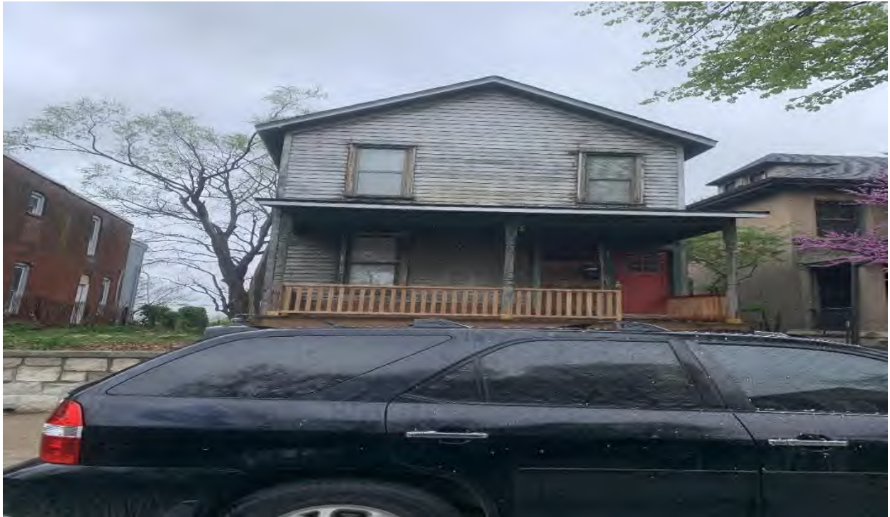
Figure 11. 1616 Madison Ave. House in disrepair.
