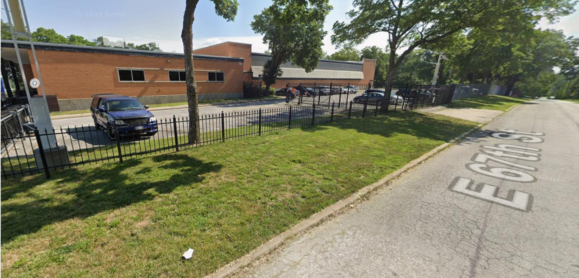
Looking towards the site from E 67 th St and Troost Ave (June 2024)
