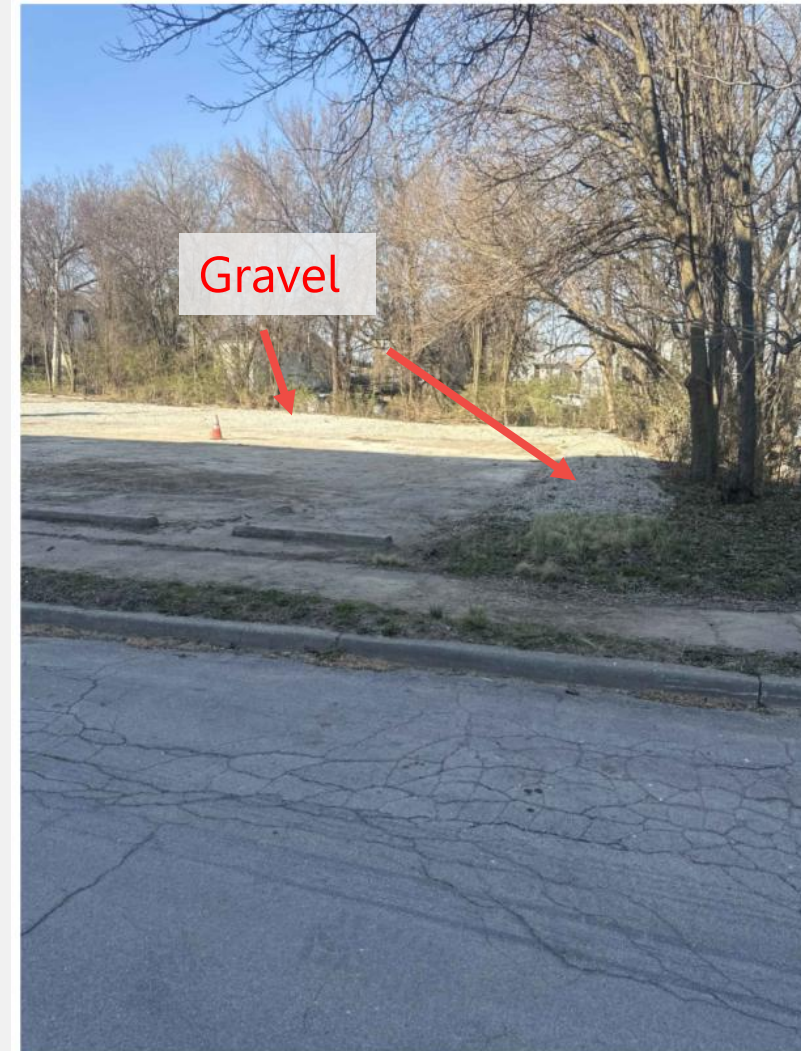
View of Northwest corner
