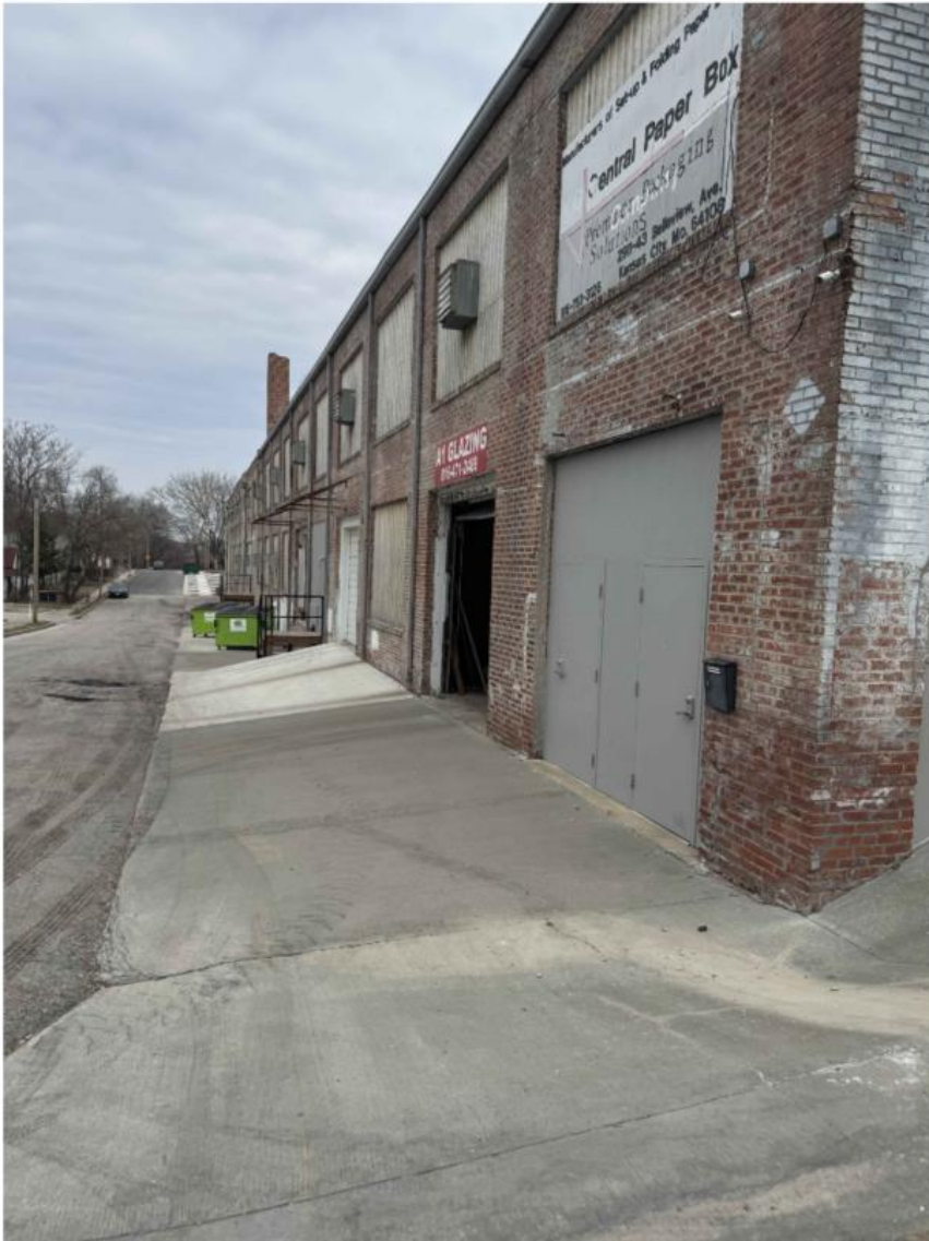
View from South looking North at building
